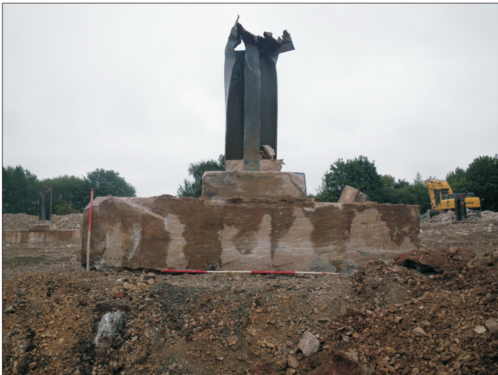
Plate 4: One of the removed stanchion bases.
