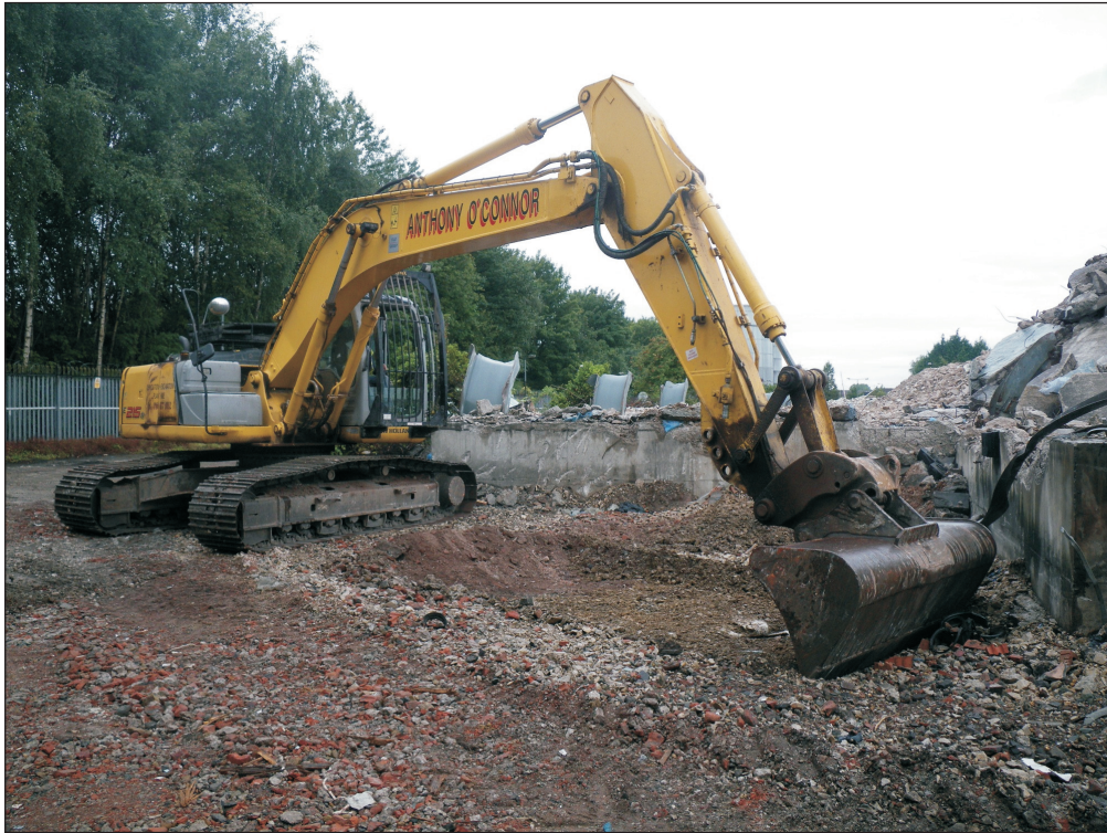
Plate 5: Pre excavation shot of Trial Trench 6.
