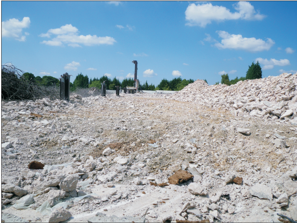
Plate 3: General shot of stanchion bases, pre excavation.
