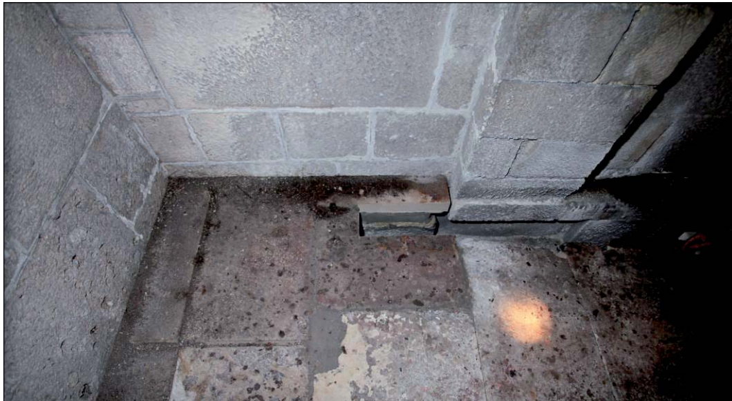
Plate 25: Evidence of re-flooring within portcullis chamber
