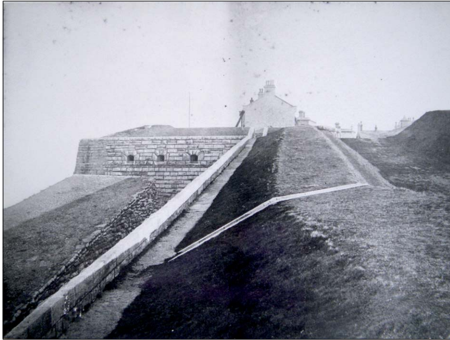
Plate 7: Royal Corps of Engineers photo dated 1877 looking north along main entrance road showing rock cut walls to entrance road
