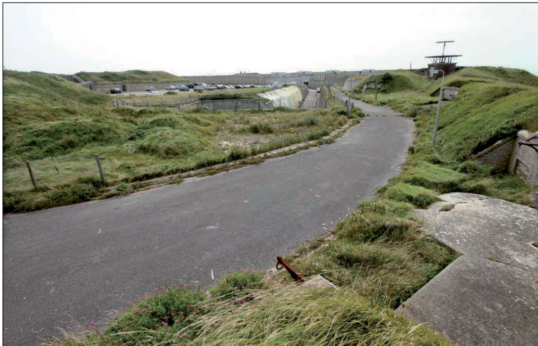
Plate 16: General area directly over main tunnel entrance viewed from north-east
