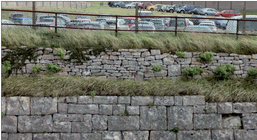
Plate 14: Detail of 'dry-stone' wall construction material and style viewed from west
