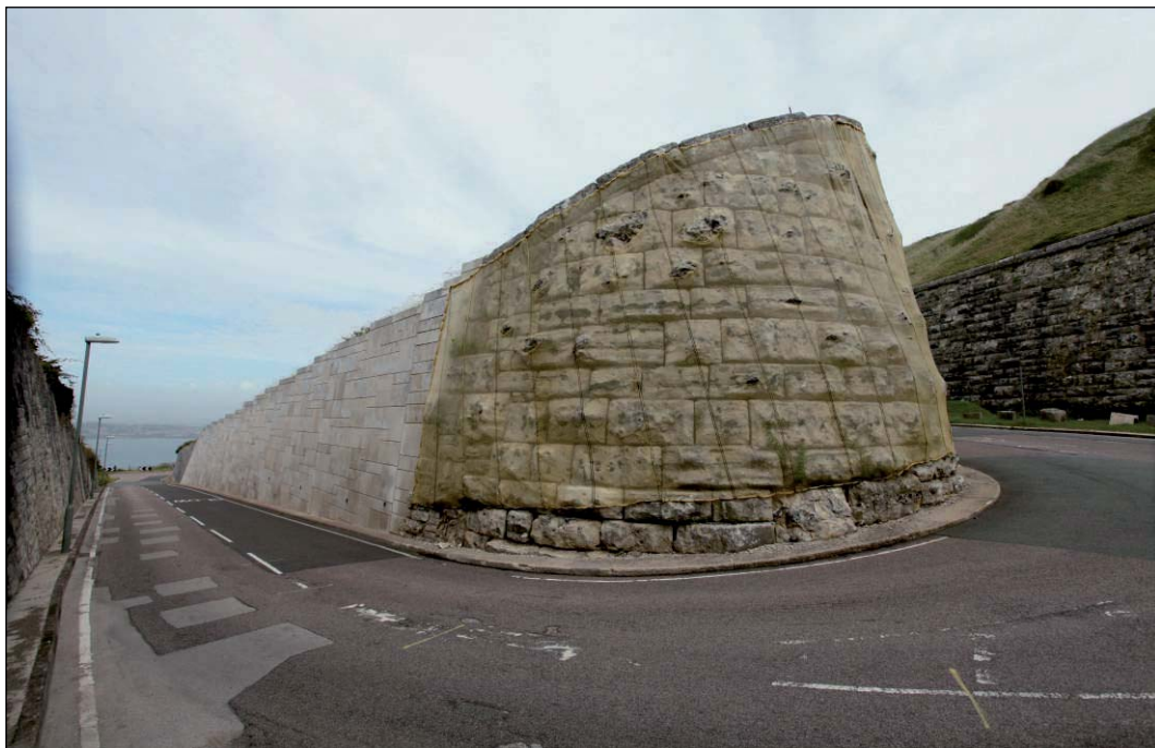
Plate 32: Roadside walling stone-faced and covered with protective netting
