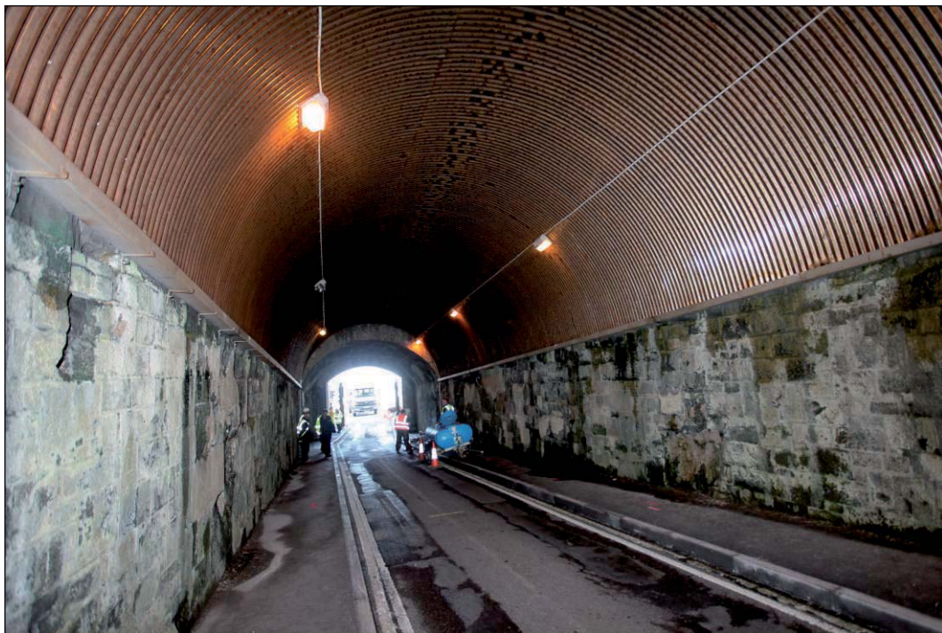
Plate 26: Main tunnel entrance roof lining viewed from south
