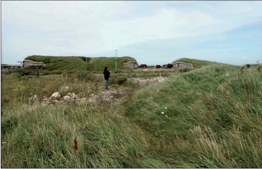
Plate 21: Area directly above south tunnel entrance viewed from east
