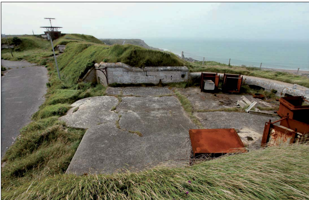
Plate 18: Overlooking 12.5 inch gun emplacement showing concrete apron and present condition viewed from north
