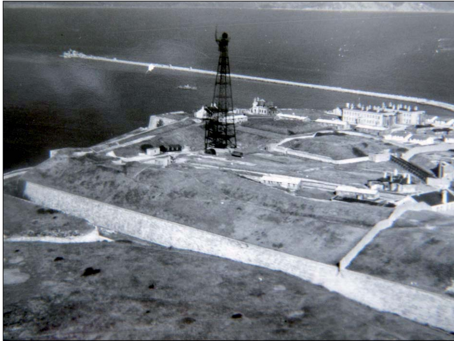
Plate 11: Military oblique aerial photo dated 1950 showing 'dry-stone' wall
