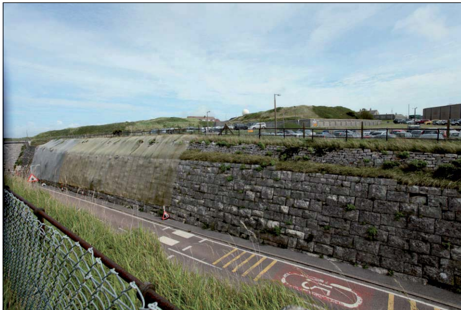
Plate 12: View along east revetting wall of access road showing 'dry-stone' wall above main wall viewed from south-west
