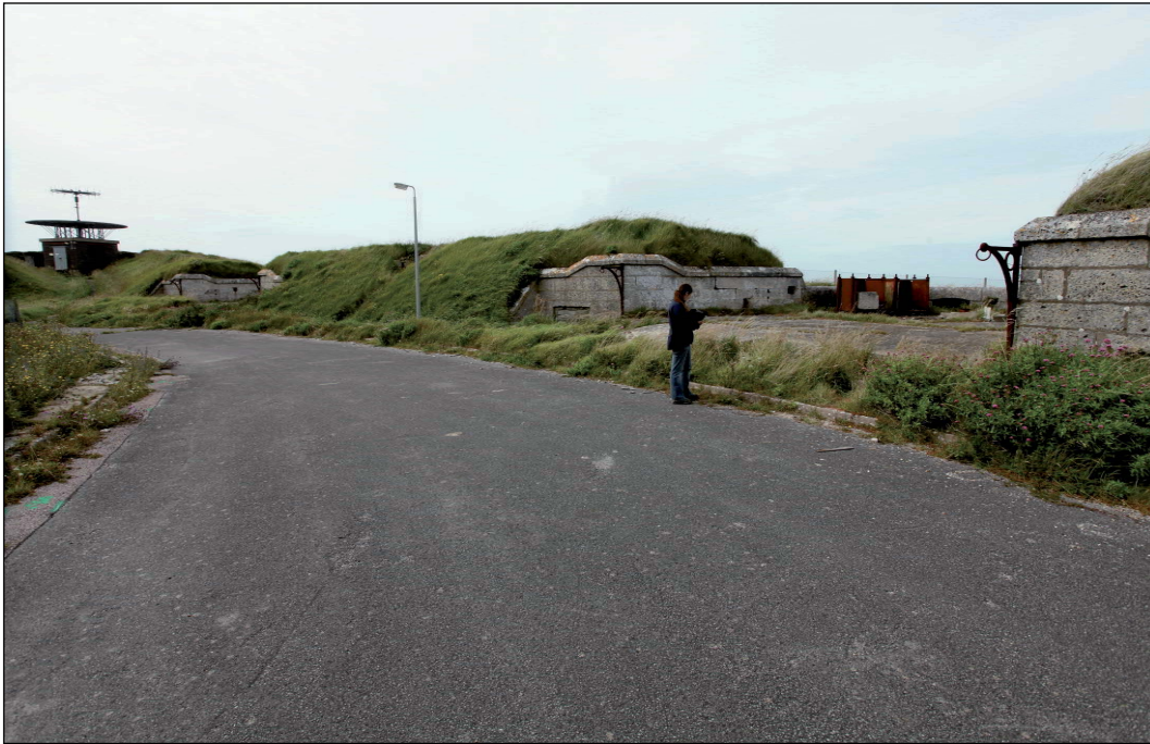
Plate 17: Ground level aspect of 12.5 inch gun emplacement and service road viewed from north-east
