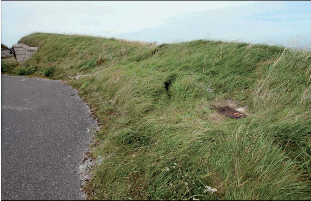
Plate 19: North embankment above main entrance viewed from east
