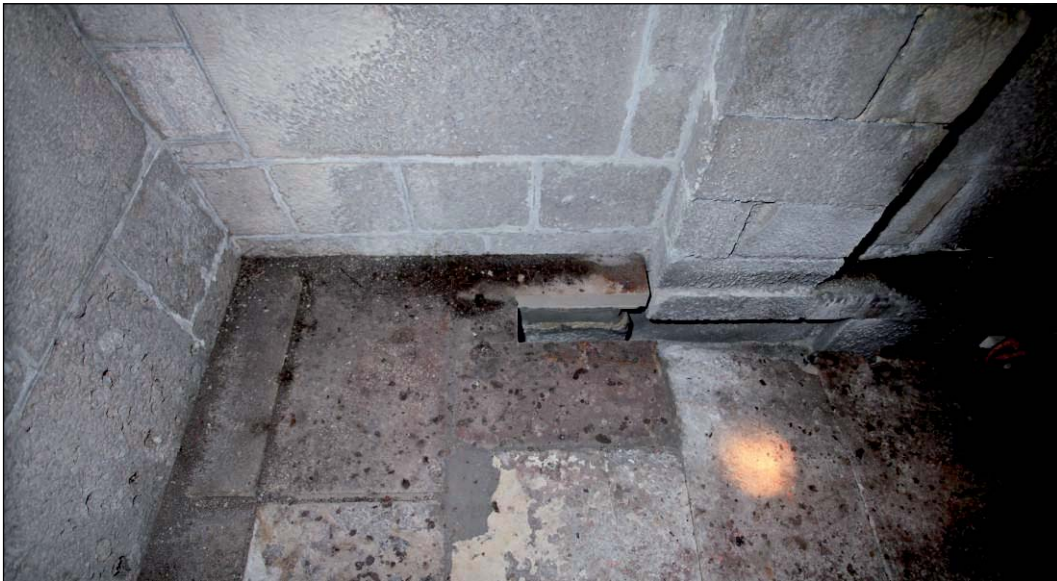
Plate 25: Evidence of re-flooring within portcullis chamber
