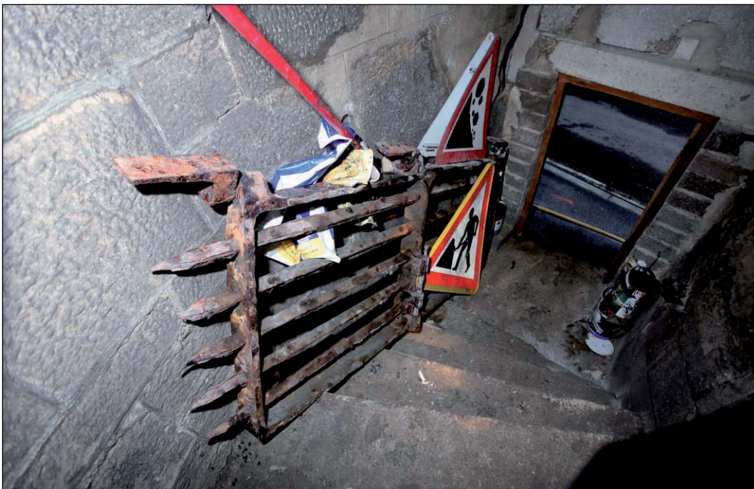
Plate 28: East portcullis chamber access gate removed and placed against internal wall
