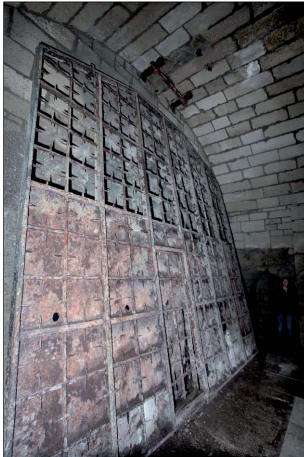
Plate 22: Detail of portcullis
