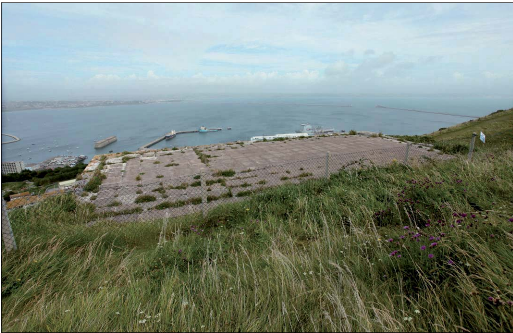
Plate 20: Top of main entrance 'terrace' viewed from south
