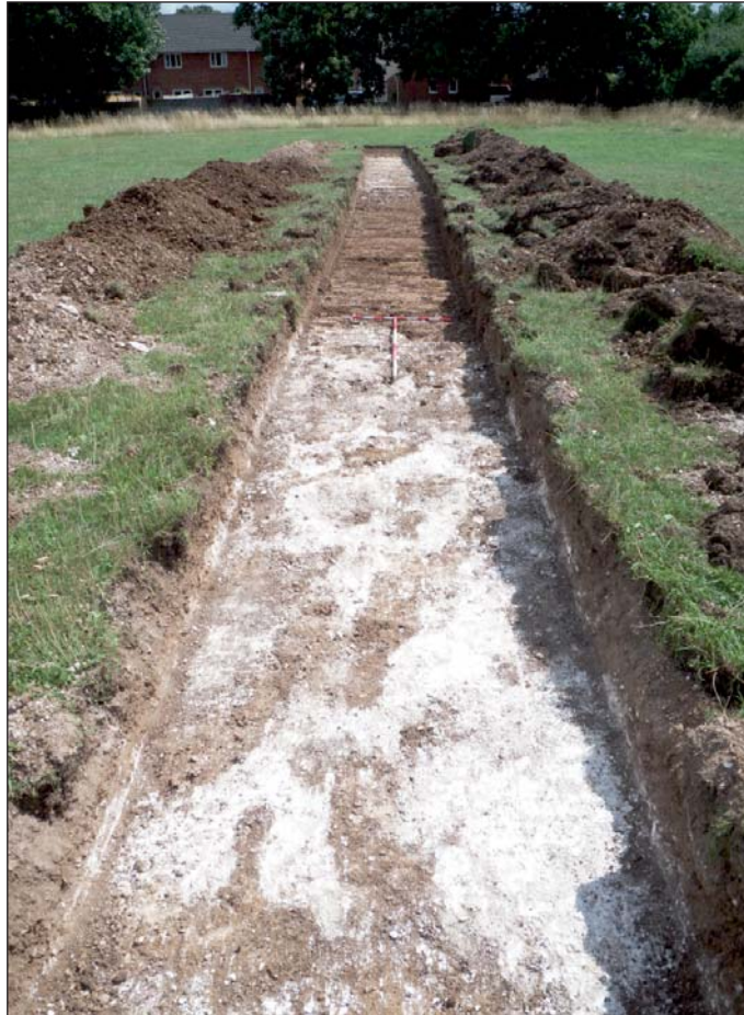
Plate 1: Trench 14, viewed from the south-west.
