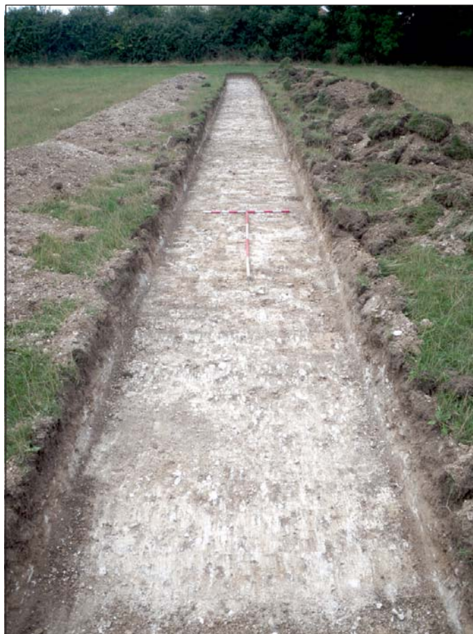
Plate 4: Trench 13, viewed from the north-east
