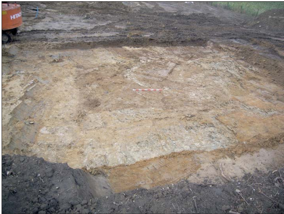
Plate 1: Made ground deposit following topsoil removal
