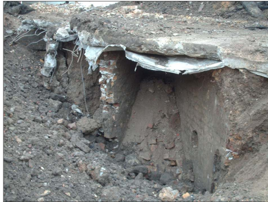
Plate 8: Walls 109 & 110, view looking south-east
