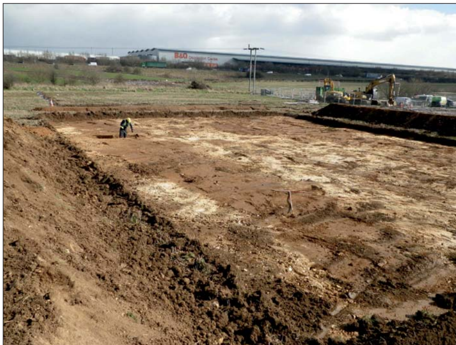
Plate 4: Mitigation Area 4, two large solution channels
