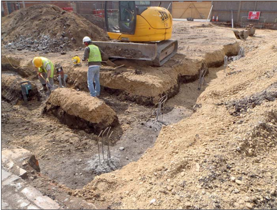
Plate 1: General view of excavated ground beam trenches
