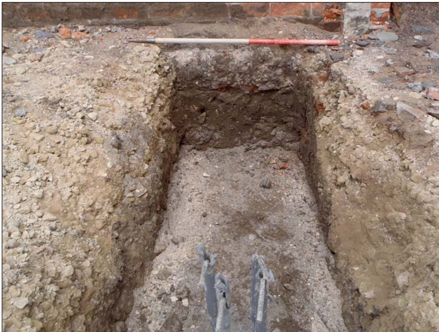
Plate 2: Stratigraphy in ground beam trench
