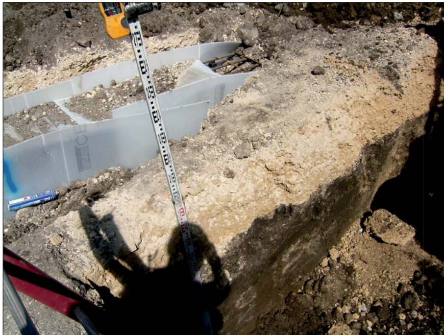
Plate 4: Excavated lift pit trench
