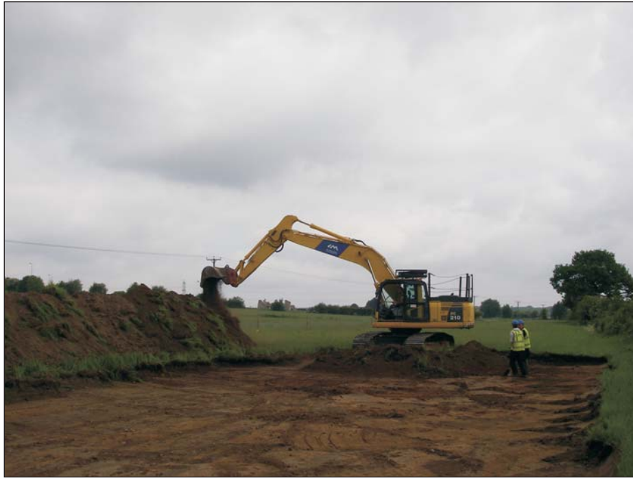
Plate 1: Topsoil stripping in Field 2, noting St. John's Palace in background, looking north.
