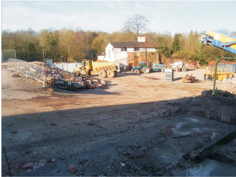
Plate 1: General view across Bath Vale Mill from north-east
