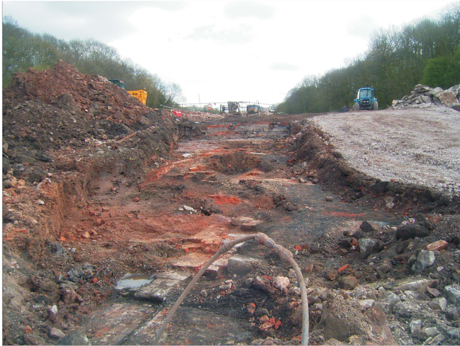
Plate 11: General view of Area 3 from the north-west showing structures associated with a former engine and boiler house.
