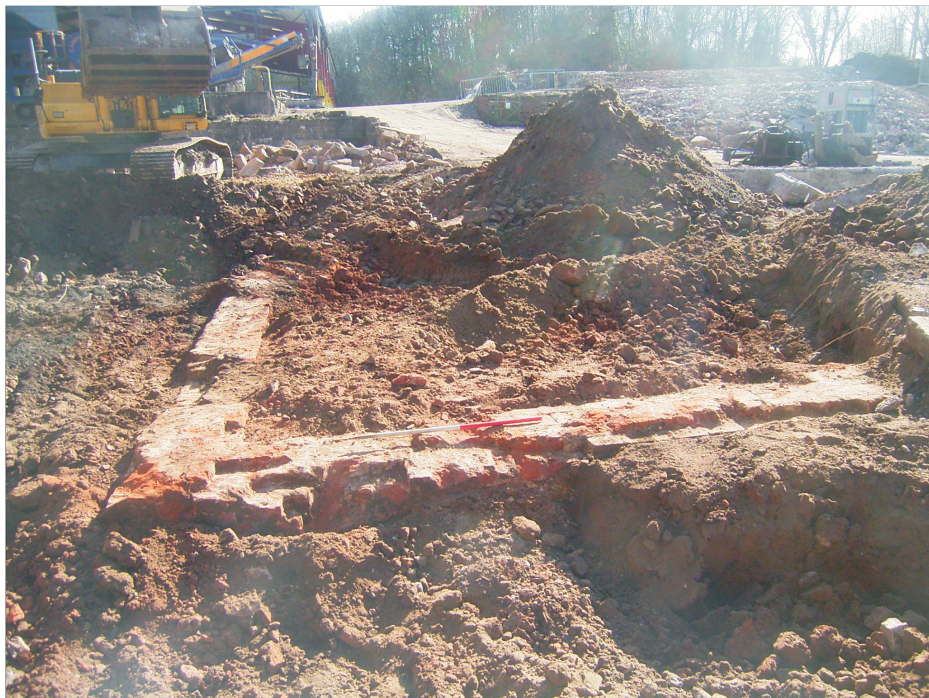
Plate 2: Exposed remnant of mill building 115 from the north-west
