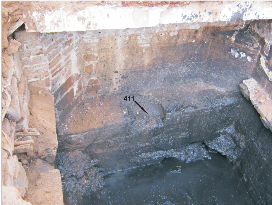
Plate 17: Detail of axle mount 411 for water wheel in northeast wall of 403 . Viewed from the south.
