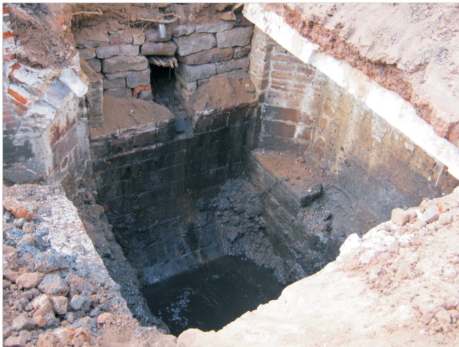
Plate 16: General view of wheel pit structure 403 in Area 4 from the east
