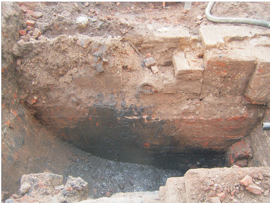
Plate 6: Detail of north-east facing elevation of 110
