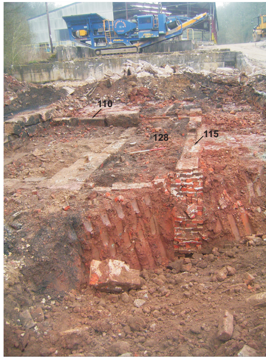
Plate 3: General view (from the north-west) showing space 128 between mill 115 and wheel pit 110 structures
