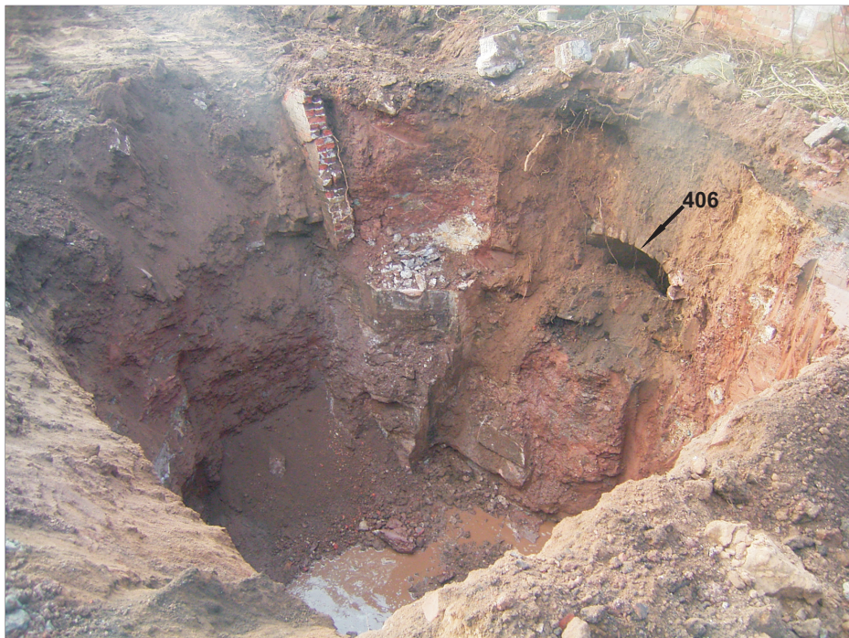
Plate 18: General view of Area 4 during remediation showing Head Race 406 from the north.
