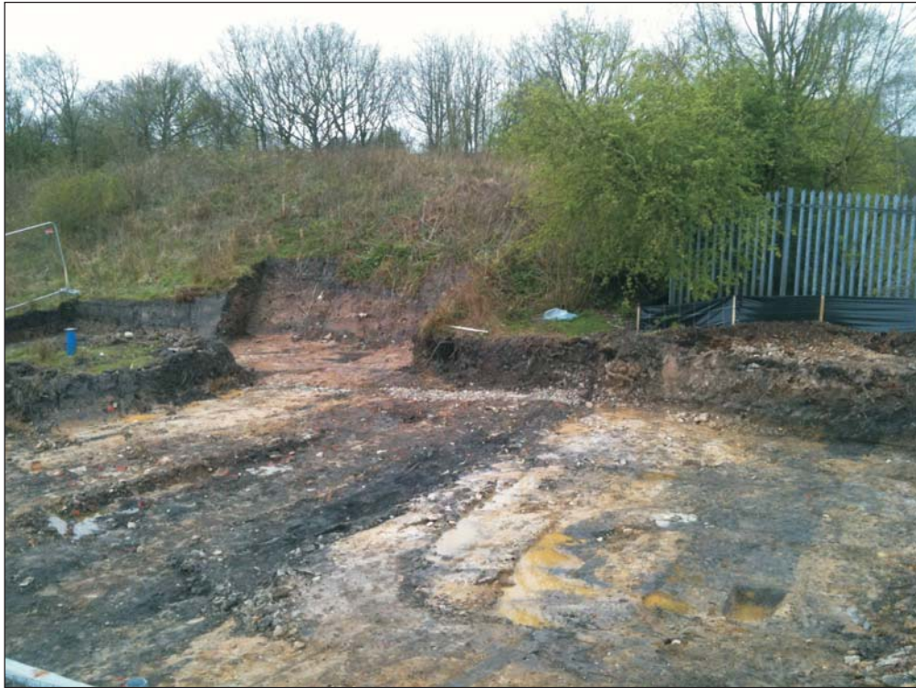
Plate 1: Trench 1, general shot following excavation, looking south west.
