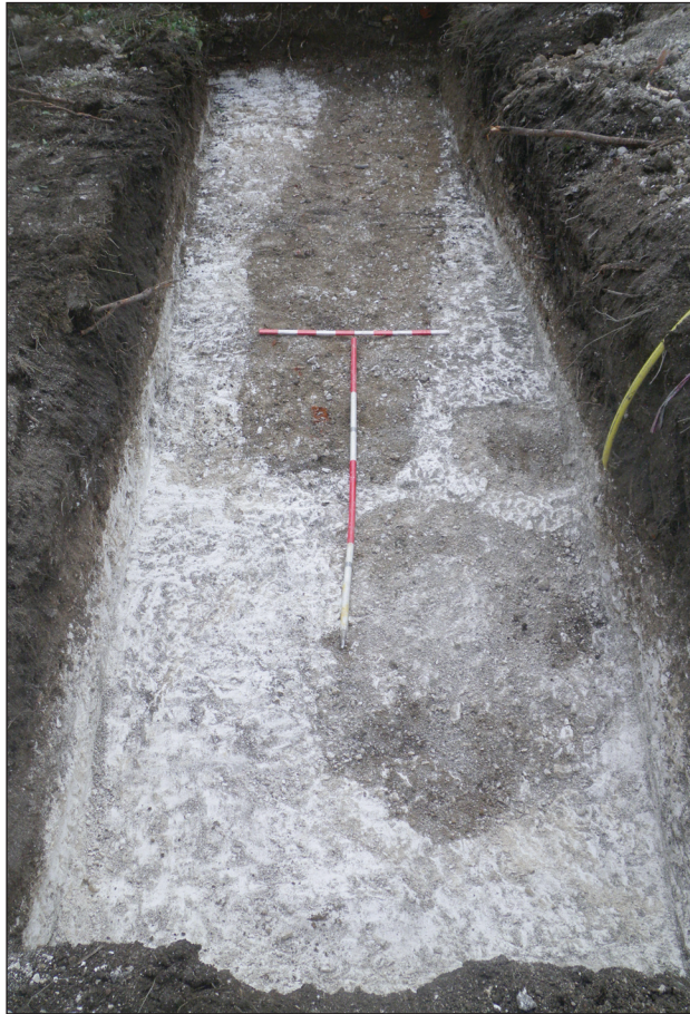
Plate 5: Trench 3, viewed from the north
