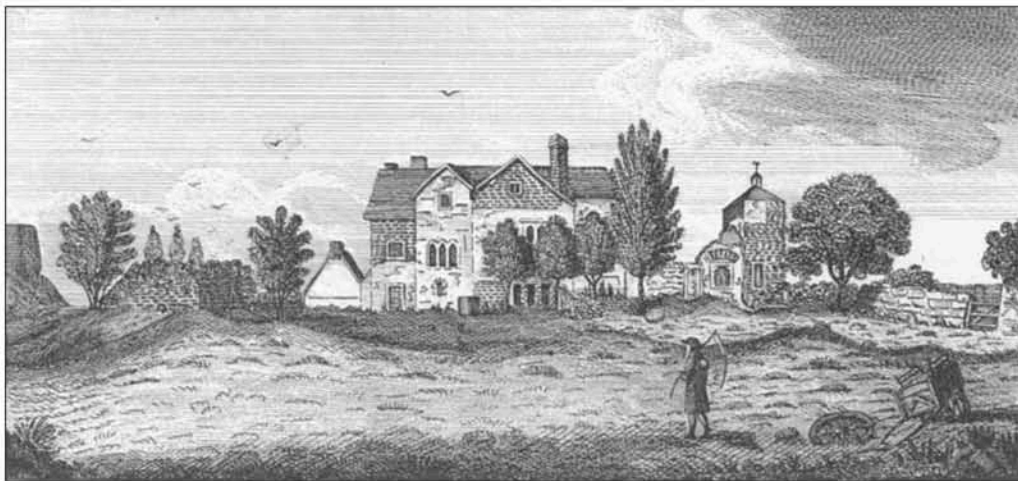
Plate 2: View of Groby Old Hall from the north-west, dated 1790 (from Nichols 1811, 634, plate 104)
