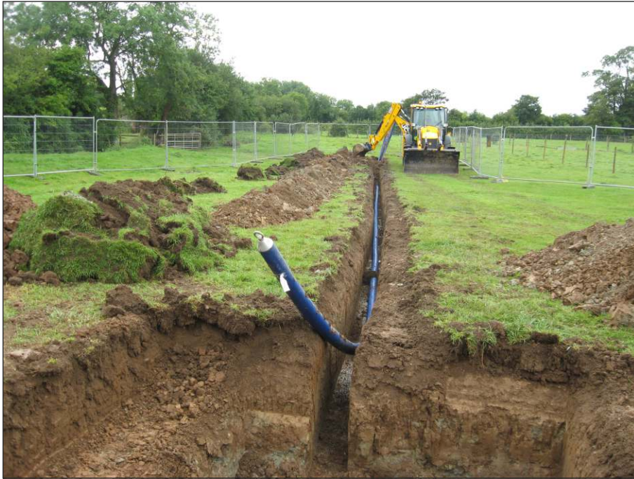
Plate 1: Laying the pipe
