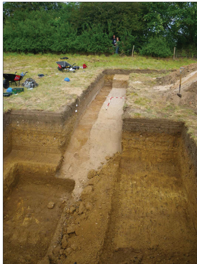
Plate 7: Trench 2 in mid-excitation, view from west
