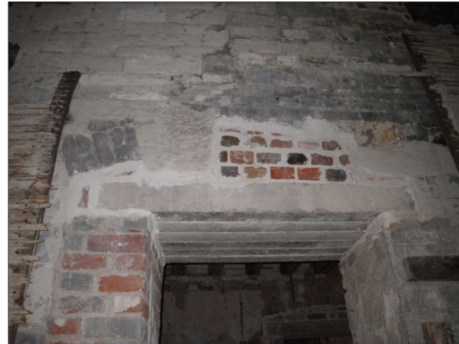
Plate 2: Reuse of remnants of voussoir windows from original stables
