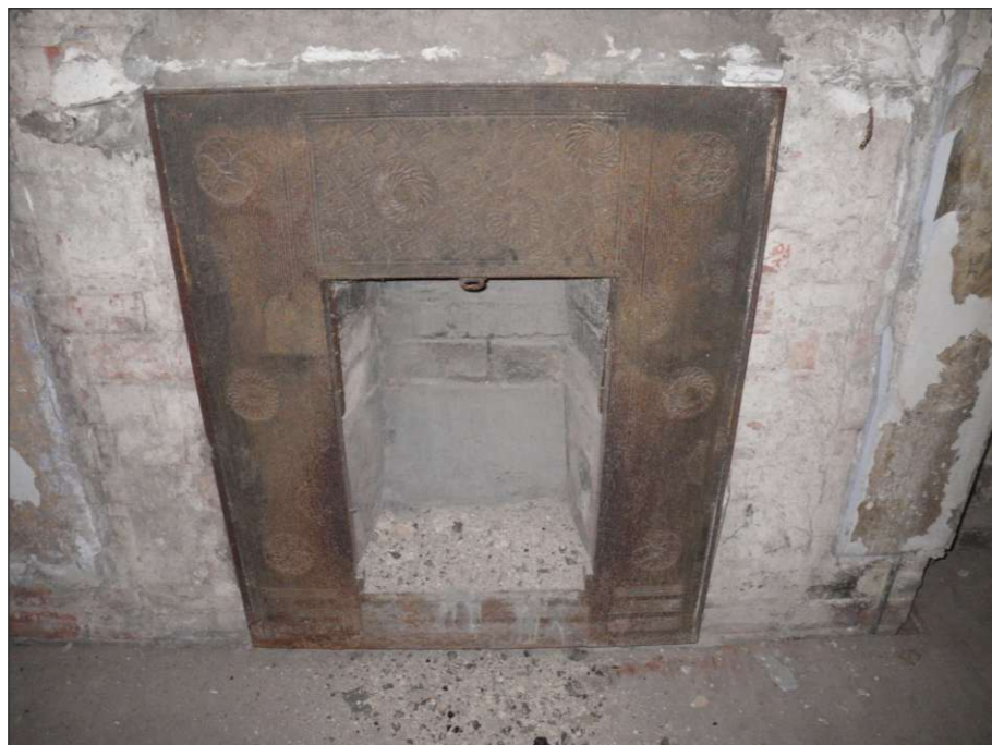
Plate 3: Thomas Jekyll design fireplace c. 1870, in Trainer's House
