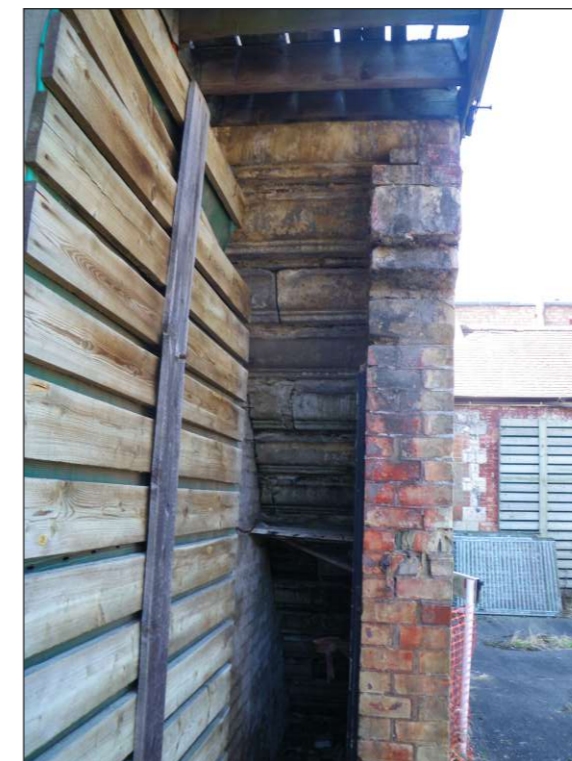
Plate 4: Moulded stone pieces reused within staircase on outside of later stable block
