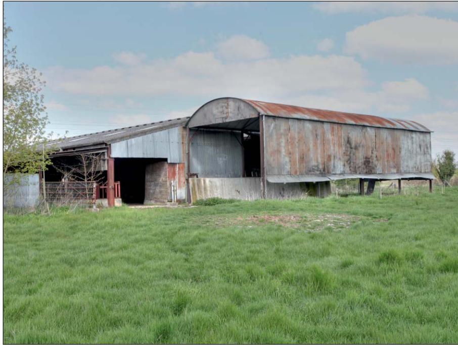
Plate 5: North-south orientated barn and raised dry store
