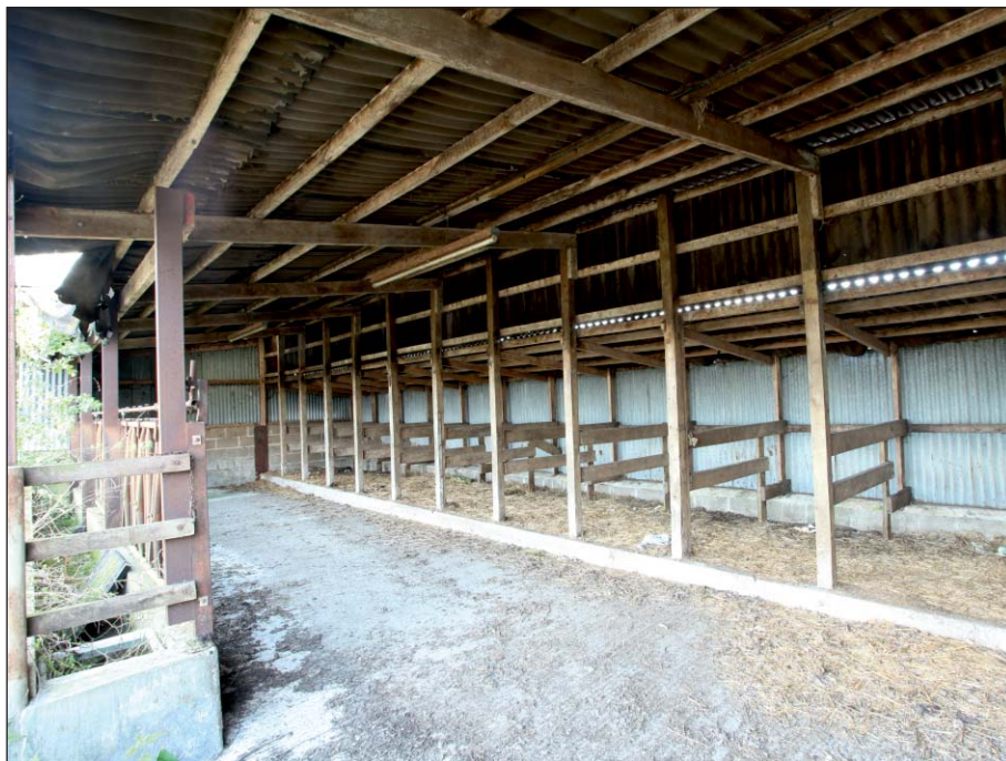
Plate 6: East-west orientated outbuilding interior
