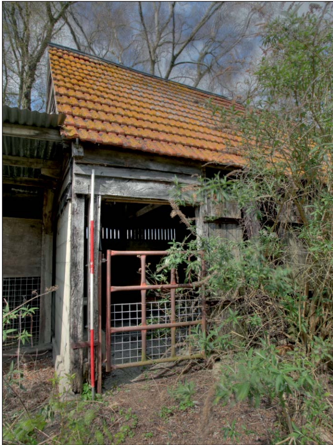
Plate 23: Eastern study building, west end: south-west corner entrance
