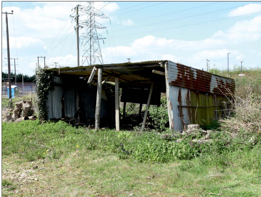
Plate 7: Corrugated iron lean-to
