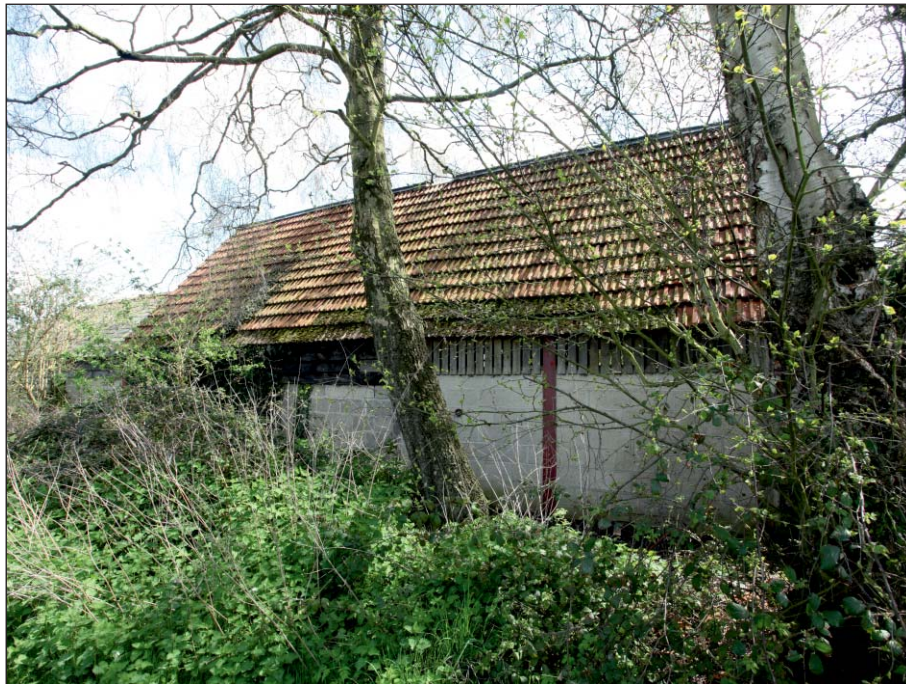
Plate 21: Eastern study building, west end: north elevation
