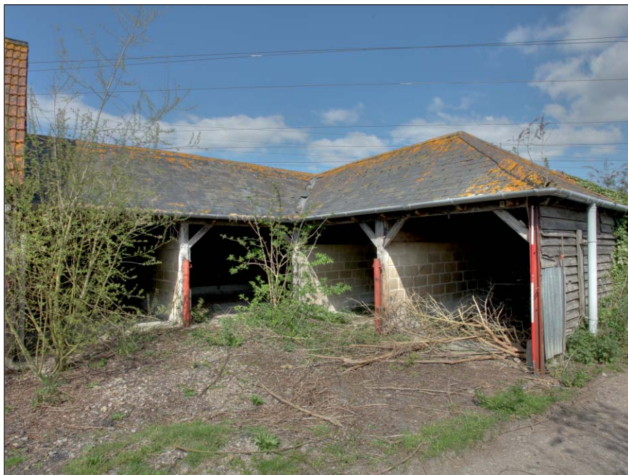
Plate 16: Eastern study building, east end: south and west elevations
