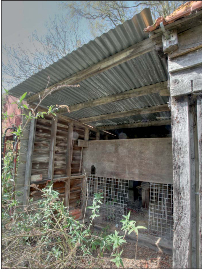
Plate 27: Eastern study building, west end: south-west corner entrance
