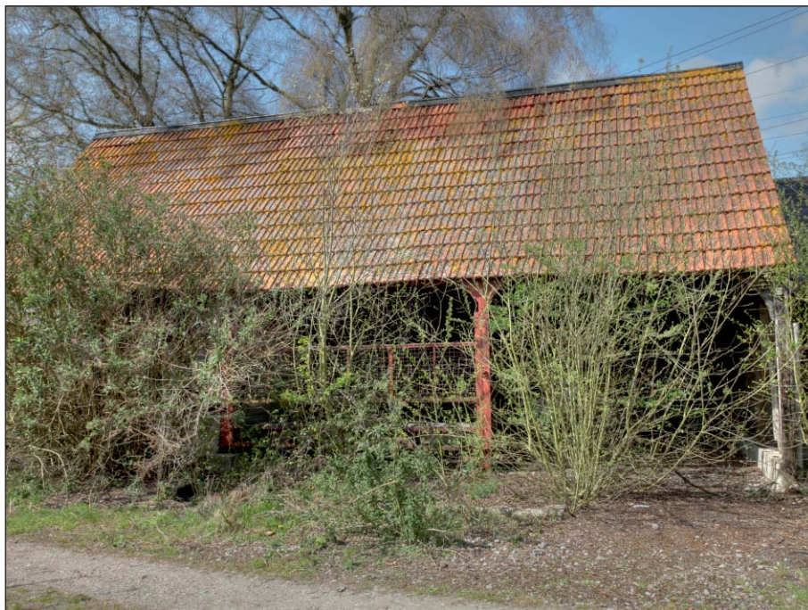
Plate 22: Eastern study building, west end: south elevation
