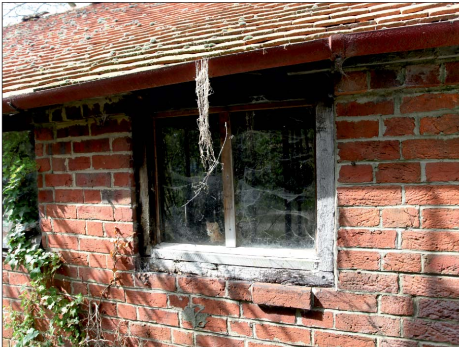
Plate 14: Western study building: typical 2-light window
