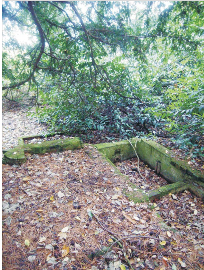
Plate 7: Spillway or pond overflow
