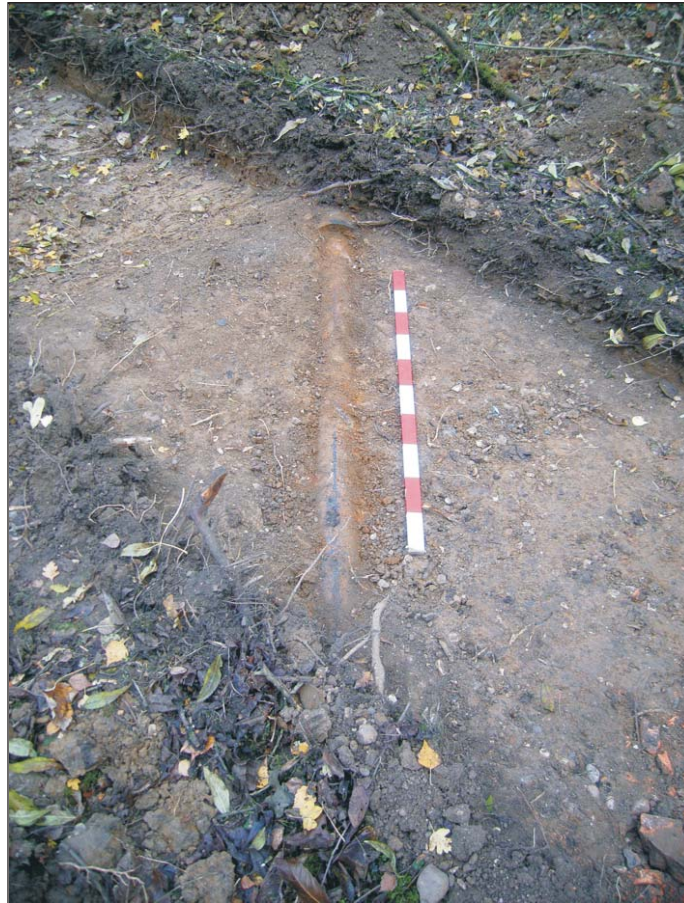
Plate 19: Trench 2 cast iron water main 204
