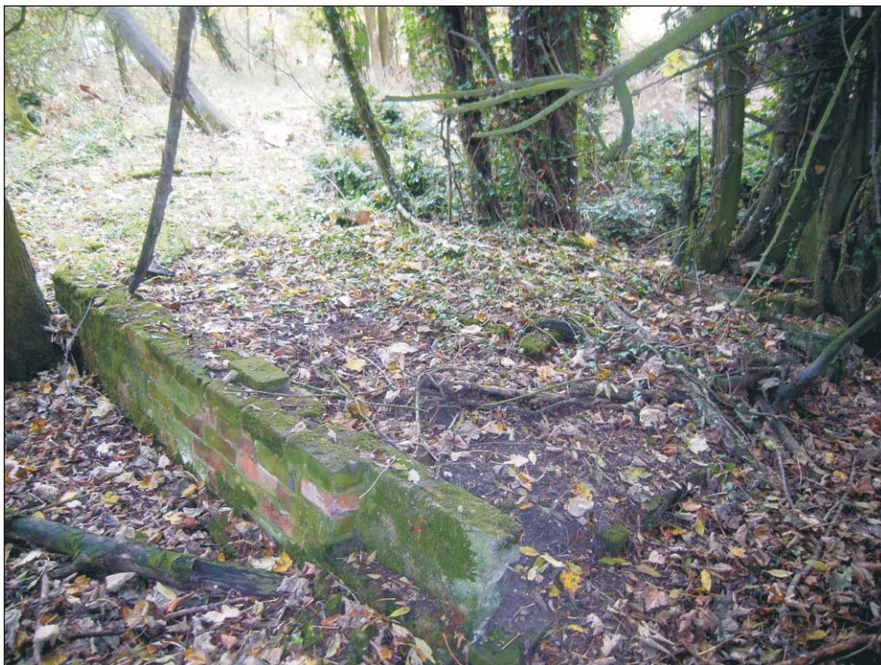
Plate 8: West end of Building 2 glasshouse foundation
