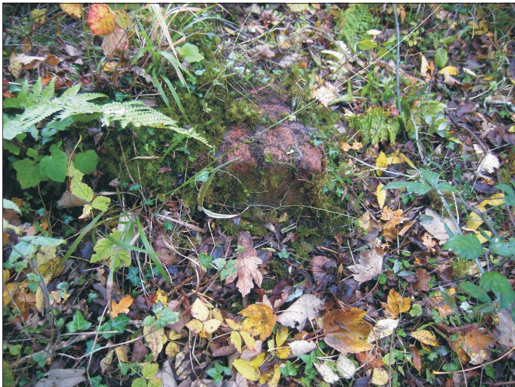
Plate 2: Remains of brick wall associated with Building 8
