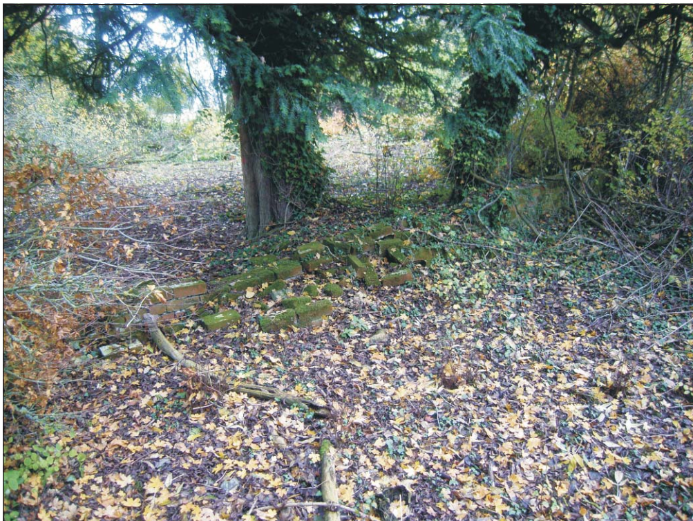
Plate 4: Section of boundary wall between house and stable (Building 8)
