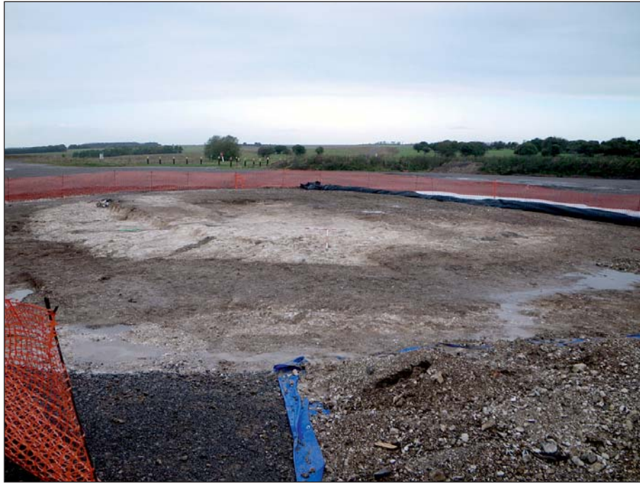
Plate 5: View of the Site from the east after cleaning
