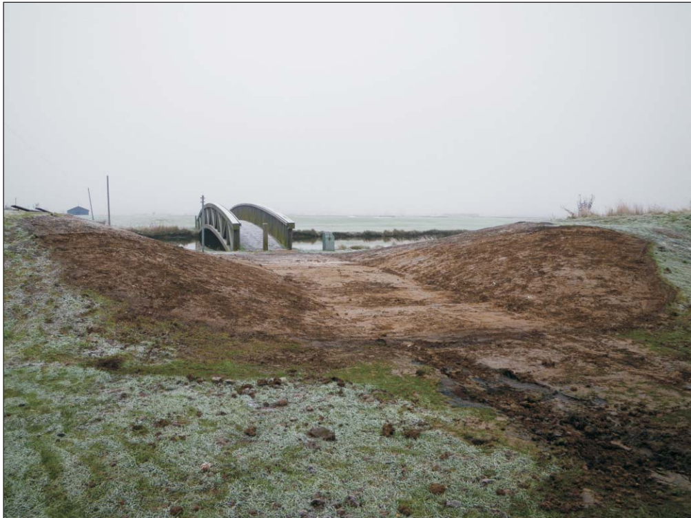
Plate 1: Excavation of cut through the Queenborough Lines
