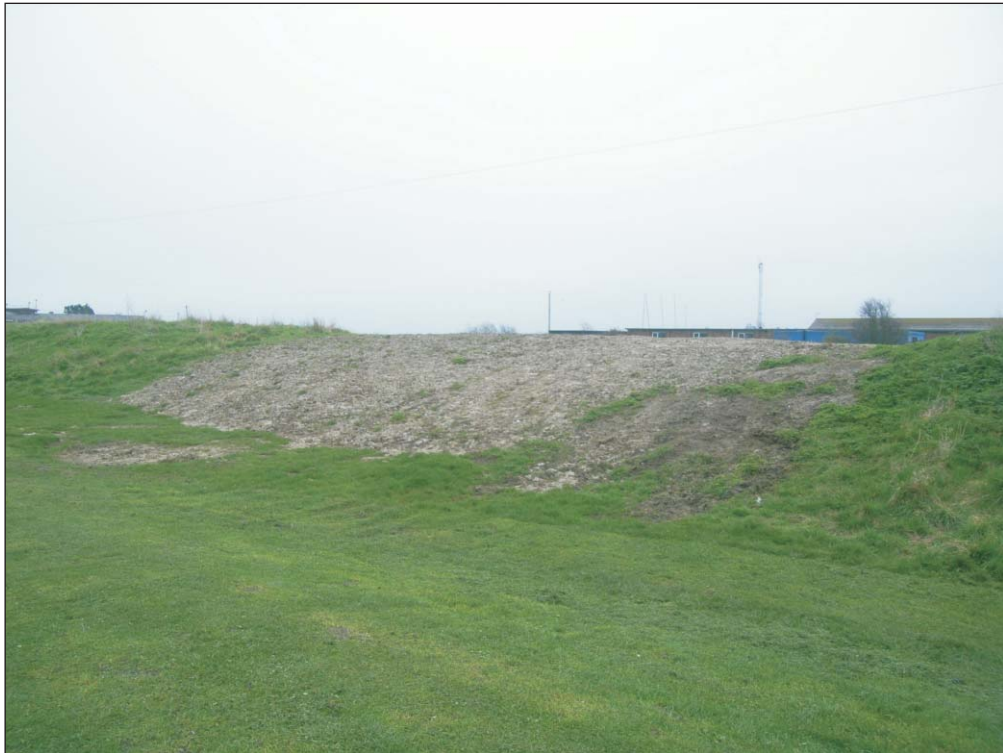
Plate 3: Infilled section of the Queenborough Lines
