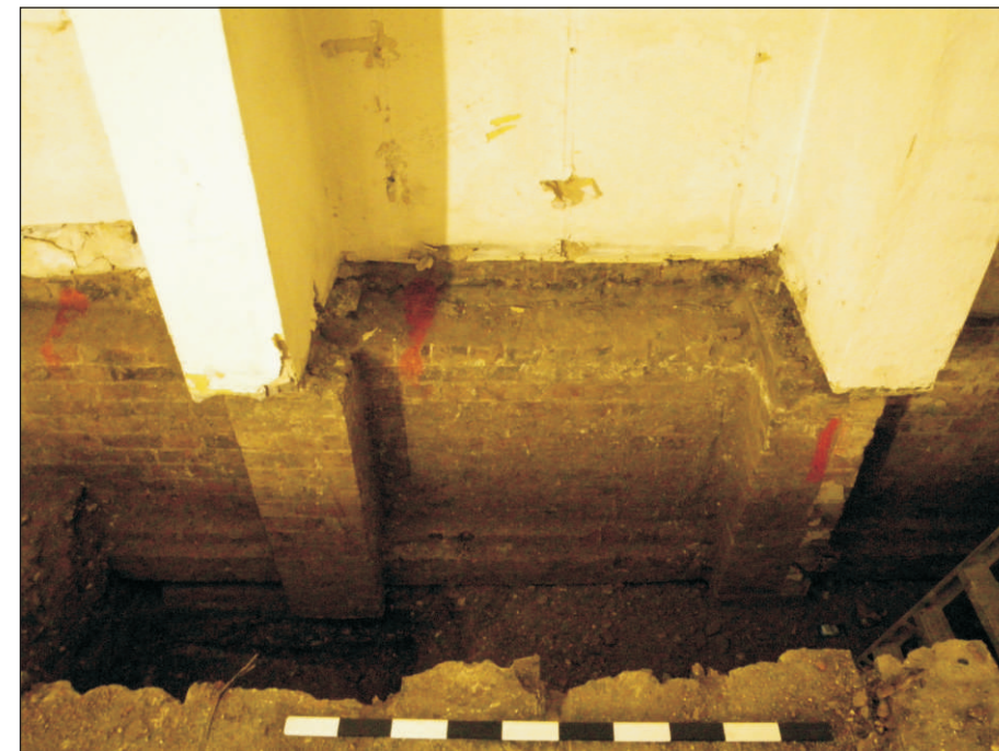
Plate 13: The White House foundations – internal face, view from north-west
