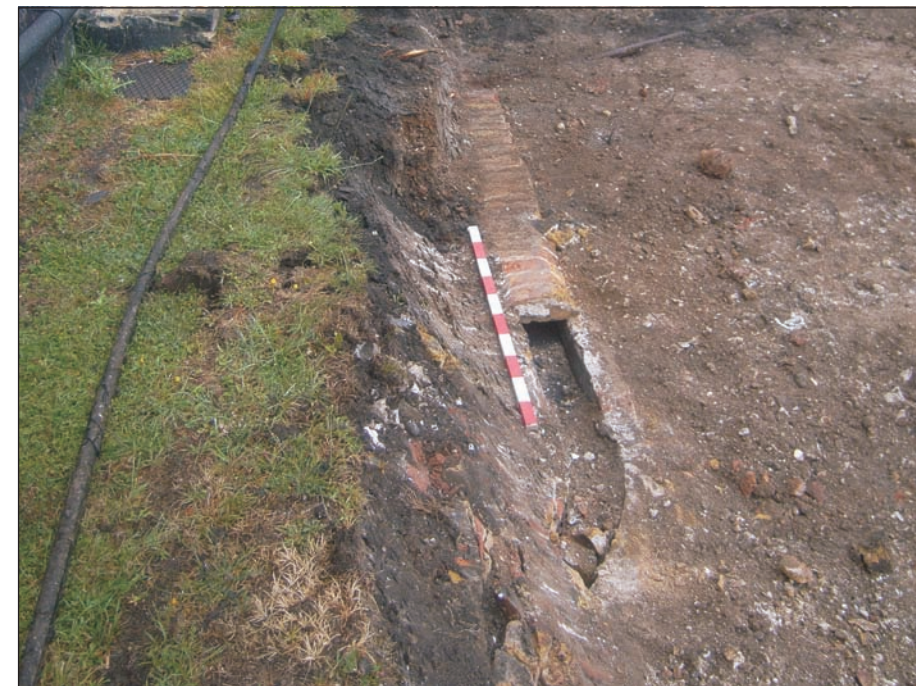
Plate 8: Brick culvert 106, view from south-east
