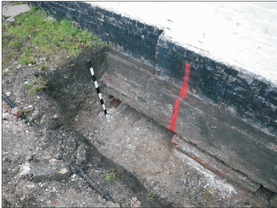
Plate 9: The White House foundations, showing made ground layer 1002, view from east
