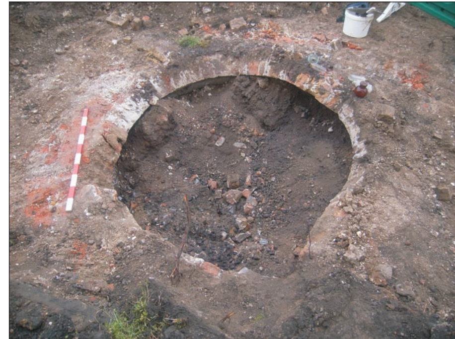
Plate 6: Water tank 103, view from east
