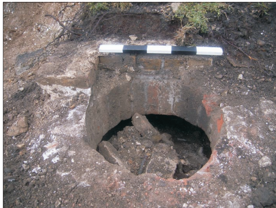
Plate 7: Water tank 108, view from east
