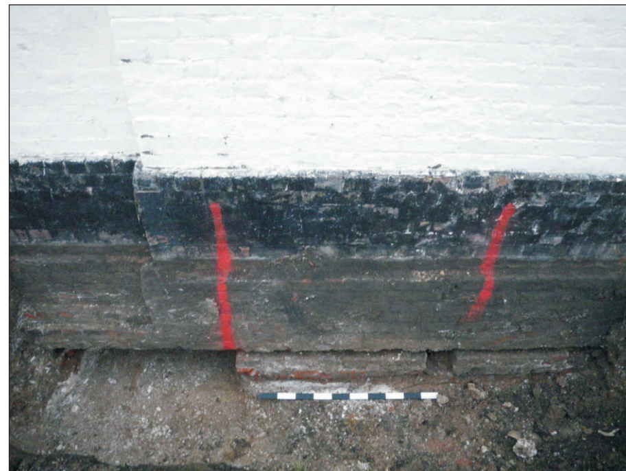
Plate 12: The White House foundations – external face, view from south-east
