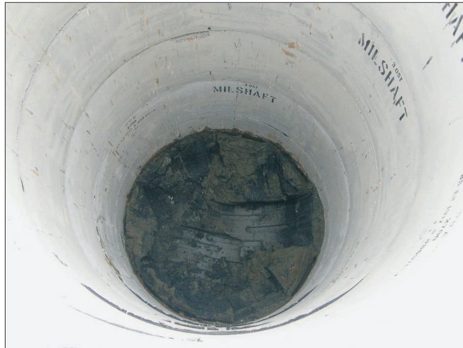
Plate 5: View of alluvium 128 in pumping station shaft
