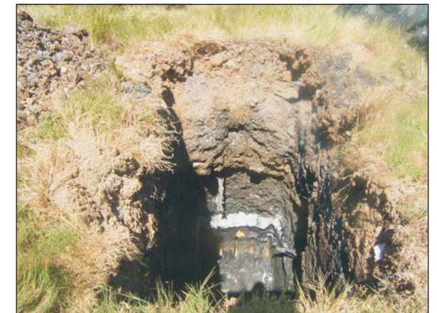
TP 21 viewed from the south
