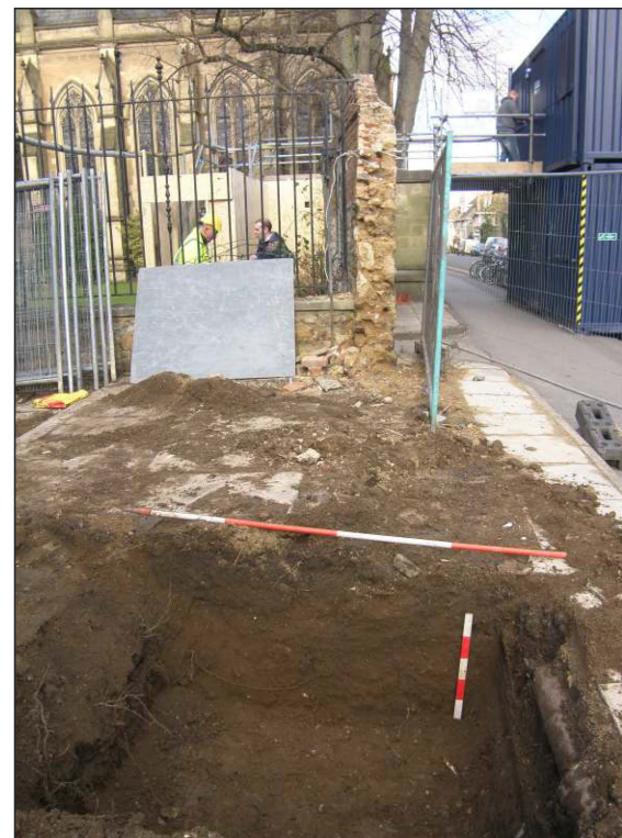
Plate 5: South facing section Trench 2 with remains of recently demolished Grade II listed boundary wall in background (scale 2m, 1m)
