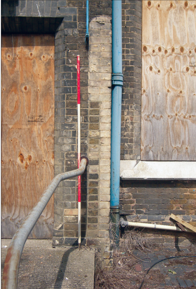
Plate 3: South facing view showing wall scar 1011
