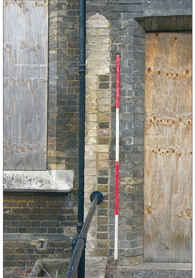
Plate 4: South facing view showing wall scar 1114
