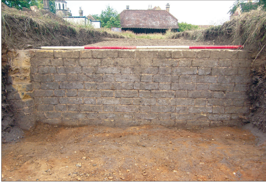
Plate 7: East facing elevation of wall 1114
