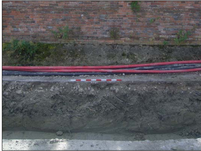
Plate 1: North facing representative section showing old ground surface/occupation layer 3 with perimeter wall in background
