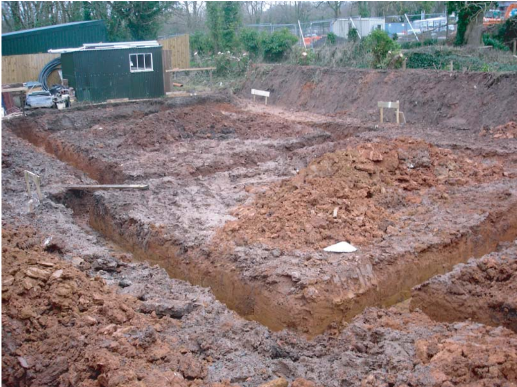
Plate 1: View of the foundation trenches from the east
