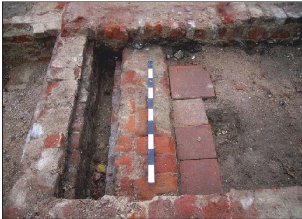
Plate 4: Detail of eastern side of Phase 1 corridor (Room 17), viewed from the south, showing the adjacent tile-capped drain
