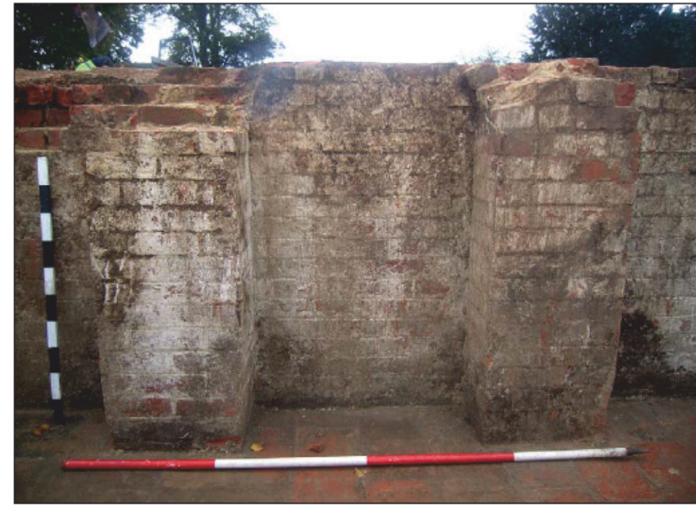
Plate 15: Chimney base in the cellar (Room 1) associated with the postulated kitchen above, viewed from the north
