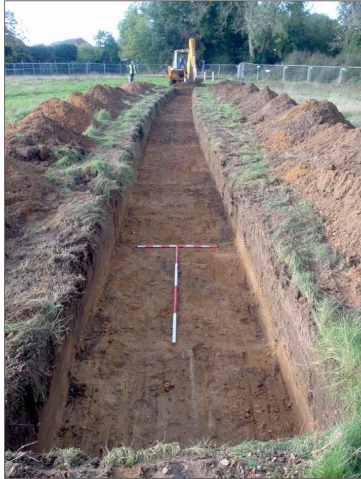
Plate 1: Trench 4, view from east
