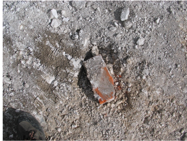
Brick exposed in base of Switch Room excavations
