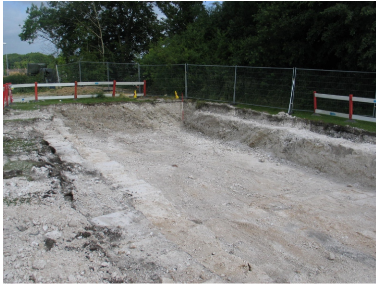
Switch Room excavation complete, viewed from the south-east
