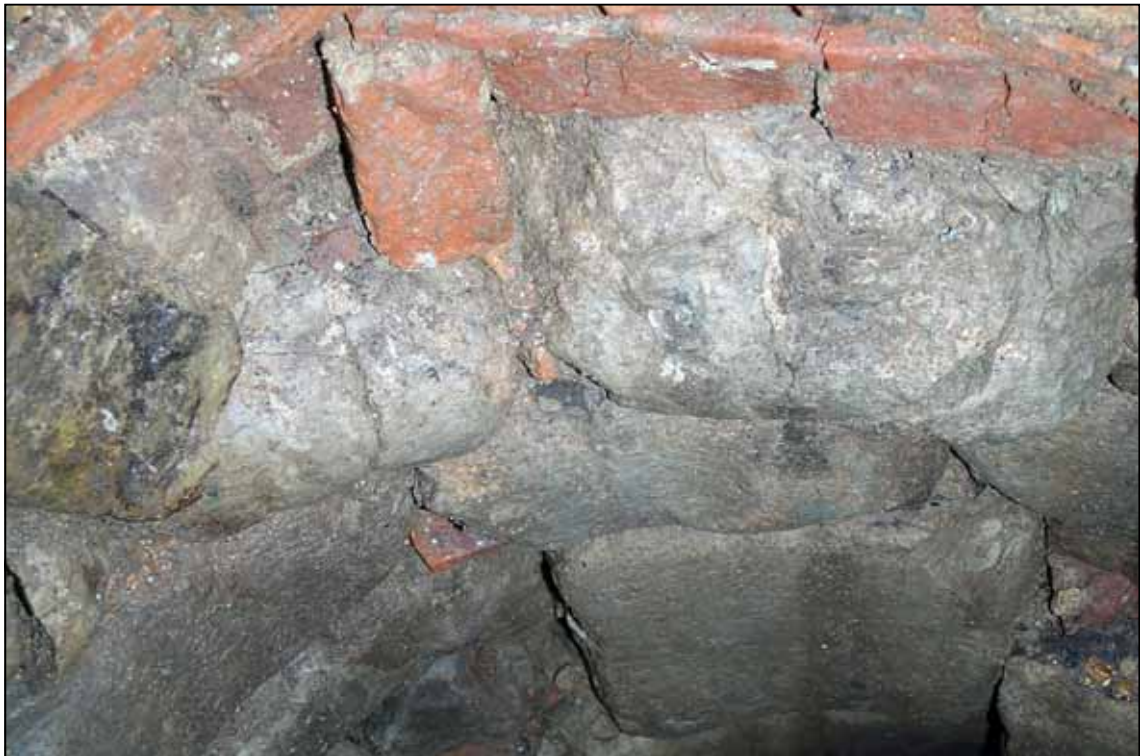
Brick and soft grey stone lining of well 105
