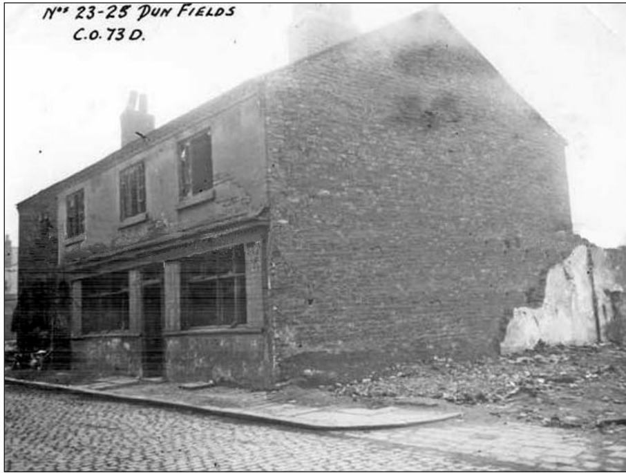
Historic Photo of the New Red House Inn (Picture Sheffield Ref: u00710)
