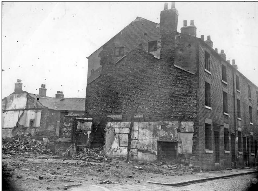
Historic Photo of No 33 Dun Fields showing damage on its western gable indicating the height of the buildings on Site (Picture Sheffield Ref: u00711)
