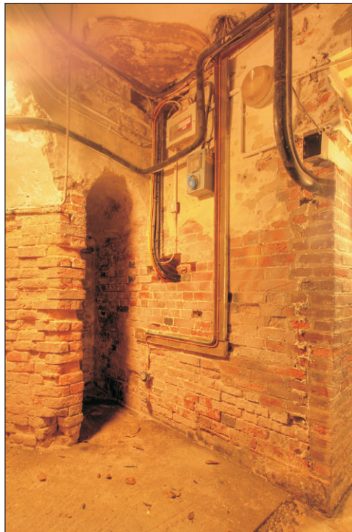
Plate 26: Basement end passageway following paint removal viewed from the south-west
