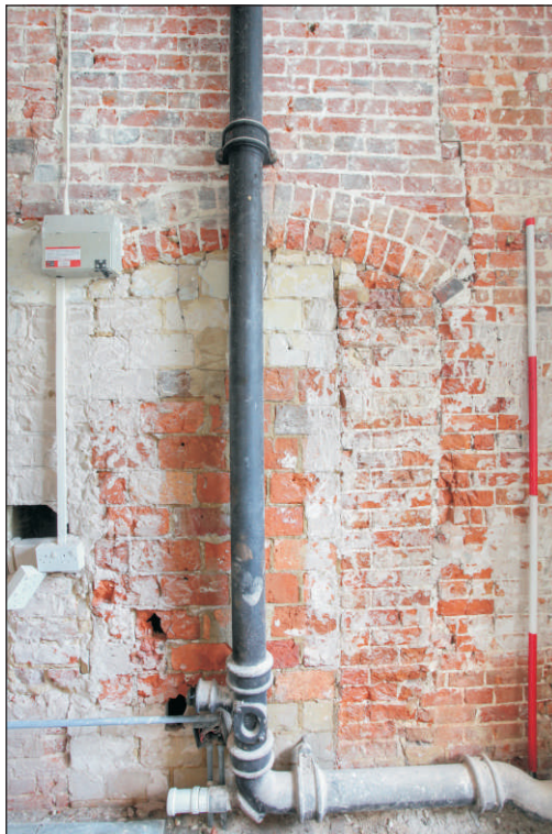
Plate 2: Room RG 08 – Blocked door viewed from the east
