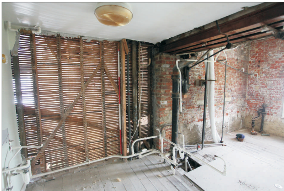
Plate 22: Room 209 – South section of timber studwork viewed from the east
