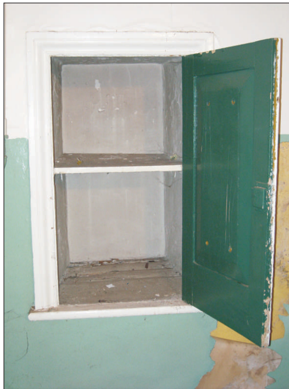
Plate 10: Room RG 07 – Small cupboard on north wall prior to remedial works
