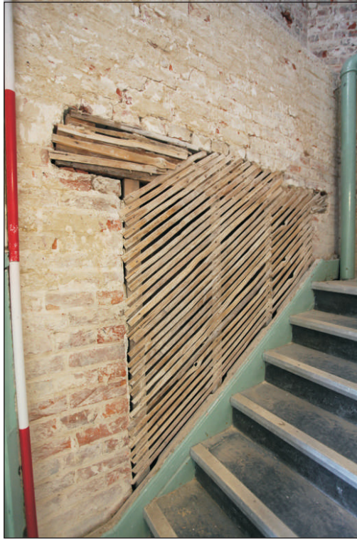
Plate 17: Room 208 – Exposed north-west wall revealing blocked window opening
