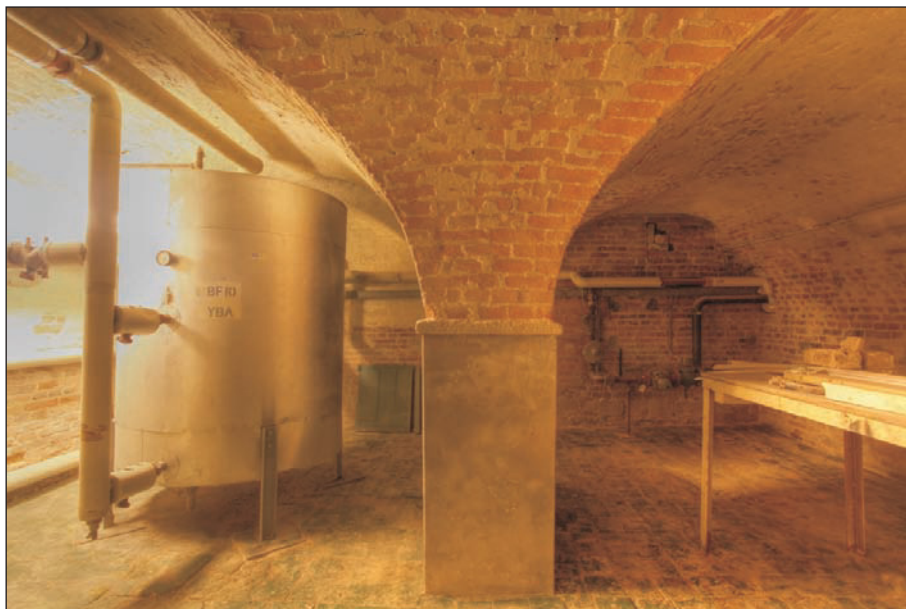
Plate 24: Room RB04 following paint removal viewed from the north
