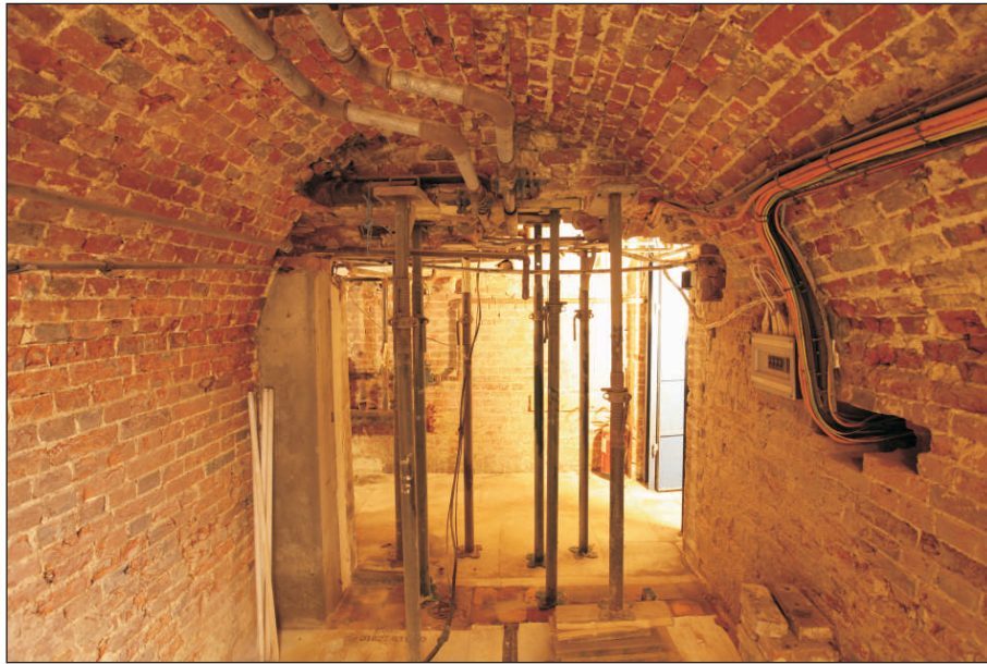
Plate 33: Room RB08 – lintel removed above doorway currently propped
