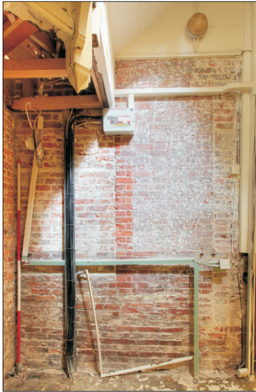
Plate 9: Room RG 07 – Exposed east wall of the Stairwell showing blocked window
