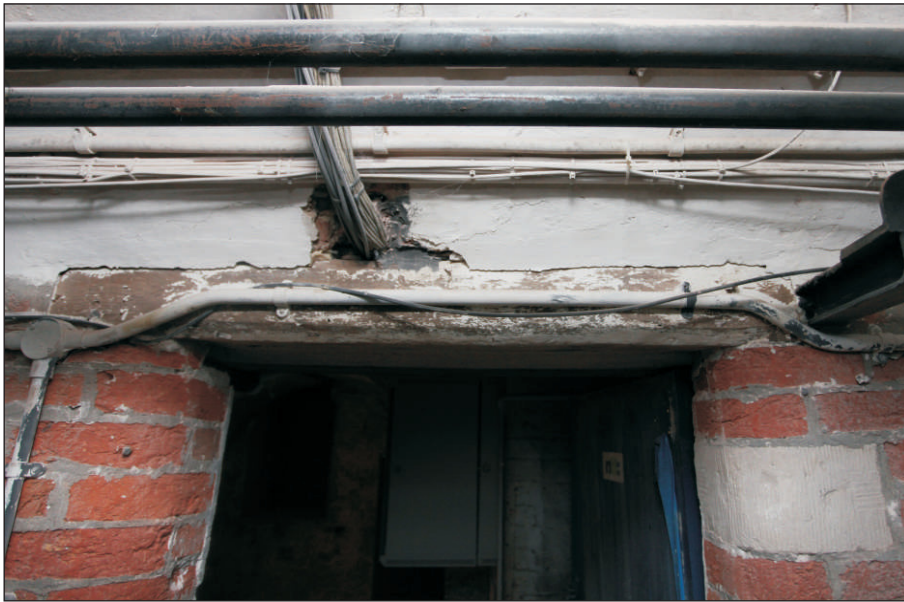
Plate 30: Room RB10 – plain stopped and chamfered timber over entrance
