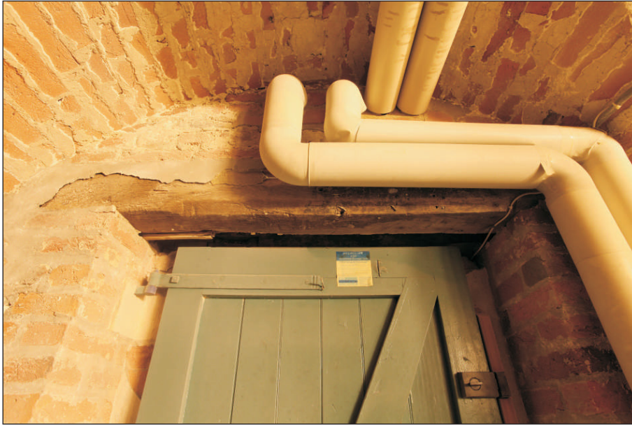
Plate 29: Room RB04 – plain stopped and chamfered timber over entrance
