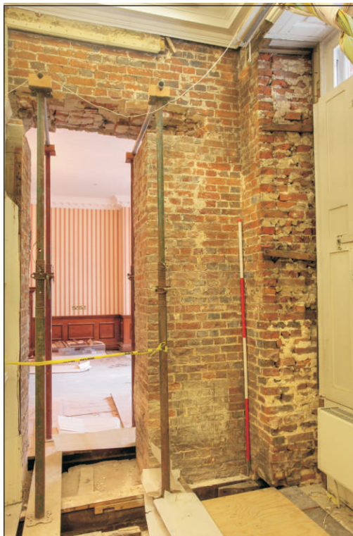
Plate 6: Room RG 04 – Exposed doorway viewed from the west
