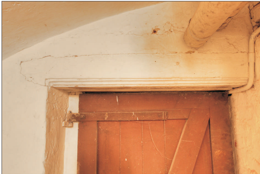
Plate 31: Room RB03 – Reused moulded timber from square-headed doorway
