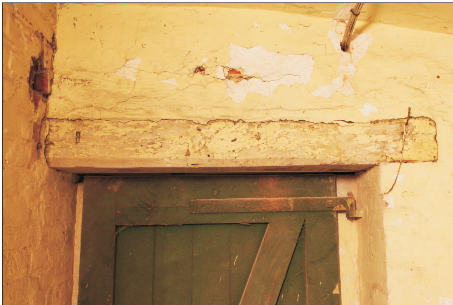
Plate 28: Room RB02 – plain stopped and chamfered timber over entrance
