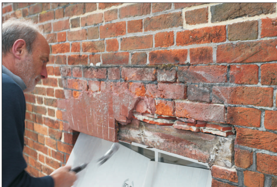
Plate 36: Second floor windows – removal of false cement arch using hand tools
