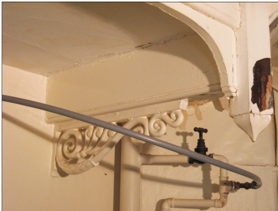
Plate 14: Room RG 07 – Scrolled cast iron bracket viewed from the south-east
