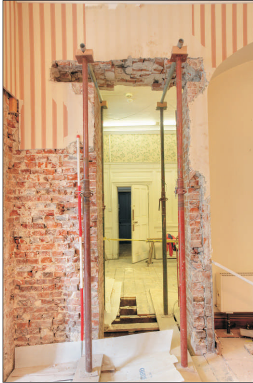
Plate 5: Room RG 03 – Exposed doorway viewed from the east
