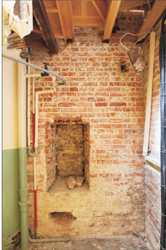
Plate 11: Room RG 07 – Exposed north wall showing former cupboard recess
