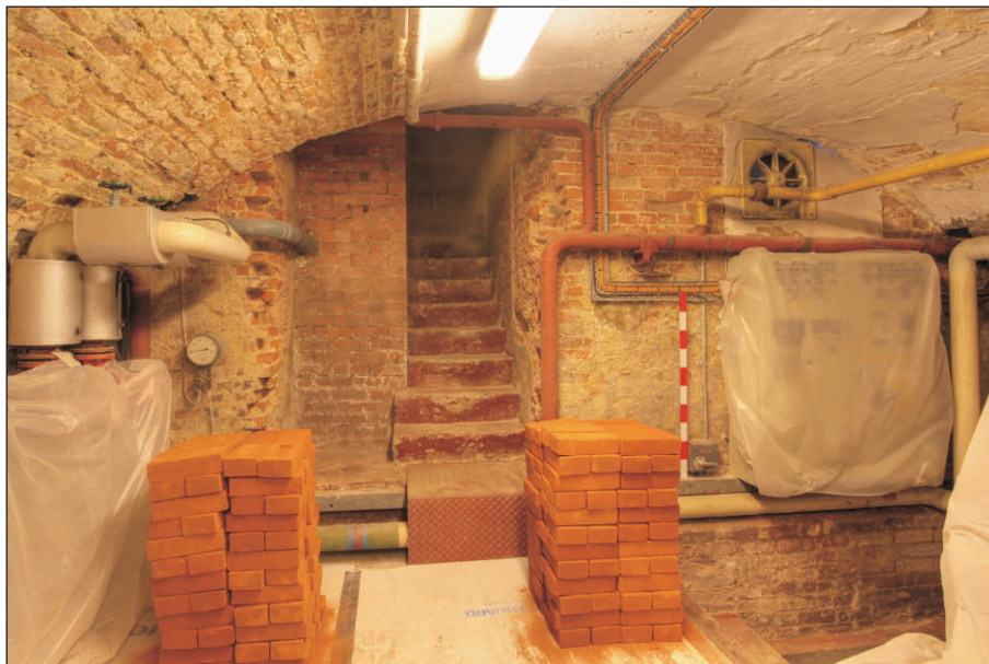
Plate 35: Room RB05 – later inserted entrance and steps on south wall
