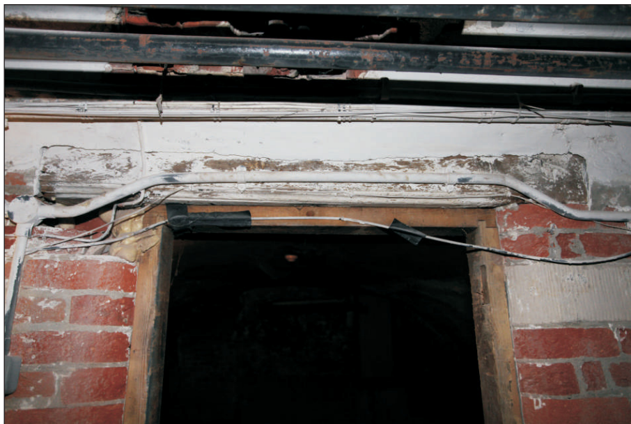
Plate 32: Room RB09 – Reused moulded timber from square-headed doorway
