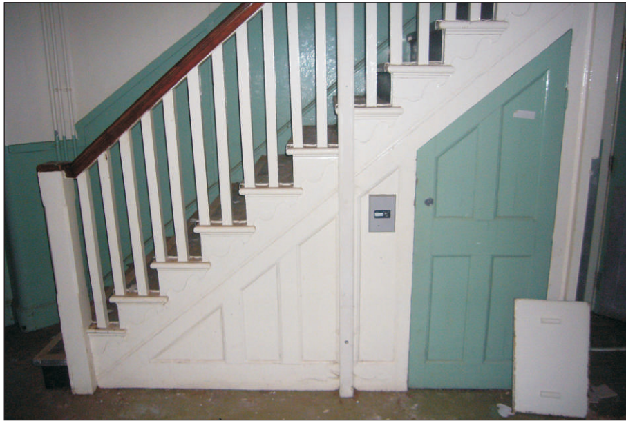
Plate 13: Room RF 07 – Base of staircase viewed from the east
