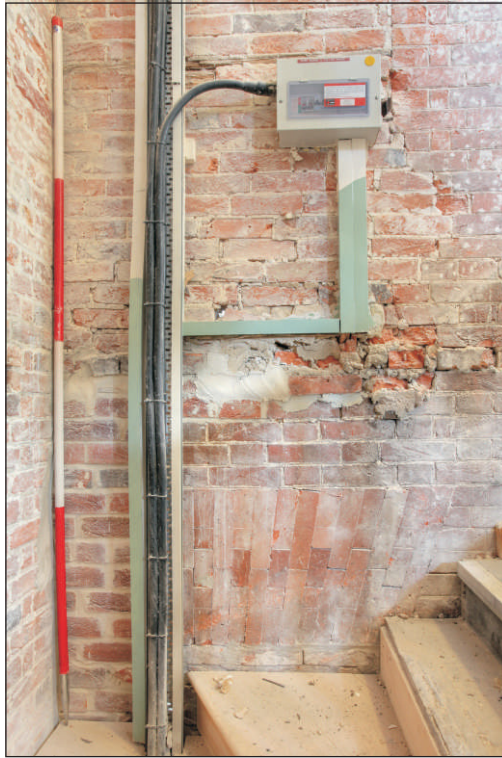
Plate 15: Room 108 – Exposed east wall showing rubbed brick arch
