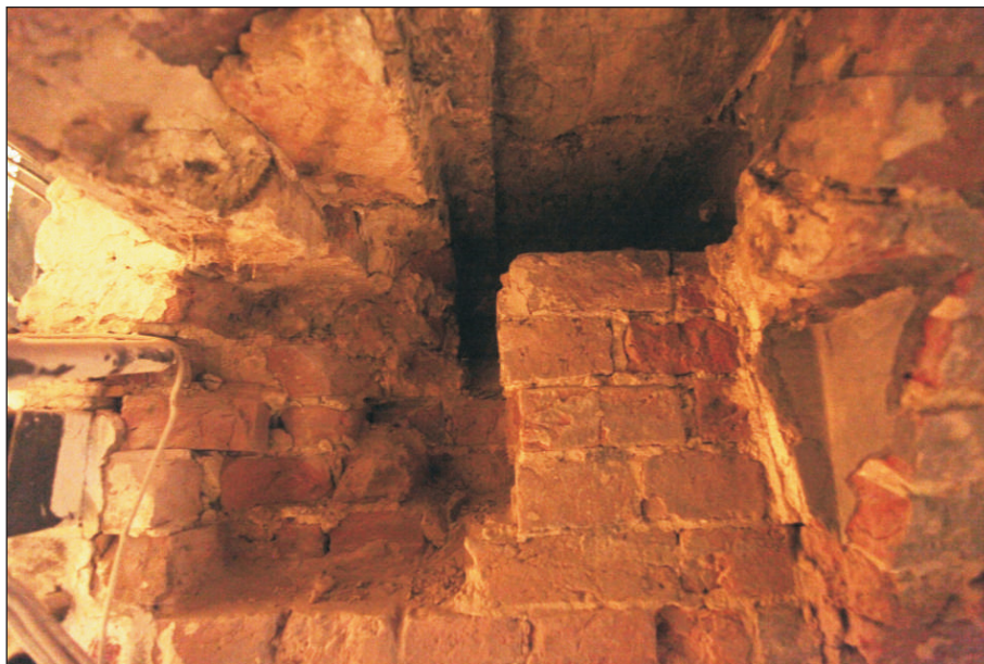
Plate 34: Room RB08 – detail of lintel socket viewed from the east
