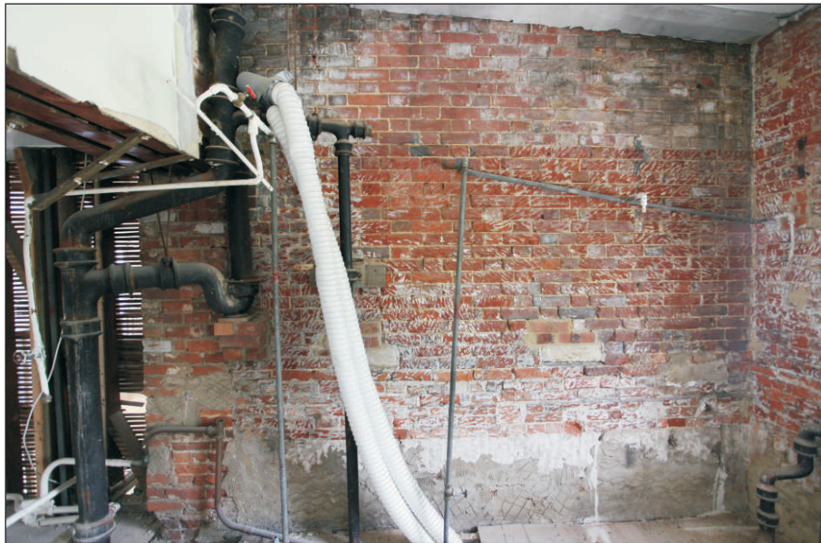
Plate 21: Room 209 – North section of wall viewed from the east
