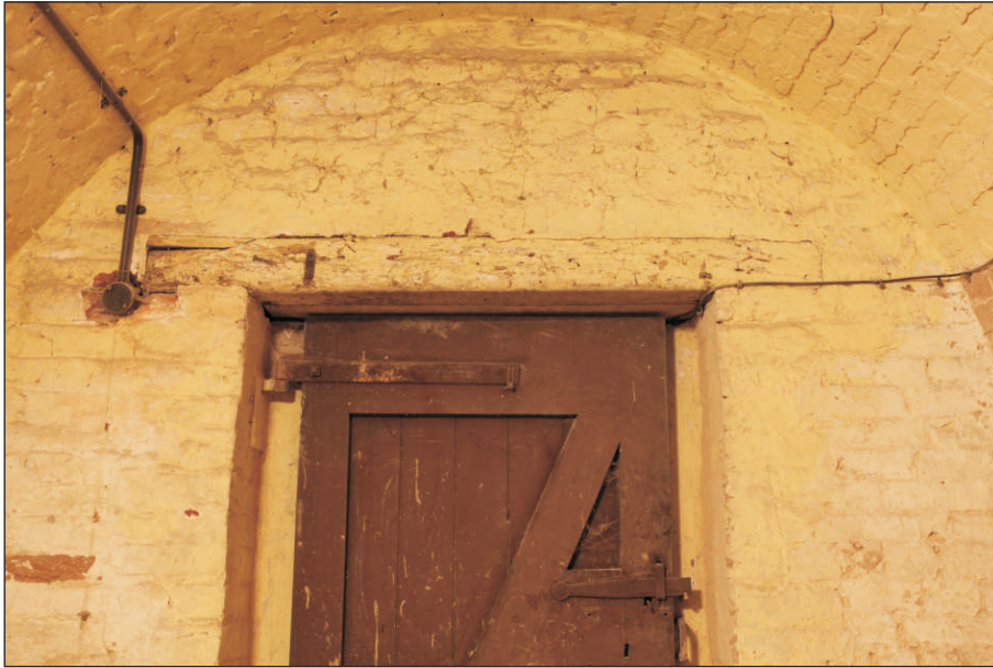
Plate 27: Room RB01 – plain lintel viewed from the south
