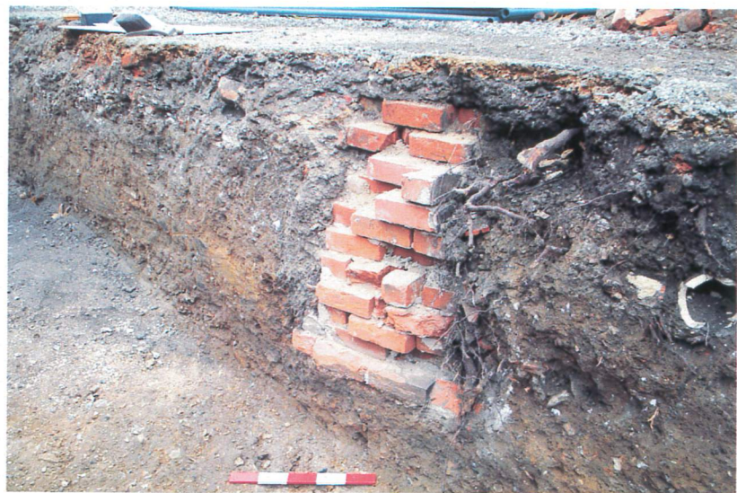
Plate 3: View of south wall footing (3006) of the Victorian schoolhouse, cut into make-up deposits and quarry backfills. Natural gravels are exposed in the base of the trench. Looking north-east, scale 0.5m
