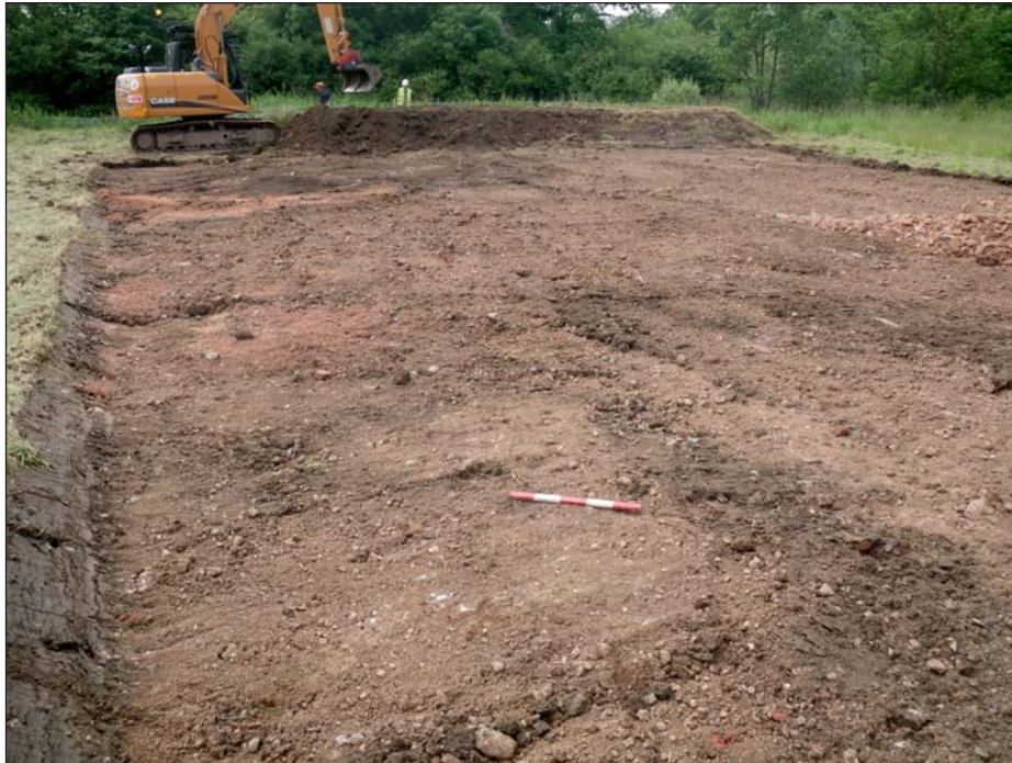
Plate 1: Topsoil strip in Trench 1
