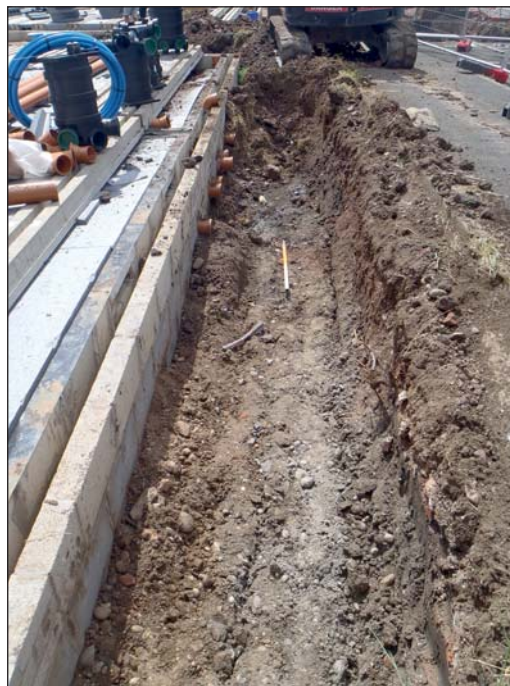
Plate 2: Foundation and pipeline excavation in Trench 8
