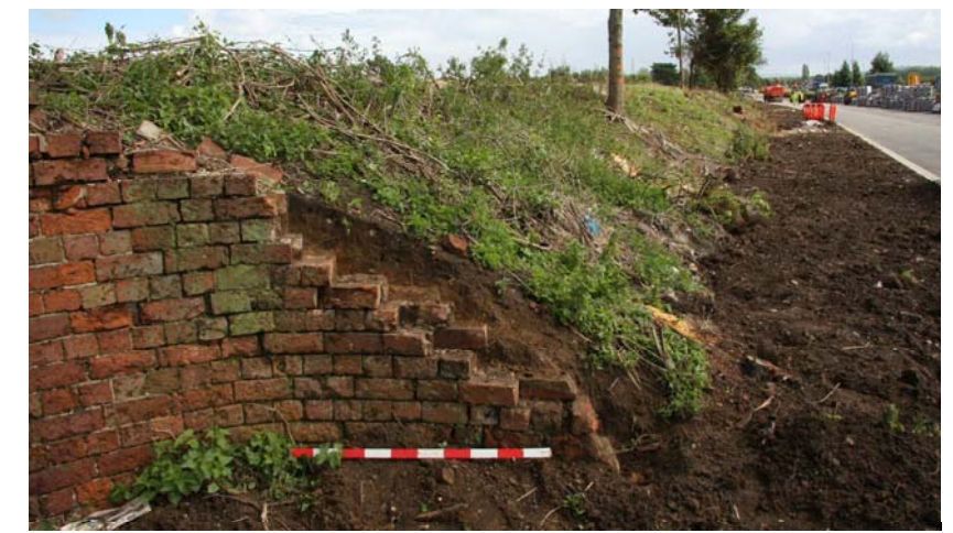
Plate 4: Detail of bus stop brickwork
