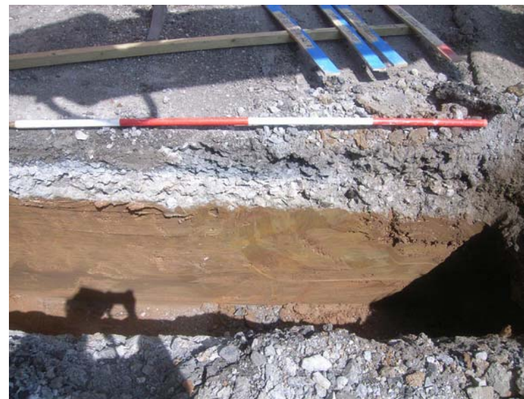
Plate 2: East facing section on central reservation
