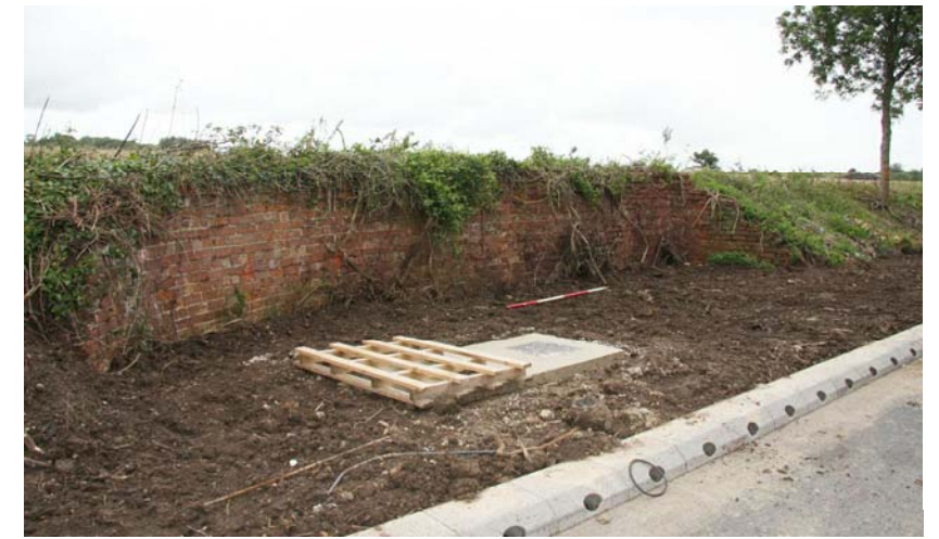
Plate 3: View of bus stop from south-west
