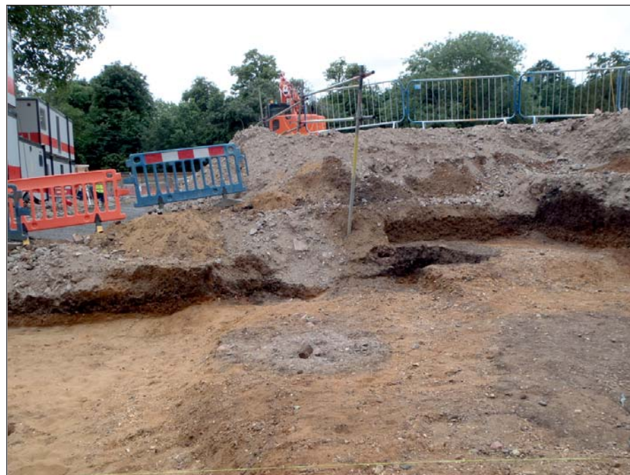
Plate 5: East facing section of Phase 3, Area 3
