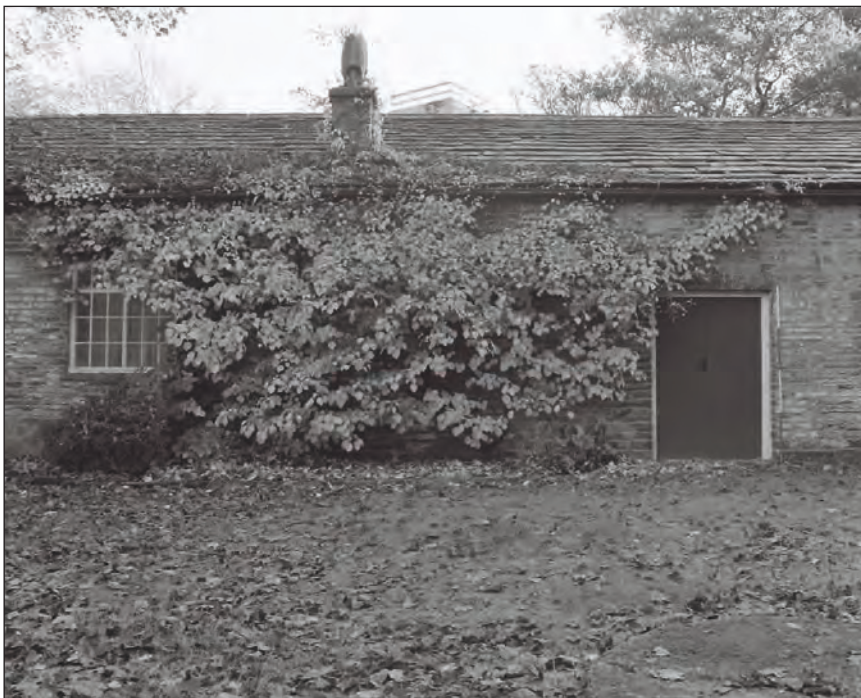
Plate 24: View of the southwest elevation of the former anvil store and workshop range (Film 1.4)
