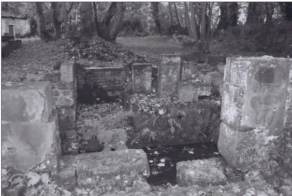
Plate 51: View of remains of wheel pit 4 adjacent to former grinding shop, south-eastern side of the central phase 1 former forge building (Film 9.14)
