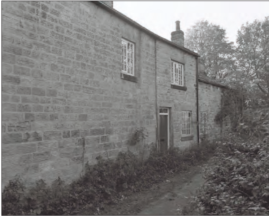
Plate 7: General view of the northwest elevation of the former Manager's House and attached furnace, Mousehole Forge (Film 3.2)
