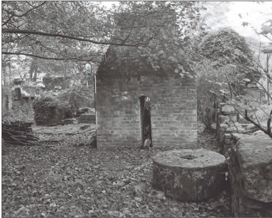
Plate 109: General 'internal' view of the eastern phase 3 range, showing rear of chimney and grinding wheel (Film 3.10)
