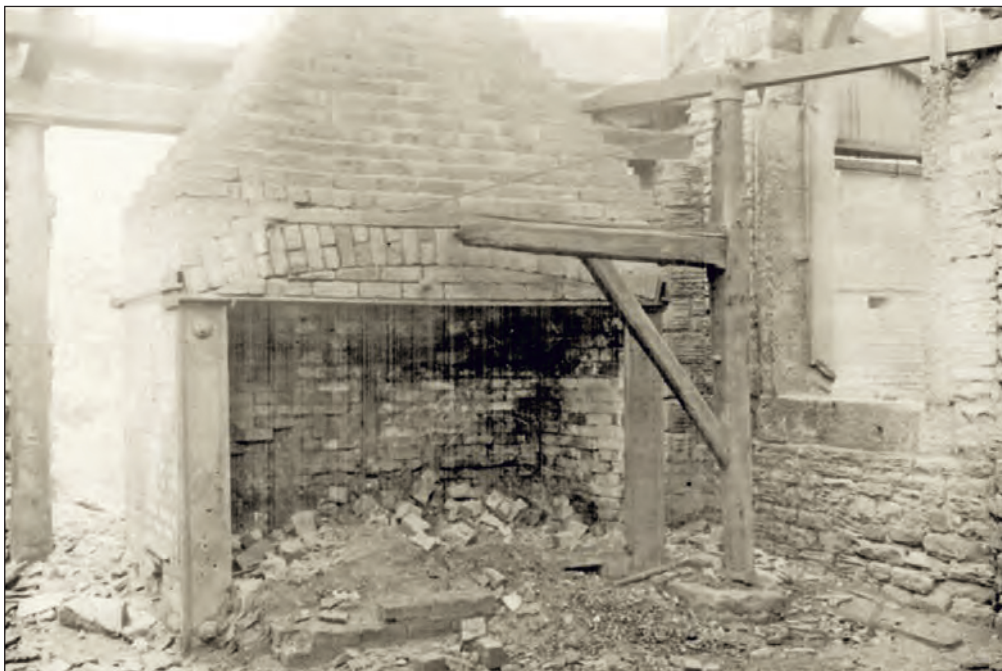
Plate 43: Historic view of the remains of the western hearth within the central phase 1 former forge building (Baker, 1940. Picture Sheffield Ref. y01186)
