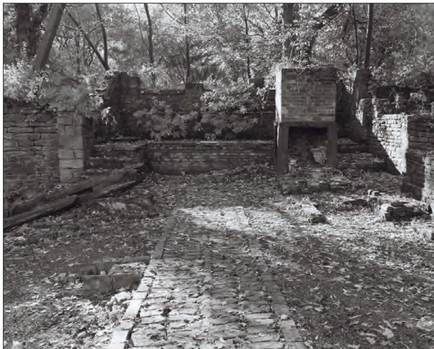
Plate 92: General view of the western phase 3 range (Film 5.10)
