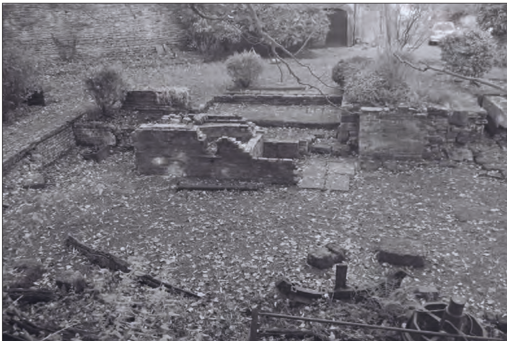
Plate 80: General view of the western phase 2 range from dam wall, showing remains of a puddling furnace (Film 11.11)
