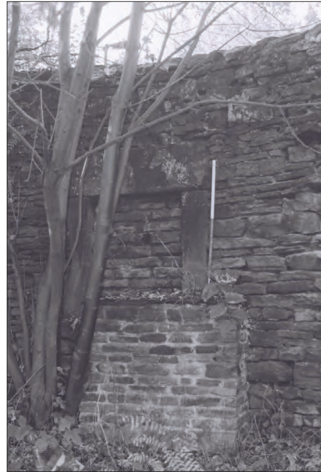
Plate 102: Detail of blocked opening within the western boundary stone wall (Film 10.33)
