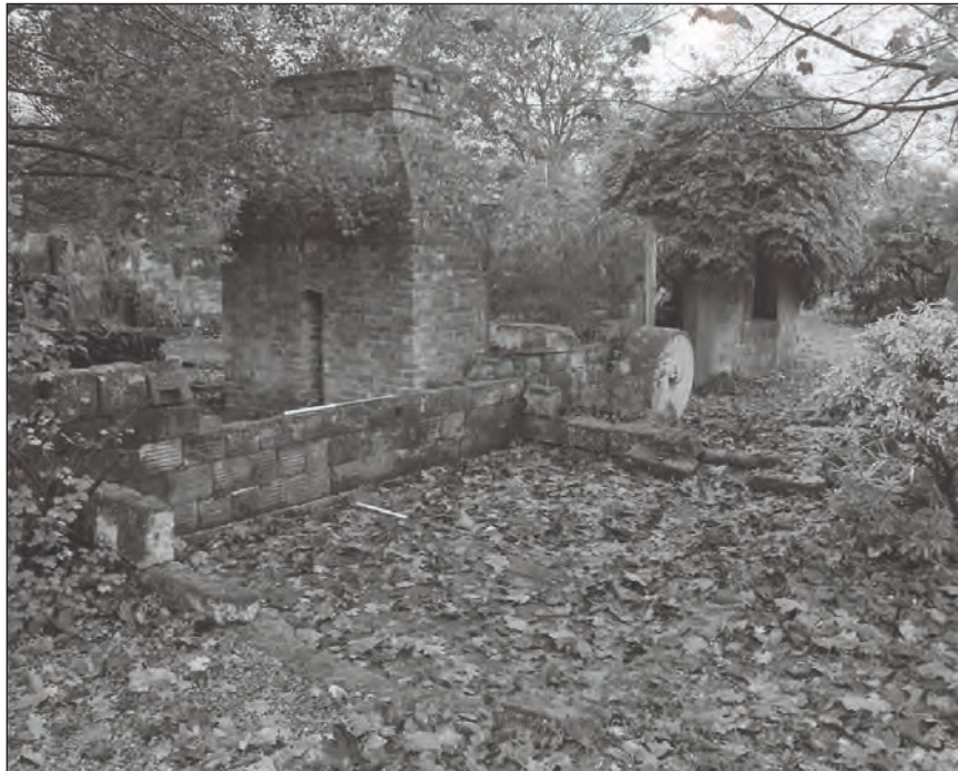
Plate 38: General view of the central phase 1 former forge building, showing truncated hearth and chimney stack and attached former joiners shop (Film 3.7)
