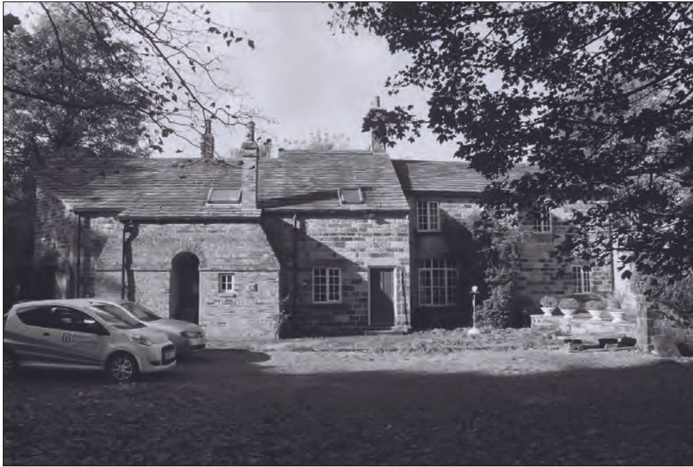
Plate 13: General view of the southeast elevation of the former Manager's House and attached furnace (Film 7.22)
