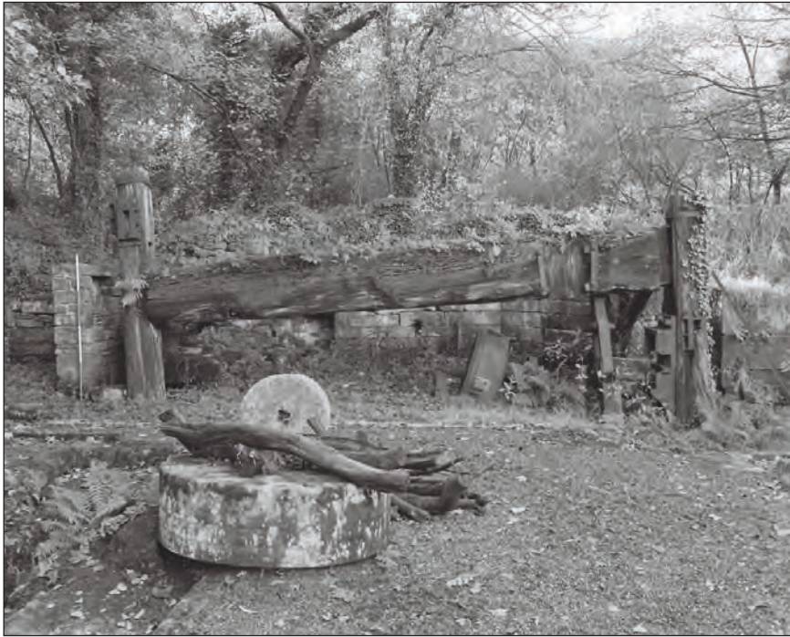
Plate 58: General view of the remaining east helve hammer, south end of the central phase 1 former forge building (Film 4.5)
