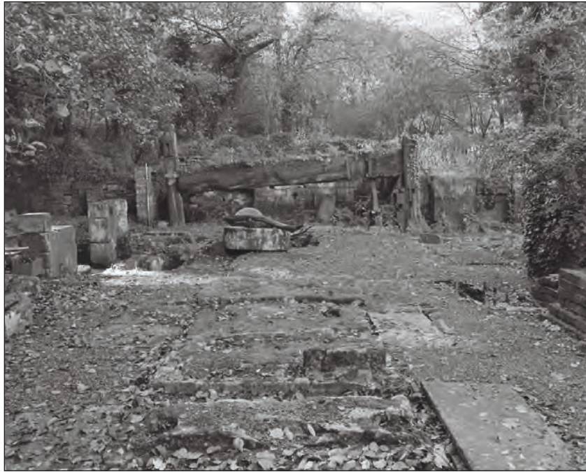
Plate 39: General (internal) view of the central phase 1 former forge building, showing steam hammer base, surviving east helve hammer and dam wall (Film 4.3)
