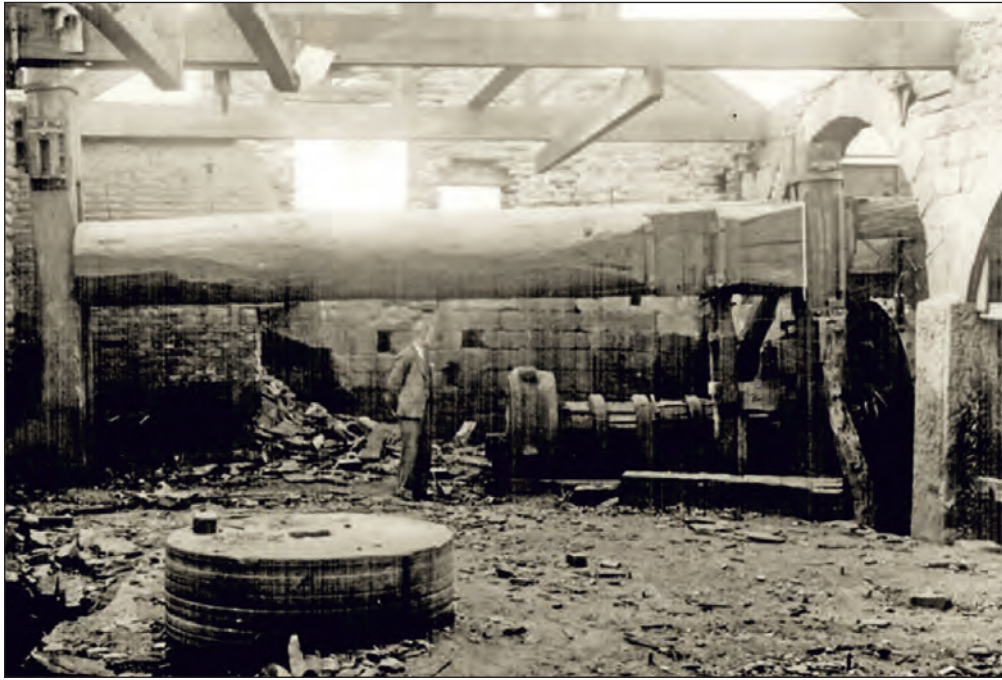
Plate 60: Historic view of the east helve hammer, south end of the central phase 1 former forge building (Baker, 1940. Picture Sheffield Ref. y01191)
