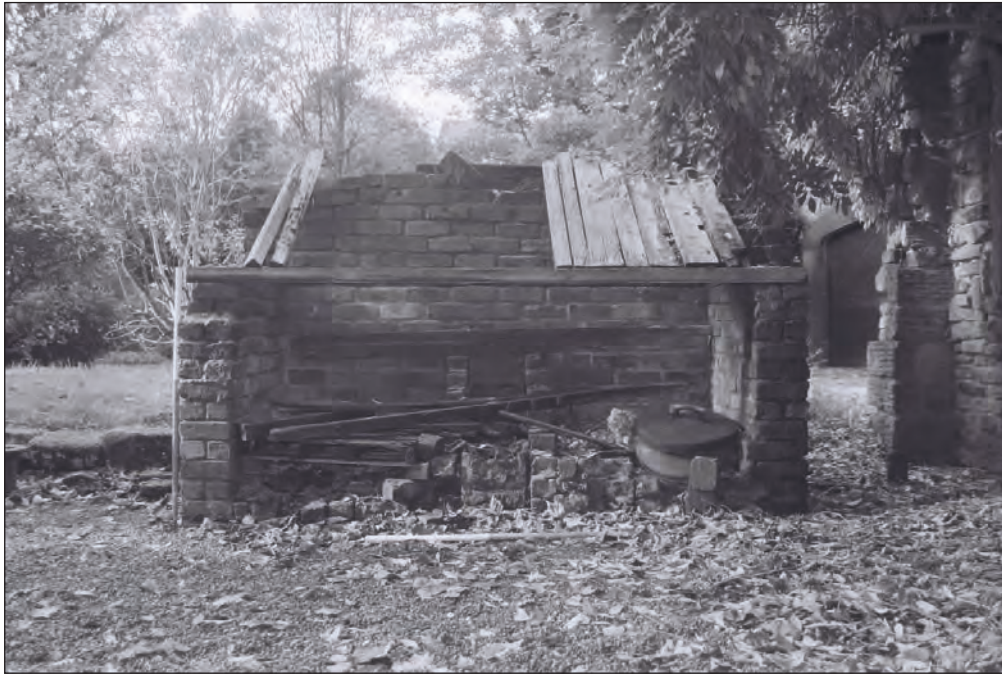
Plate 42: Detail of the remains of the western hearth within the central phase 1 former forge building (Film 8.20)
