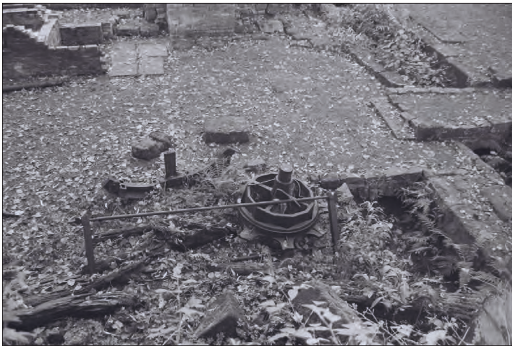
Plate 72: General view of the collapsed west helve hammer from the dam wall at the south end of the phase 2 range (Film 11.12)
