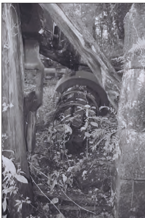
Plate 69: Detail of the cam wheel at the west end of the east helve hammer, south end of the central phase 1 former forge building, from the adjacent wheel pit (Film 9.36)
