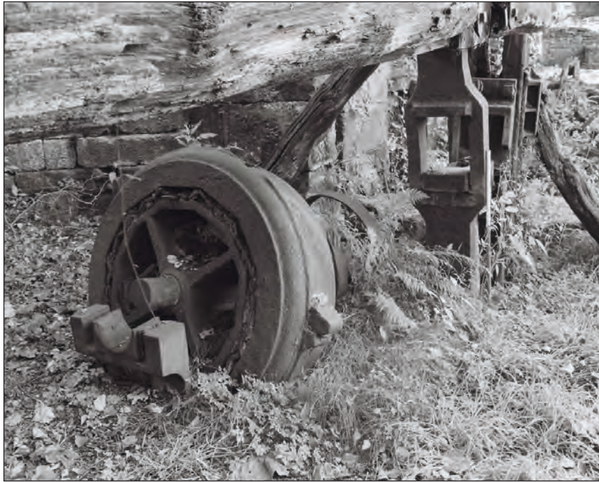
Plate 65: Detail of the cam wheel at the west end of the east helve hammer, south end of the central phase 1 former forge building (Film 5.6)
