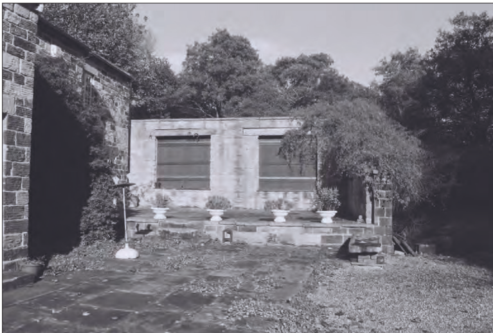
Plate 16: General view of the remains of the former office, looking north (Film 7.23)
