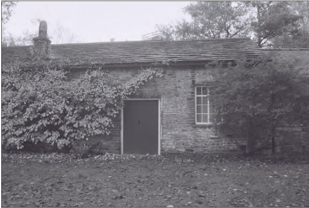
Plate 25: View of the southwest elevation of the former anvil store and workshop range (Film 7.28)
