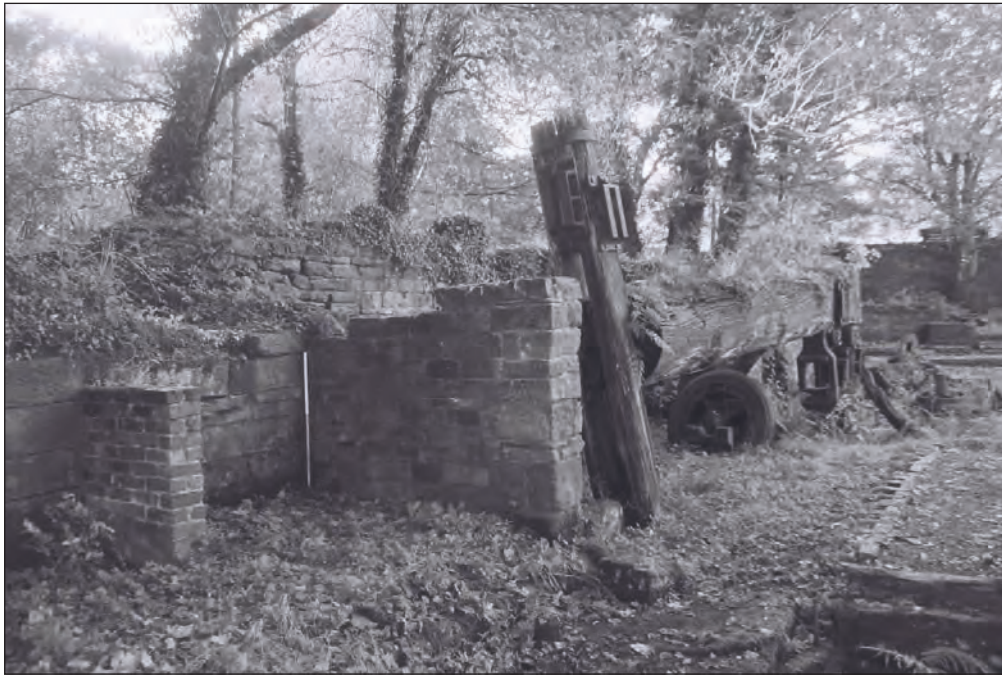
Plate 61: General view of the remaining east helve hammer and dam wall, south end of the central phase 1 former forge building (Film 9.24)
