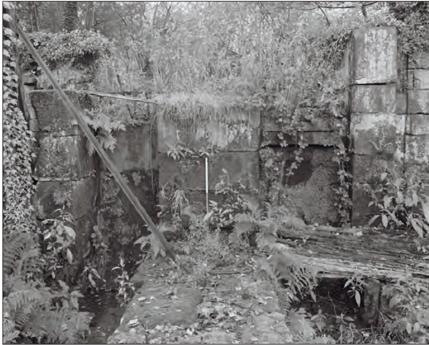
Plate 73: General view of wheel pits 1 and 2, sluices and dam wall (Film 5.7)
