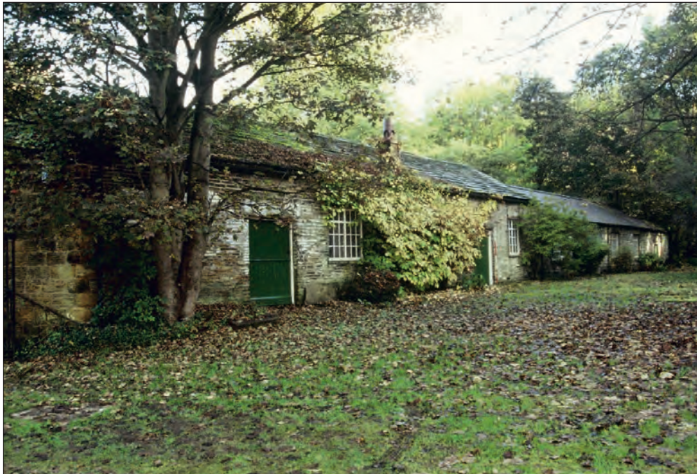
Plate 22: General view of the southwest elevation of the former anvil store and workshop range (Film CS. 25)
