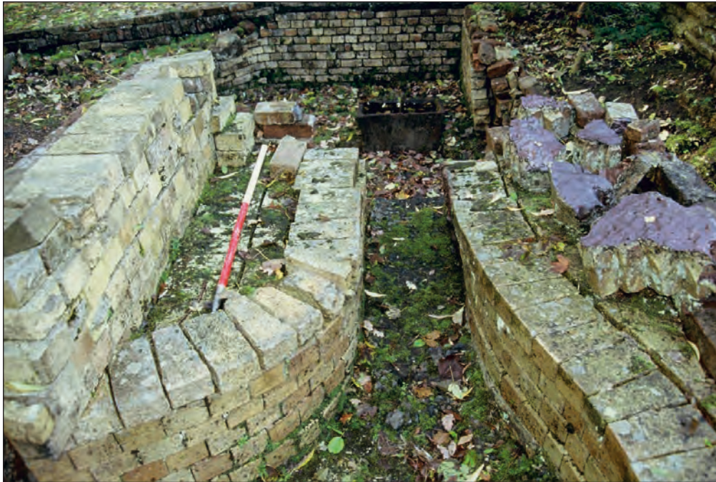
Plate 89: General view of the puddling furnace at north side of the western phase 2 range (Film CS. 7)
