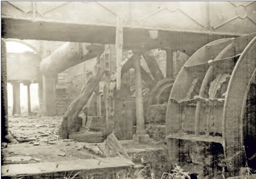
Plate 74: Historic view of wheel pits 1 and 2 and the east helve hammer beyond (Baker, 1940. Picture Sheffield Ref. y01187)
