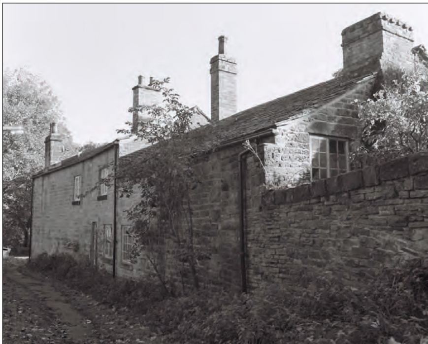
Plate 8: General view of the northwest elevation of the former Manager's House and attached furnace, Mousehole Forge (Film 3.1)
