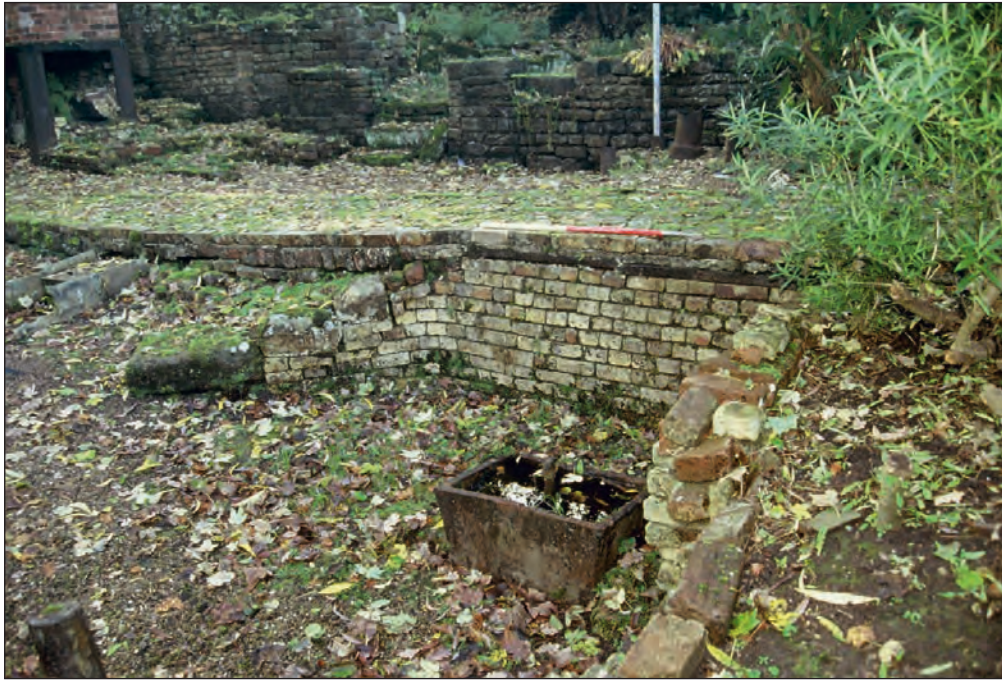
Plate 91: General view of the puddling furnace flue at north side of the western phase 2 range (Film CS. 3)
