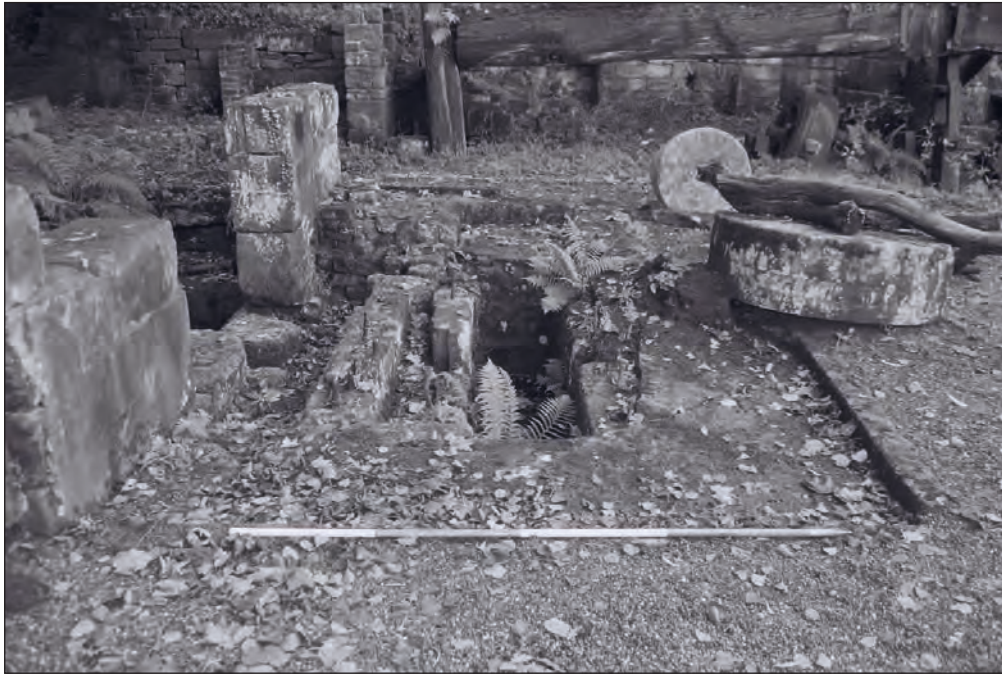
Plate 48: View of remains of structures and machine bases associated with grinding, adjacent to wheel pit, along the south-eastern side of the central phase 1 former forge building (Film 8.33)
