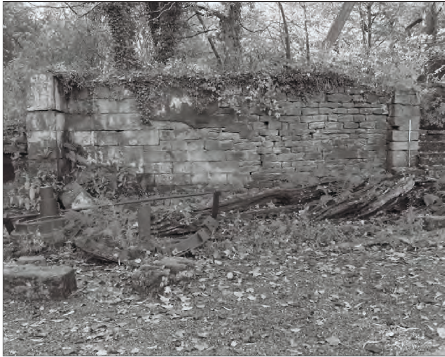
Plate 71: General view of the collapsed west helve hammer and dam wall at the south end of the phase 2 range (Film 5.8)
