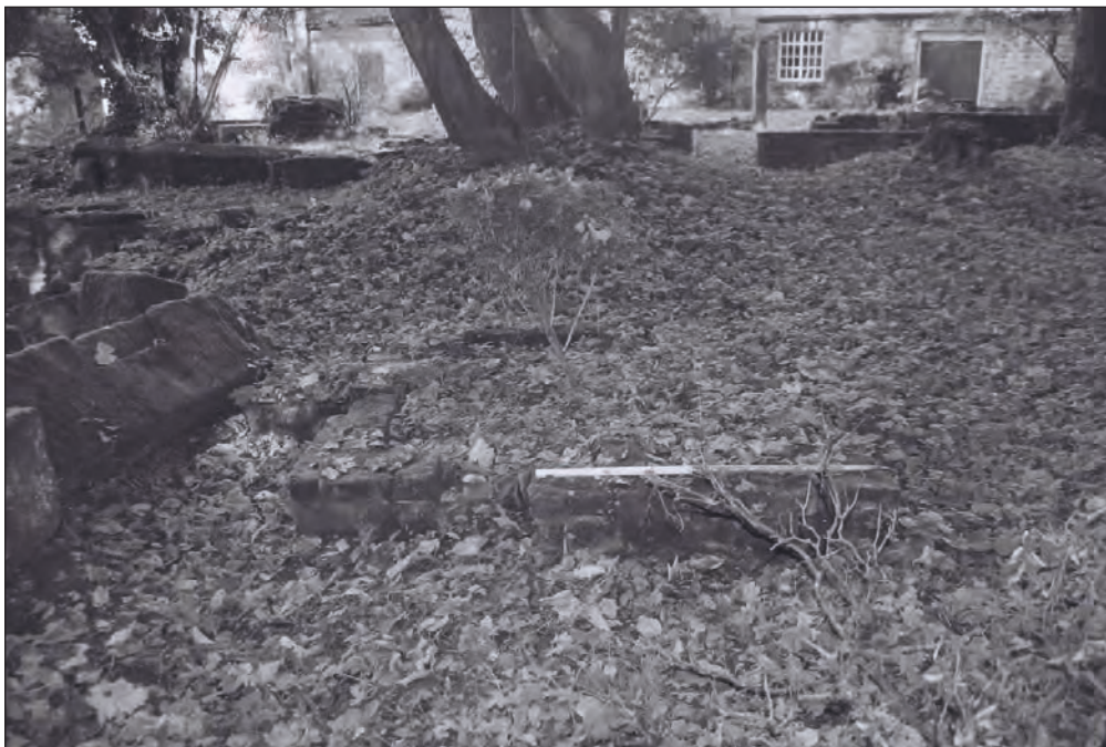
Plate 114: Detail of brick chimney base within the south-eastern phase 4 range (Film 9.18)
