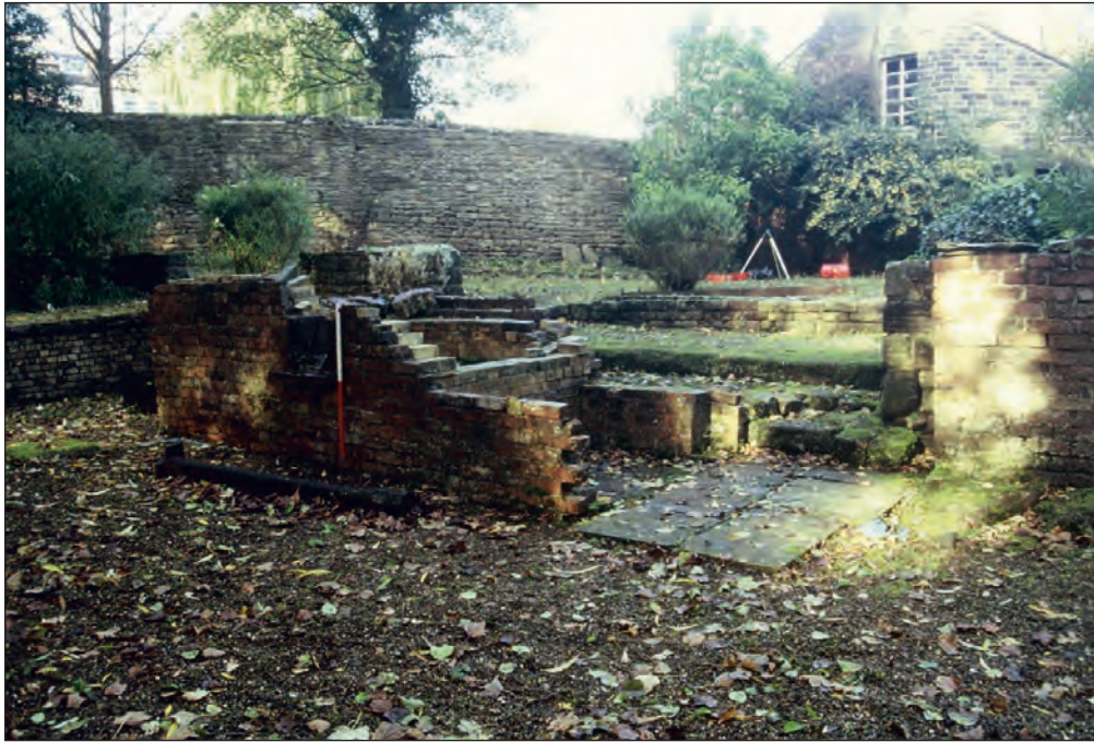
Plate 85: General view of a puddling furnace at north side of the western phase 2 range (Film CS. 13)
