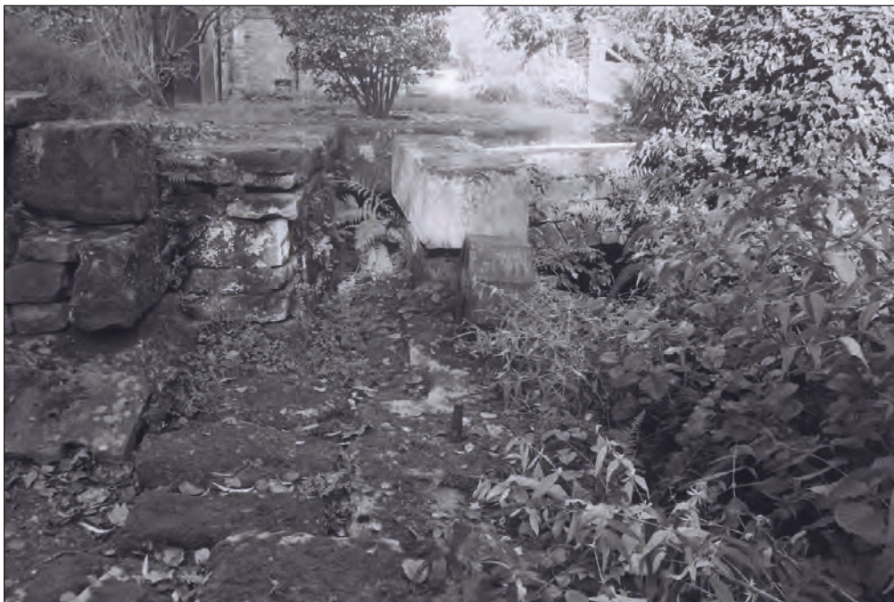
Plate 82: General view of wheel pit and structural remains at the north end of the western phase 2 range (Film 10.4)
