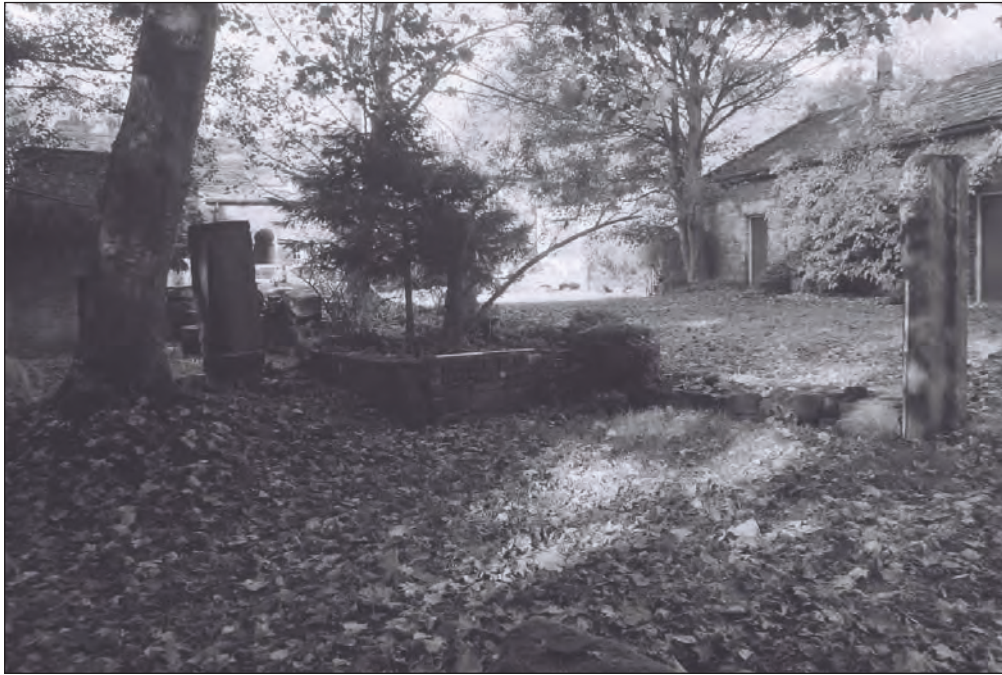
Plate 107: General 'internal' view of the eastern phase 4 range (Film 8.6)
