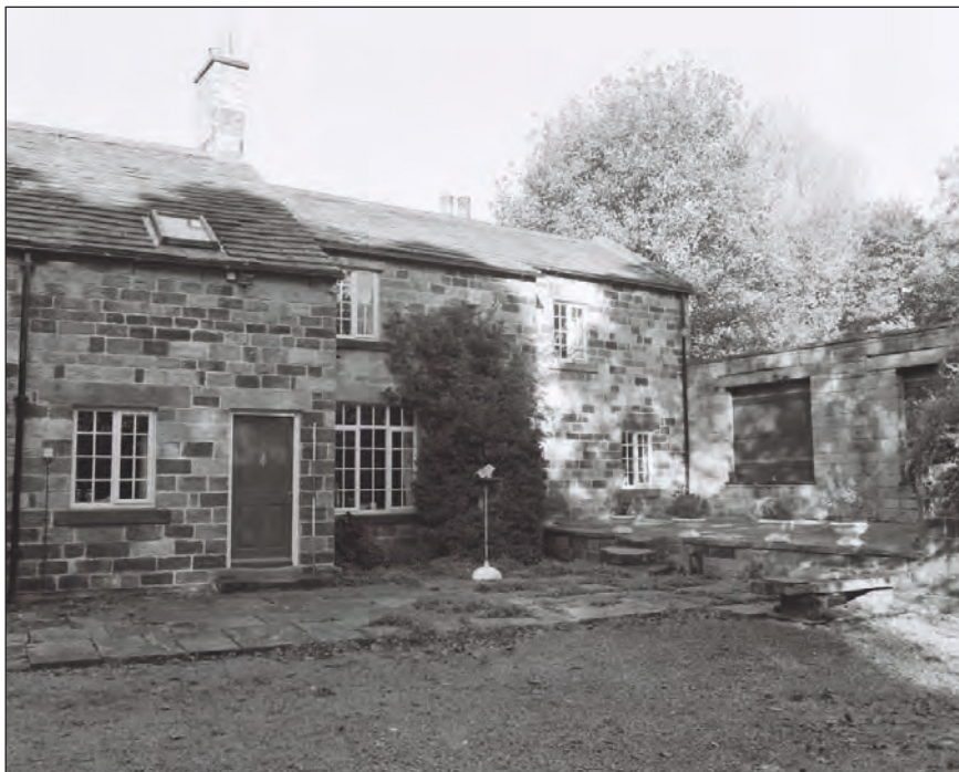
Plate 12: General view of the southeast elevation of the former Manager's House and remains of the former office (Film 3.4)
