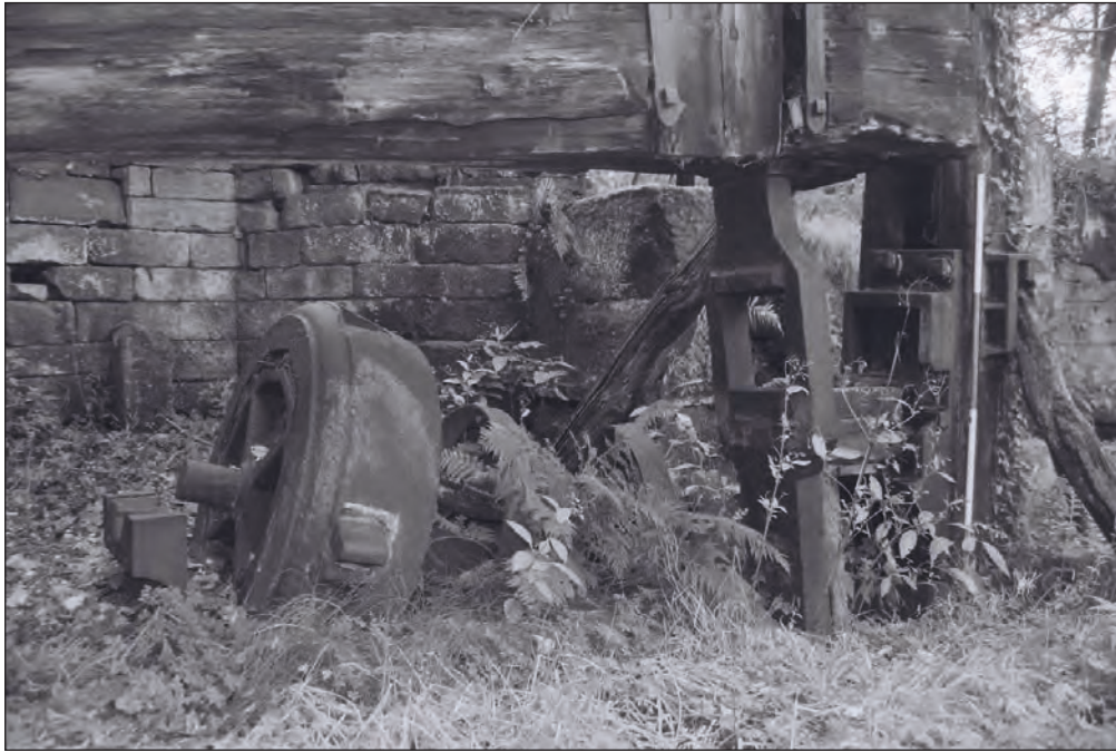
Plate 62: Detail of the west end mechanisms of the east helve hammer, south end of the central phase 1 former forge building (Film 9.6)
