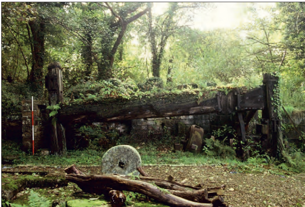
Plate 59: General view of the remaining east helve hammer, south end of the central phase 1 former forge building (Film CS. 21)
