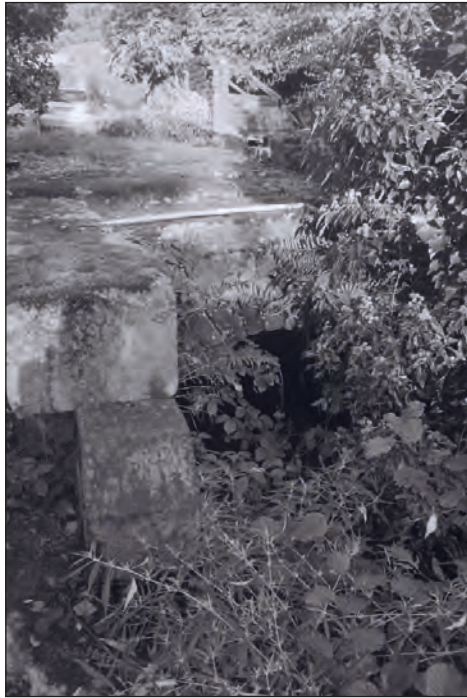
Plate 83: View of the wheel pit and tail race at the north end of the western phase 2 range (Film 10.6)
