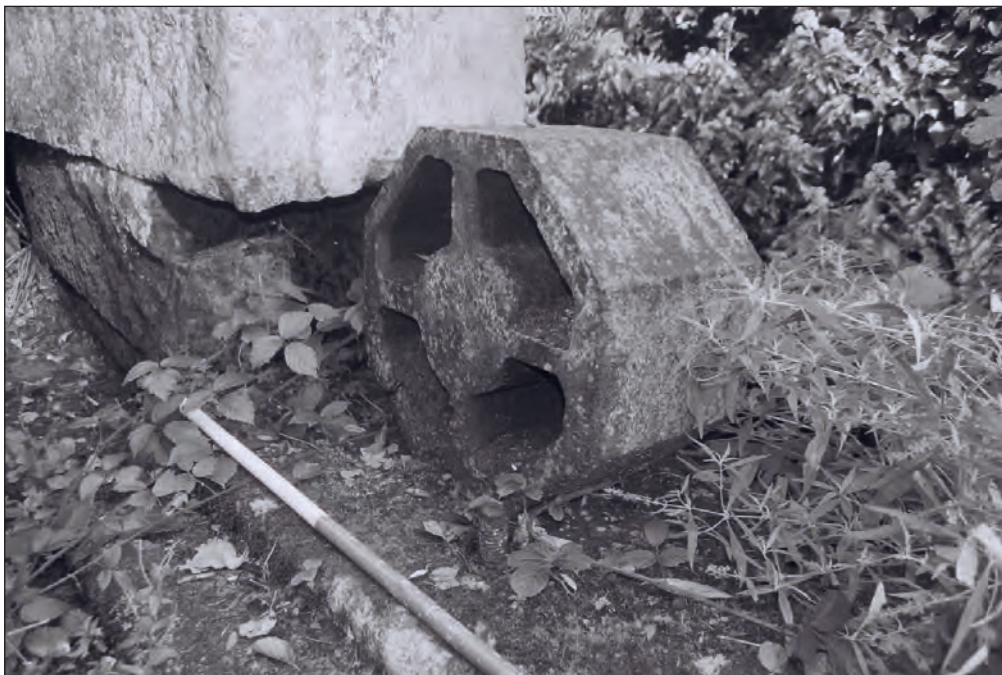
Plate 84: Detail of wheel mechanism remains at the north end of the western phase 2 range (Film 10.8)
