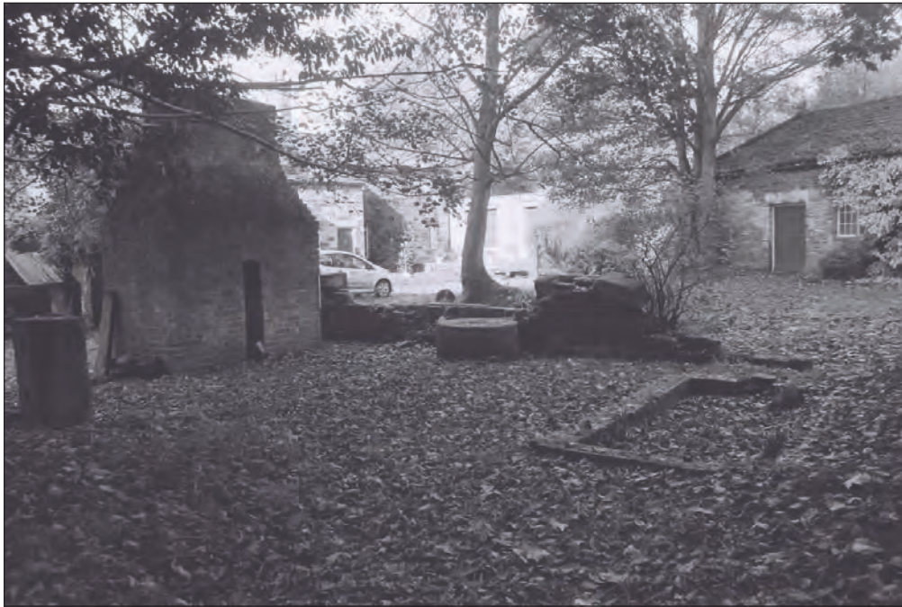
Plate 108: General 'internal' view of the eastern phase 3 range (Film 8.8)
