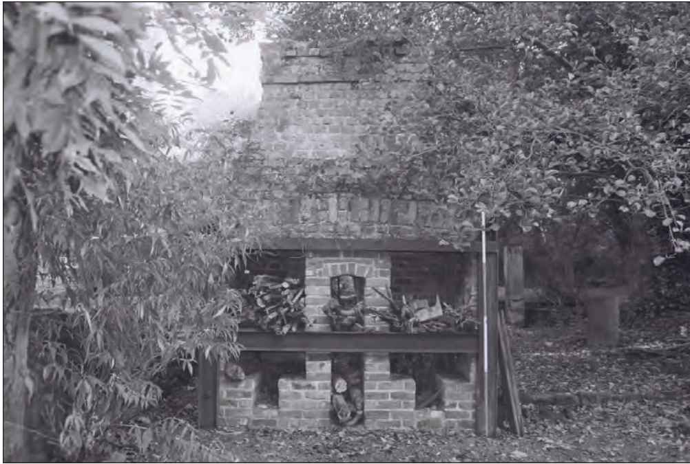
Plate 44: Detail of the remains of the eastern hearth within the central phase 1 former forge building (Film 8.22)
