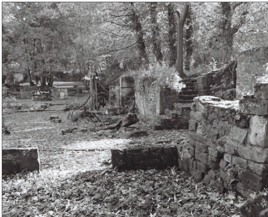
Plate 94: General view of the western phase 3 and 4 ranges (Film 6.3)
