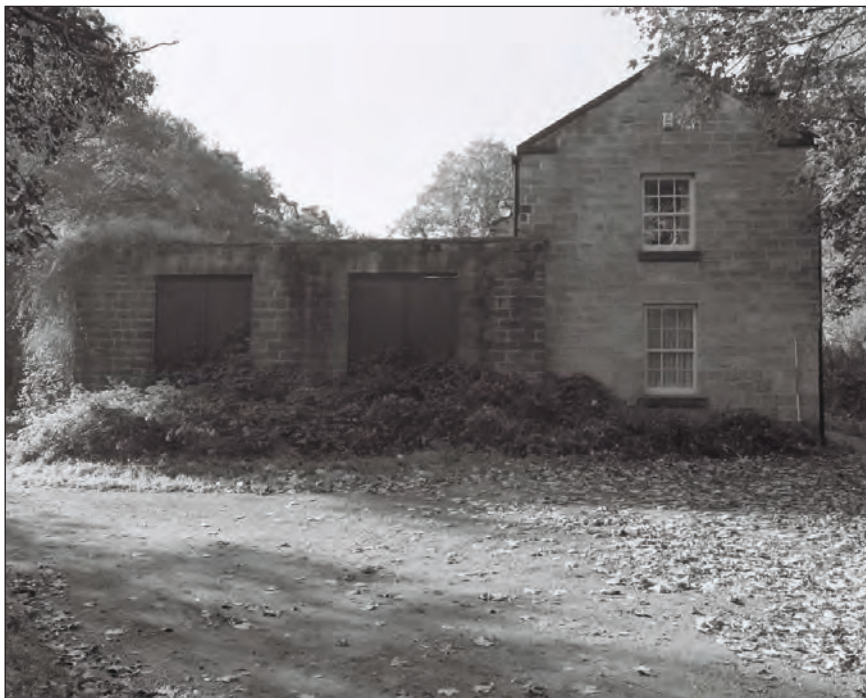
Plate 6: General view of the northeast elevation of the former Manager's House and office, Mousehole Forge from the 'Easy Going Trail' footpath (Film 2.7)
