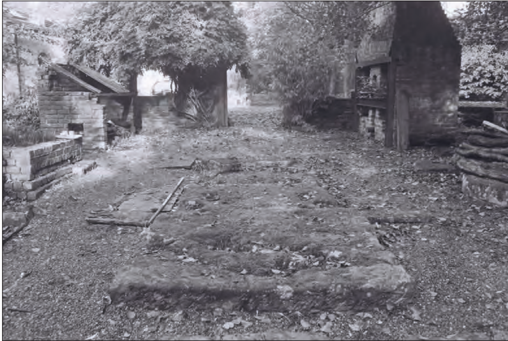
Plate 41: View of the former steam hammer base, looking northeast (Film 8.26)
