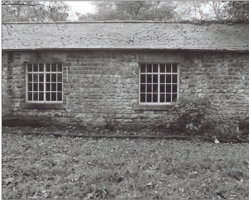
Plate 29: View of the south end of the southwest elevation of the former anvil store and workshop range (Film 1.6)
