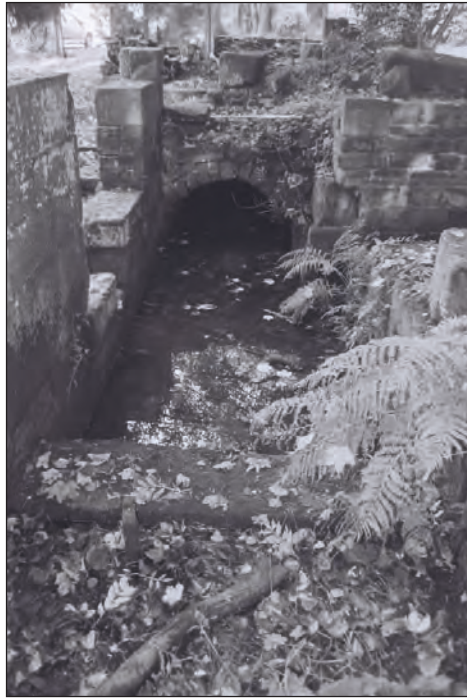
Plate 52: View of remains of wheel pit 4 adjacent to former grinding shop, south-eastern side of the central phase 1 former forge building, and tail goit (Film 9.8)
