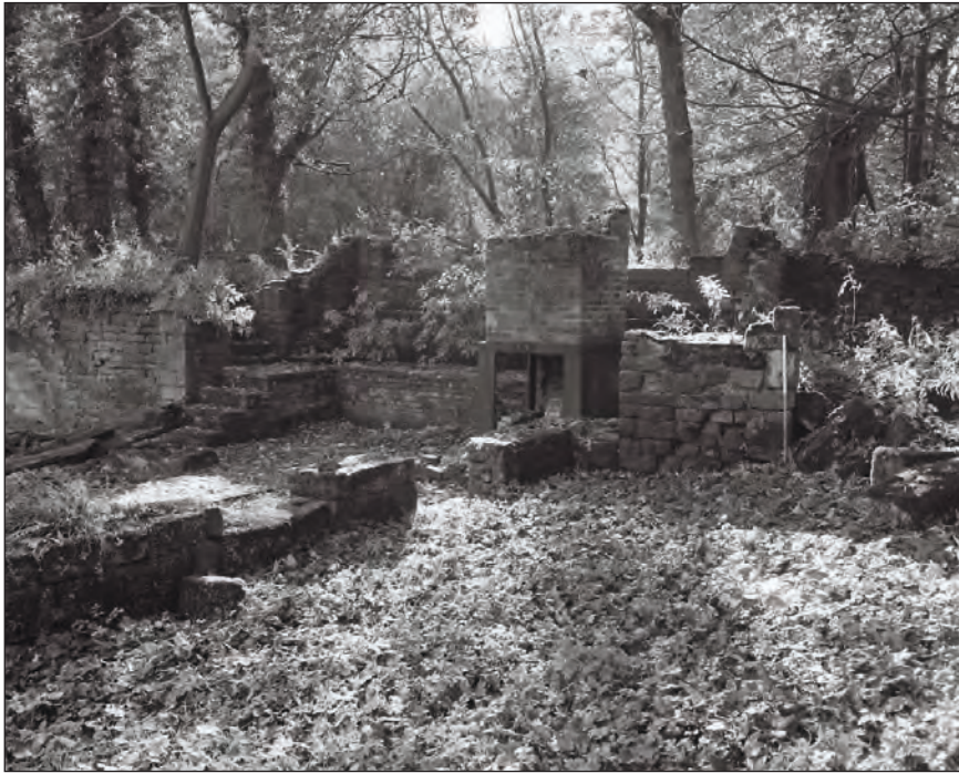
Plate 93: General view of the western phase 3 and 4 ranges (Film 6.1)
