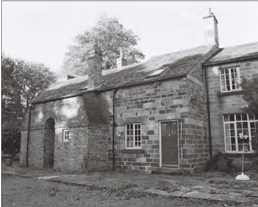
Plate 11: General view of the southeast elevation of the former Manager's House and attached furnace (Film 3.3)
