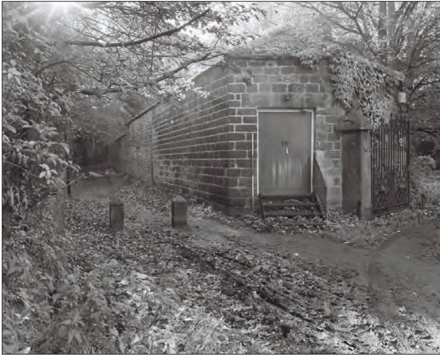
Plate 17: General view of the angled north corner of the Grade II listed former anvil store and workshop range (Film 2.6)
