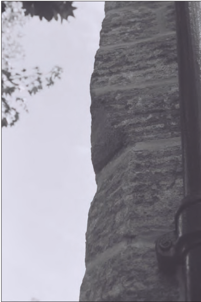
Plate 9: Detail of the chamfered and stopped north corner of the northeast and northwest elevation of the former Manager's House (Film 7.15)
