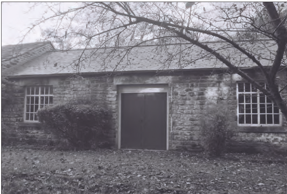
Plate 28: View of the south end of the southwest elevation of the former anvil store and workshop range (Film 7.29)
