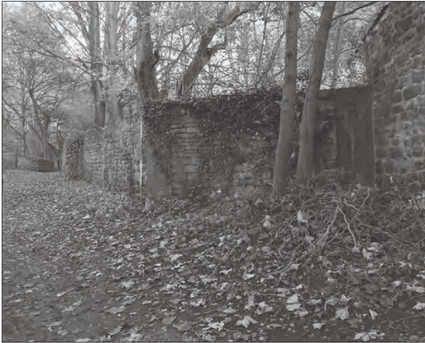
Plate 21: View of blocked entranceway within the eastern boundary (Film 2.3)
