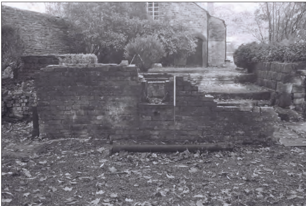
Plate 86: View of the south elevation of the puddling furnace at the north side of the western phase 2 range (Film 10.12)
