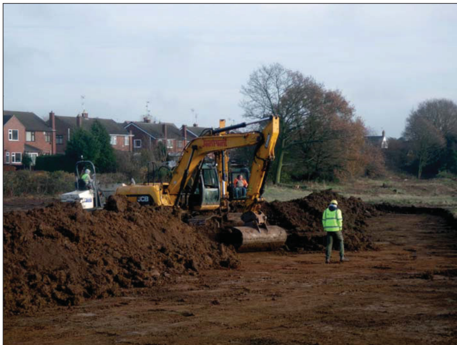
Plate 10: General shot of Area 2 during stripping
