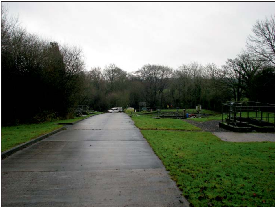
Plate 2: View facing east across sewage treatment works
