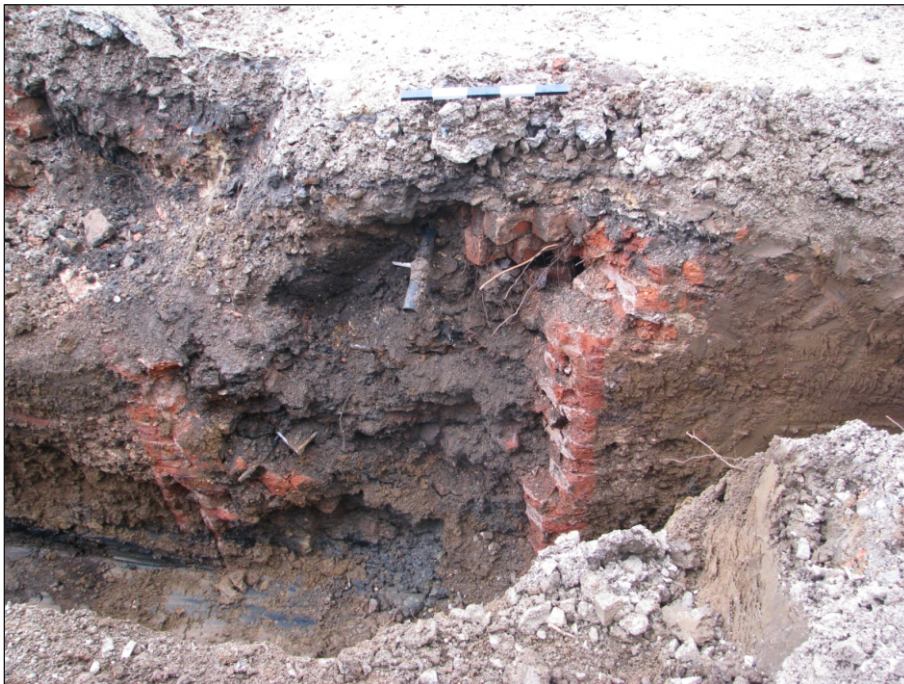
Plate 22: Modern redbrick manhole 903 in the northeast facing section of foundation trench, Plot 9
