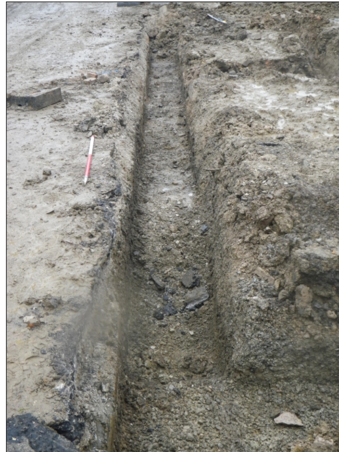
Plate 16: View of west foundation trench, in Plot 1, looking north
