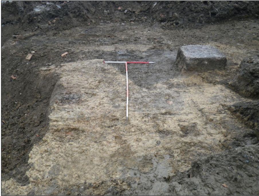
Plate 1: General view of Area 1 showing demolition cut 1003 , concrete stanchion base, cut of pit 1009 and the natural clay 1004 , looking west
