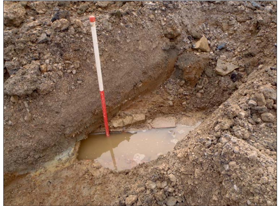
Plate 18: View of culvert 202 , Plot 6, looking southeast
