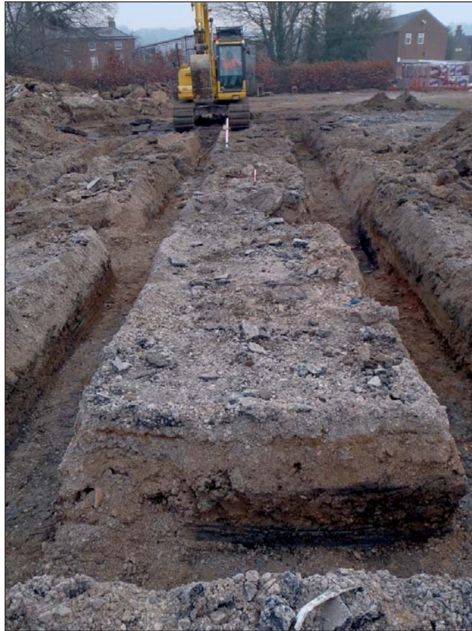
Plate 17: View of typical foundation trenches to Plot 6, looking east
