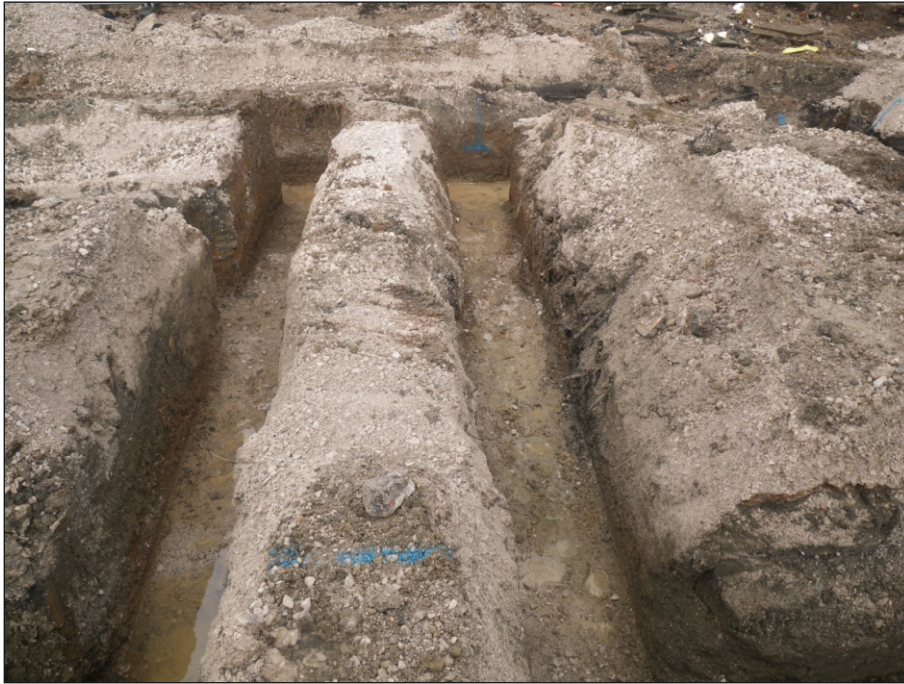
Plate 21: View of typical foundation trenches to Plots 7 and 8, looking north
