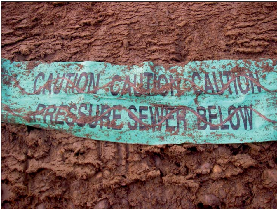
Plate 4: Pressure sewer warning tape
