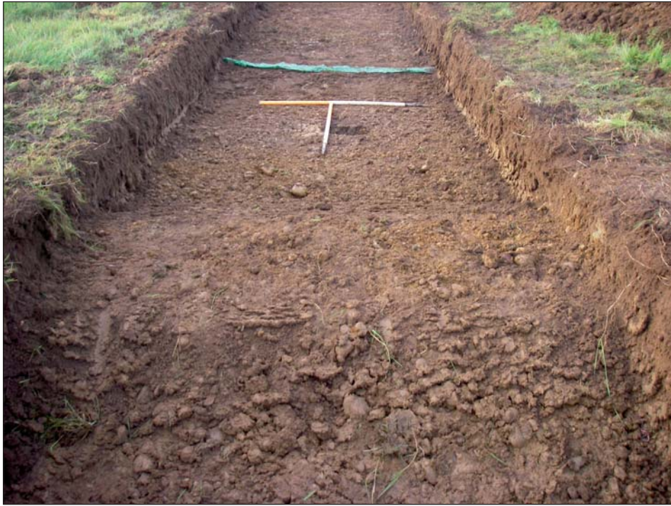
Plate 3: Pressure sewer cut with warning tape
