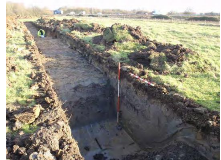
Plate 7: General view of canal, shows machine excavated test pit in foreground
