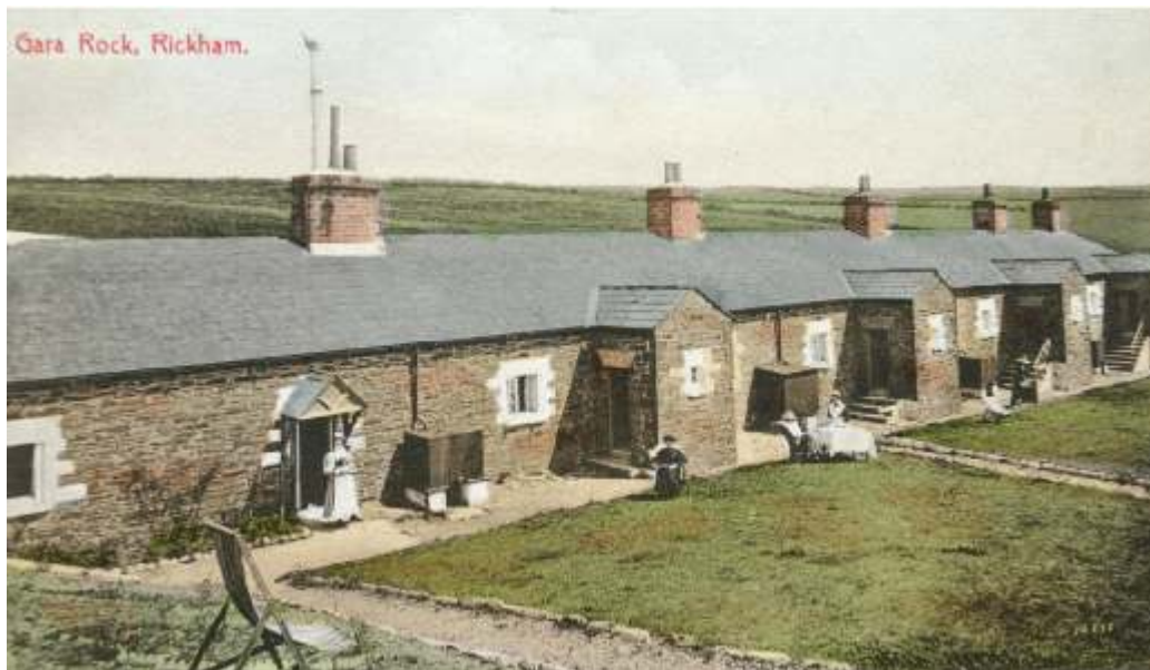
Plate 2. South facing range in 1909 just after the Jordans bought the property
