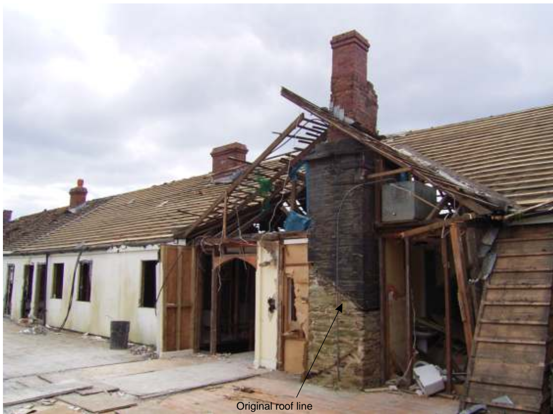
Plate 11. North-west chimney showing original roof line at first floor level
