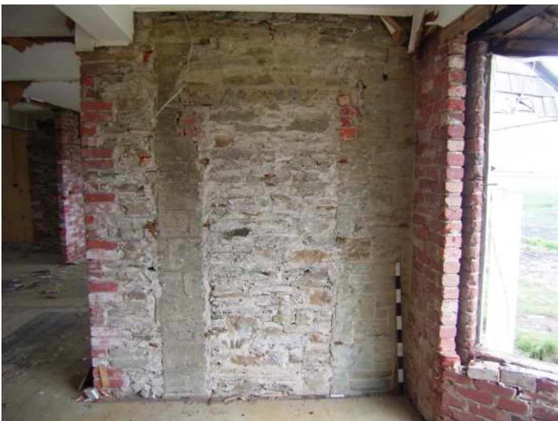
Plate 13. Surviving porch showing blocked original 19th century doorway
