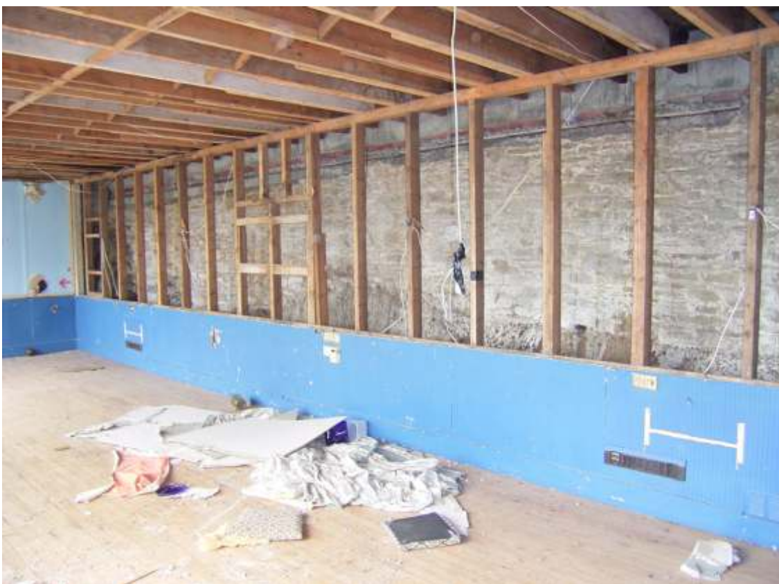
Plate 15. Store boundary wall; 'Great wall of Gara', behind panelling in breakfast room
