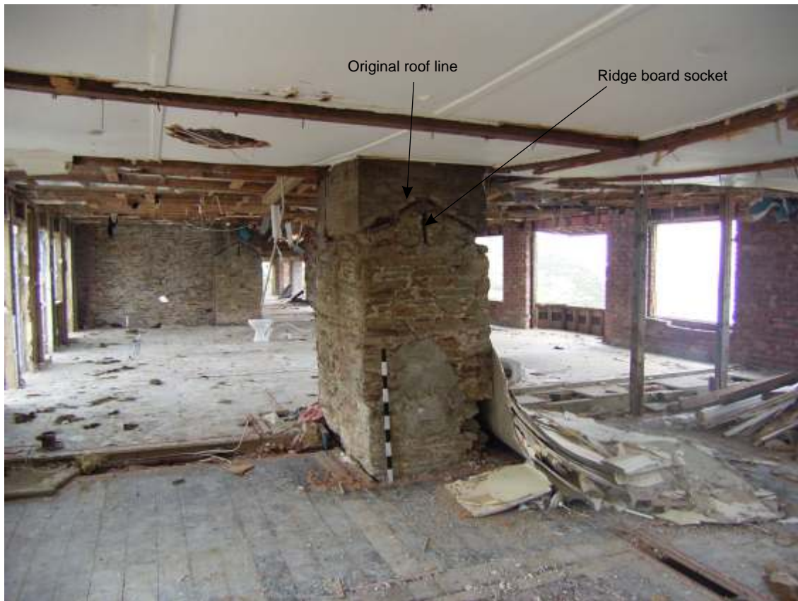
Plate 10. 19th century original chimneys and roof line within first floor space
