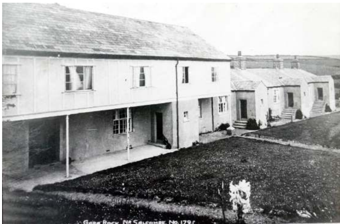
Plate 4. South facing range circa 1925 showing second storey
