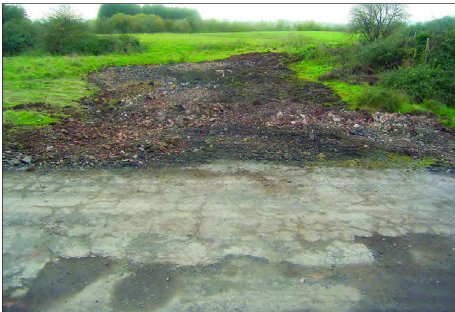
Plate 8: Surviving tarmac surface of perimeter road and hardcore base of fighter pen 90
