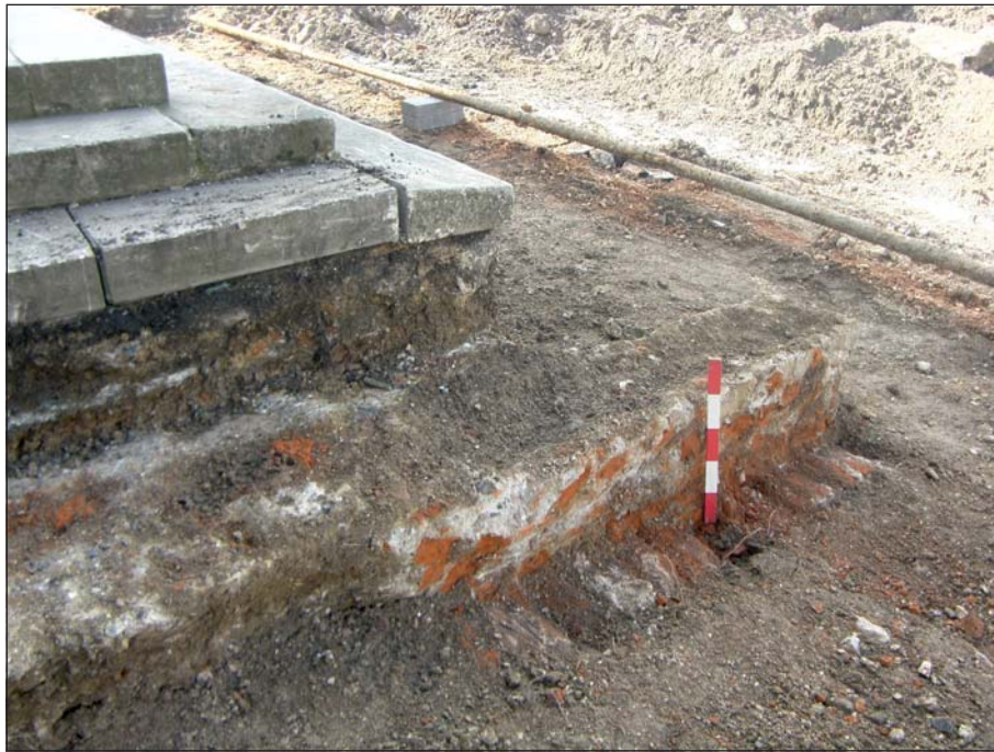
Plate 1: Wall 120, adjacent to Guildhall steps (view from south-east; scale = 0.5m)
