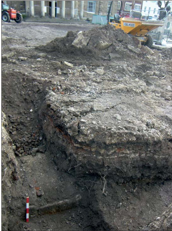
Plate 3: Structure 114, exposed in base of pipe trench (view from north; scale = 0.5m)
