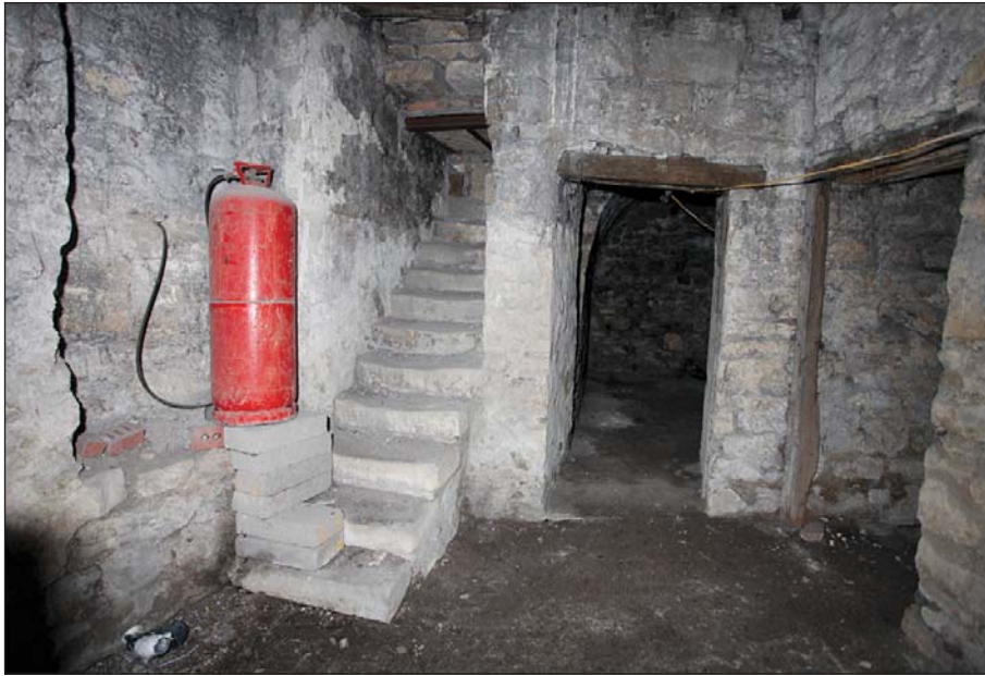
Plate 13: Sub-basement 10 Bridge Street. Truncated stone steps to basement.
