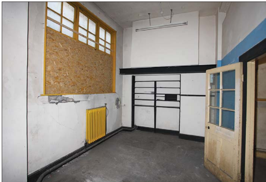
Plate 31: Basement SLe, south room
