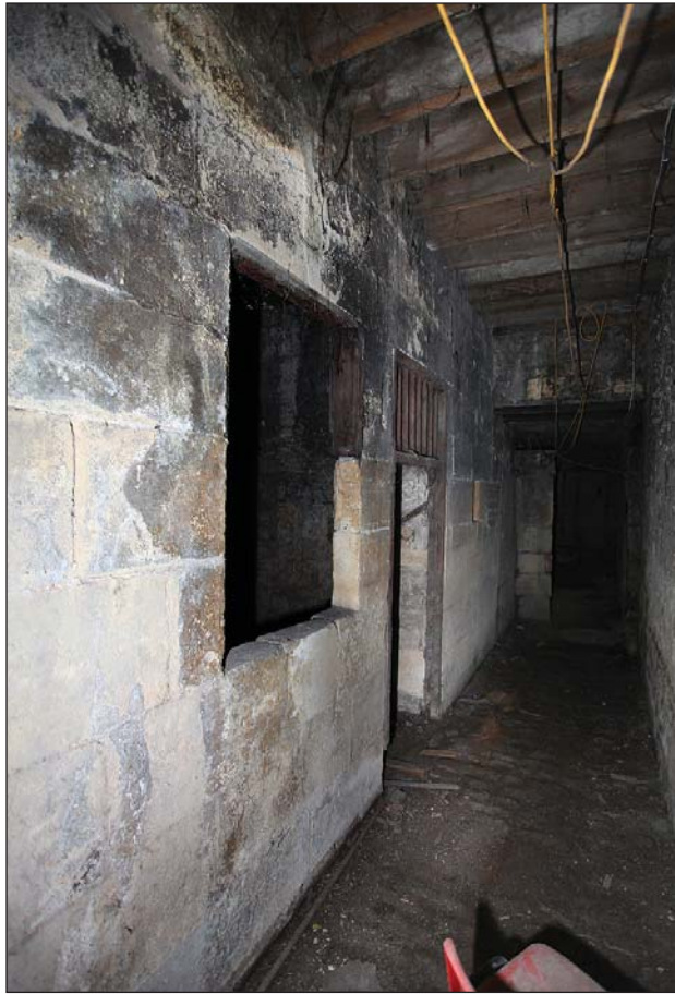
Plate 11: Sub-basement 10 Bridge Street. Early 20th century walling creating workshops.
