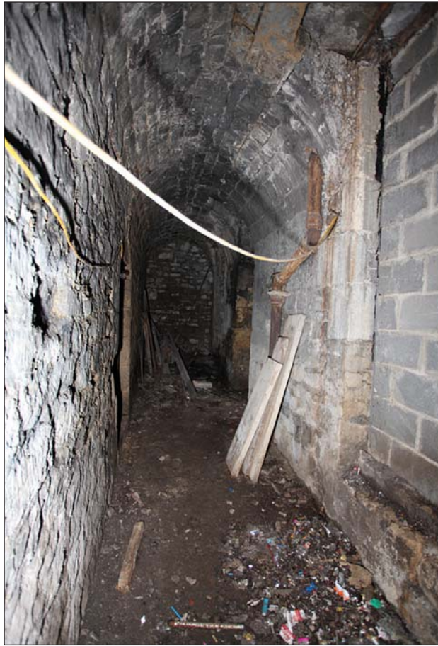
Plate 15: Sub-basement light wells and passage at east side of 9 Bridge Street
