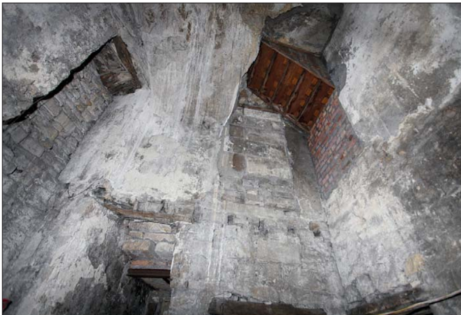
Plate 12: Sub-basement 10 Bridge Street. Inserted staircase visible in ceiling.
