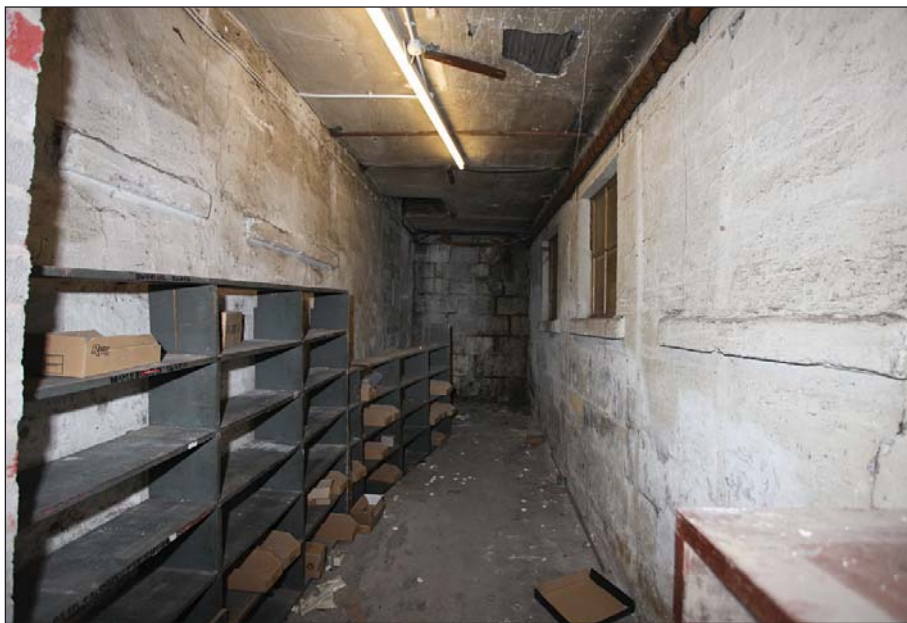
Plate 25: Basement NSd west-east passage, enclosed in early 20th century.
