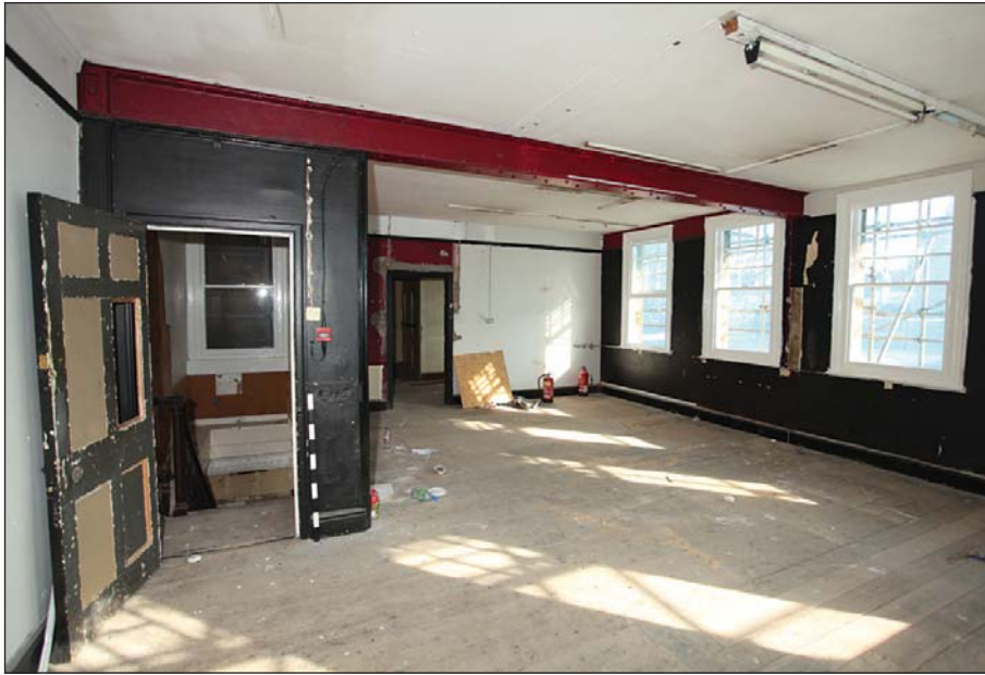
Plate 52: 1st floor 9 Bridge Street showing staircase to ground level
