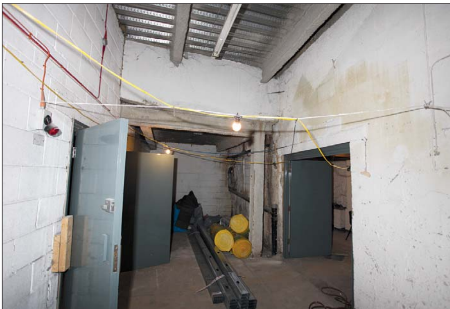
Plate 33: Basement 11 Bridge Street
