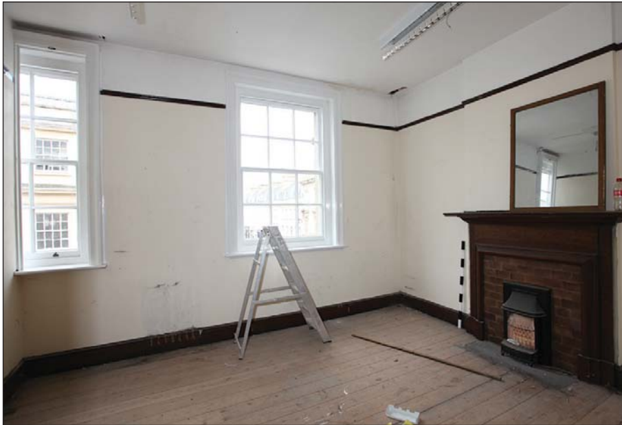
Plate 54: 2nd floor 12 Northgate Street west room with typical fixtures and fittings (circa 1928)
