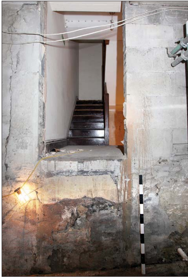
Plate 28: Basement SLa stairwell viewed from NSd passage
