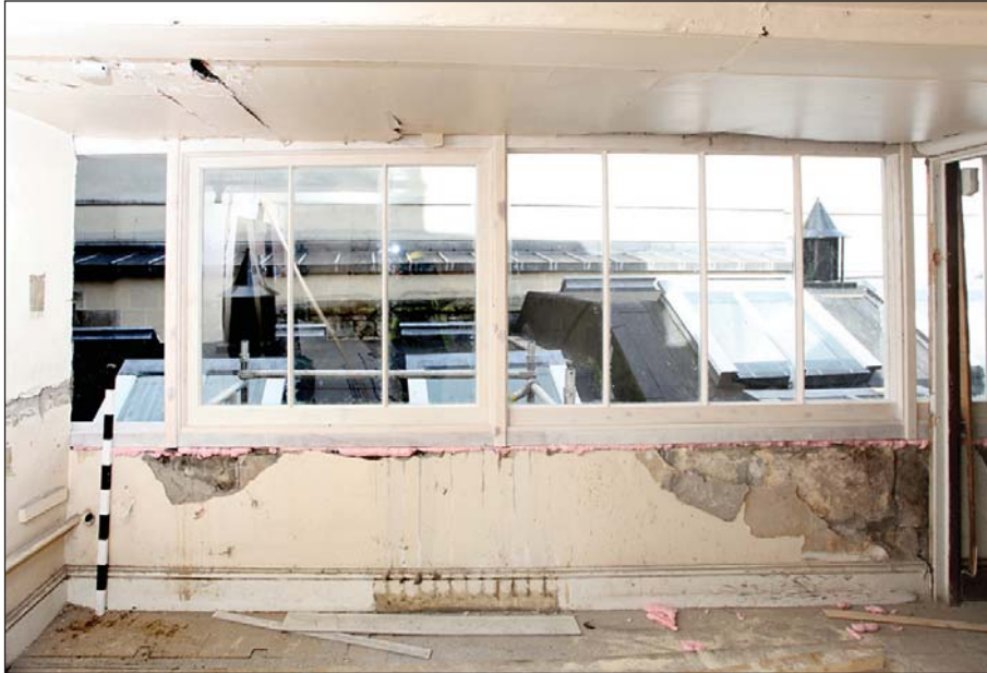
Plate 50: 1st floor SLa, east room windows
