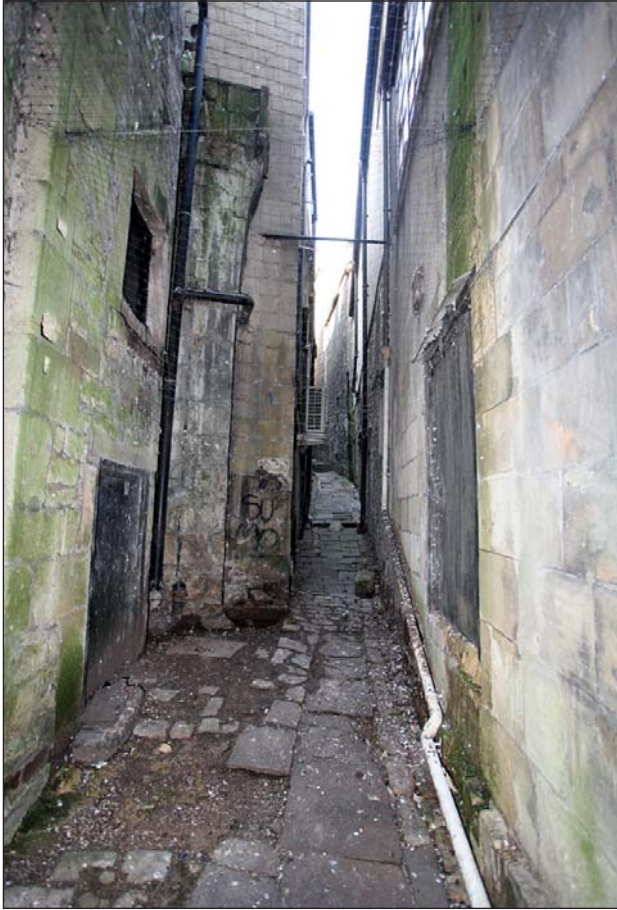
Plate 3: Remnant of medieval city wall preserved in-situ in south side of Slippery Lane
