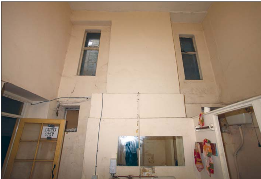
Plate 29: Basement SLa east room, south wall
