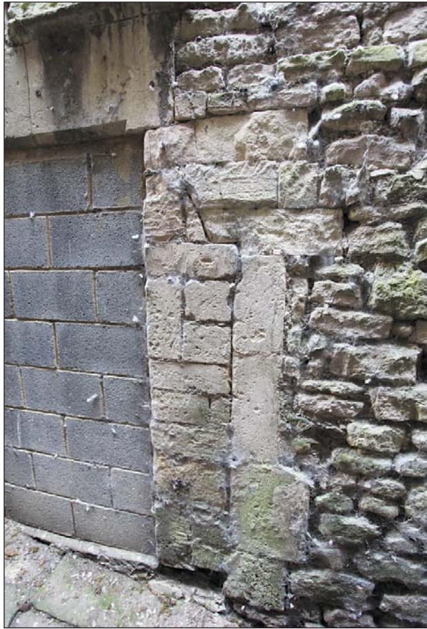
Plate 7: Evidence of earlier opening on east side of doorway, building SLd
