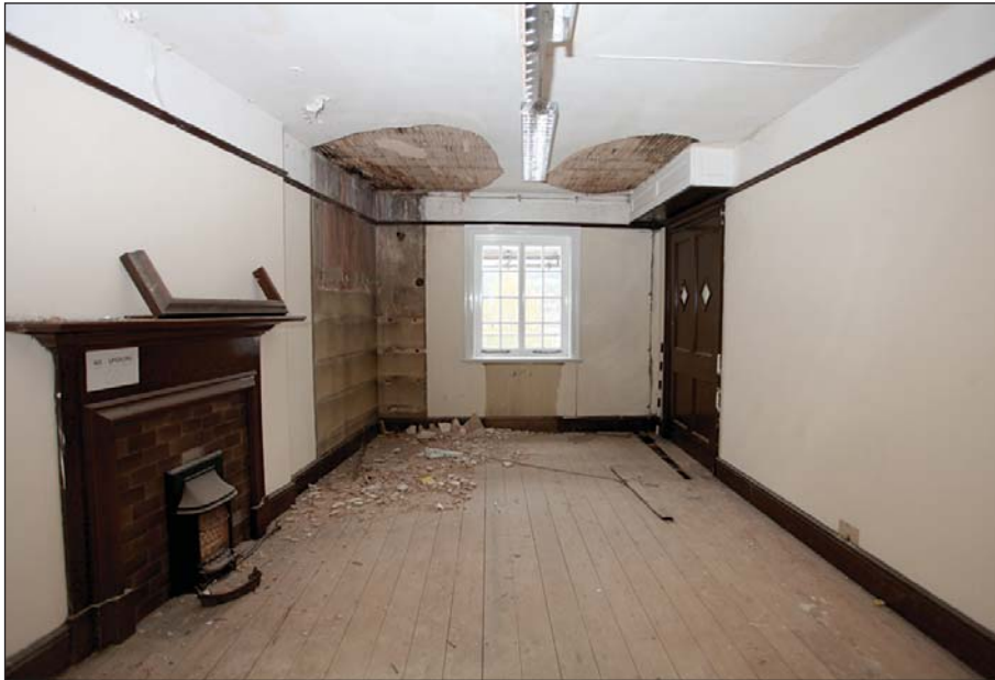
Plate 56: 3rd floor 12 Northgate Street east room
