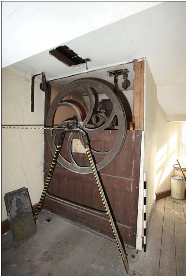
Plate 58: Lift mechanism to former lift shaft within 10 Bridge Street
