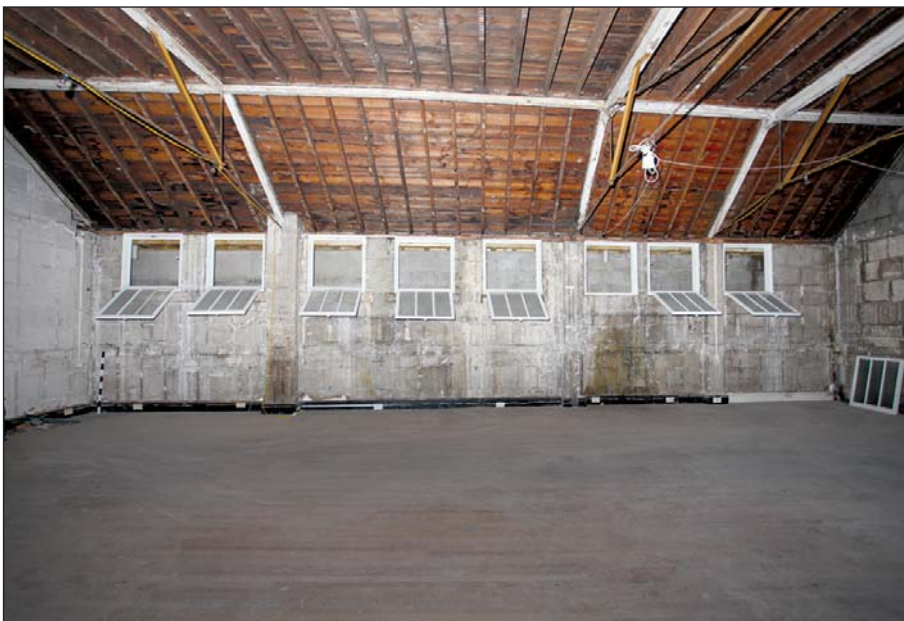
Plate 39: Ground floor, NSd-e north wall adjacent to the Podium Centre
