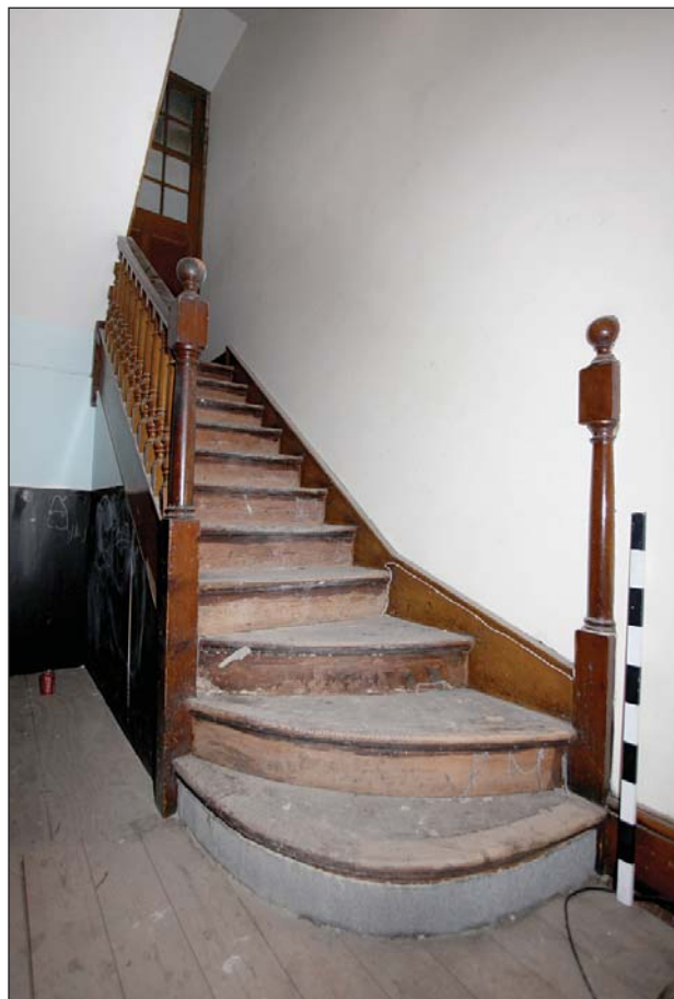
Plate 49: 12 Northgate Street stairwell at ground floor level
