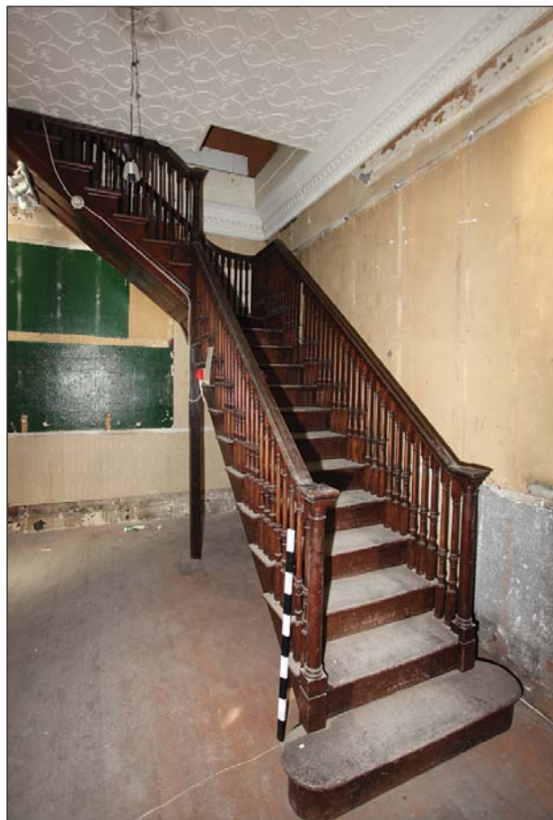
Plate 45: Detail of ground to 1st floor staircase in 9 Bridge Street
