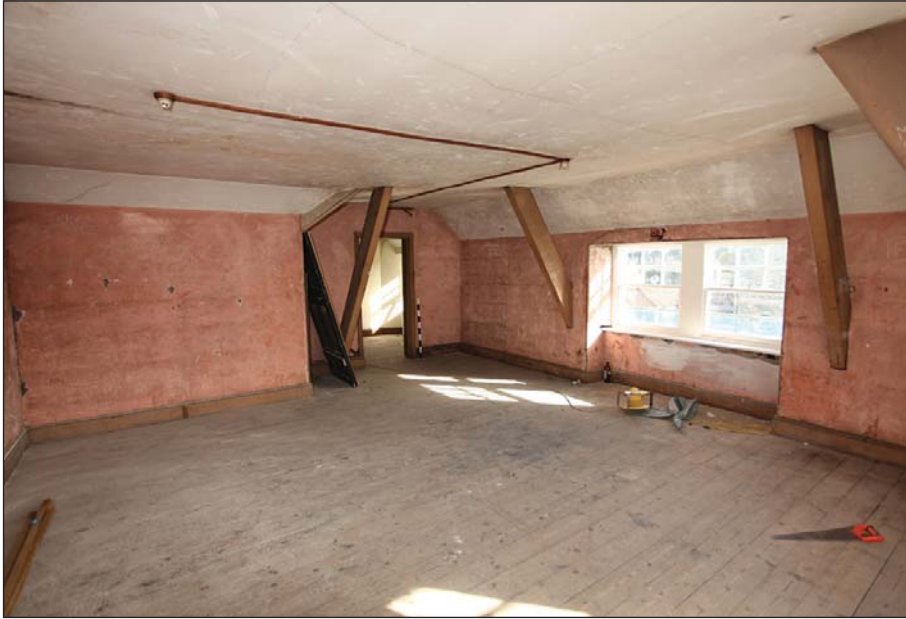
Plate 60: 3rd floor 9 Bridge Street
