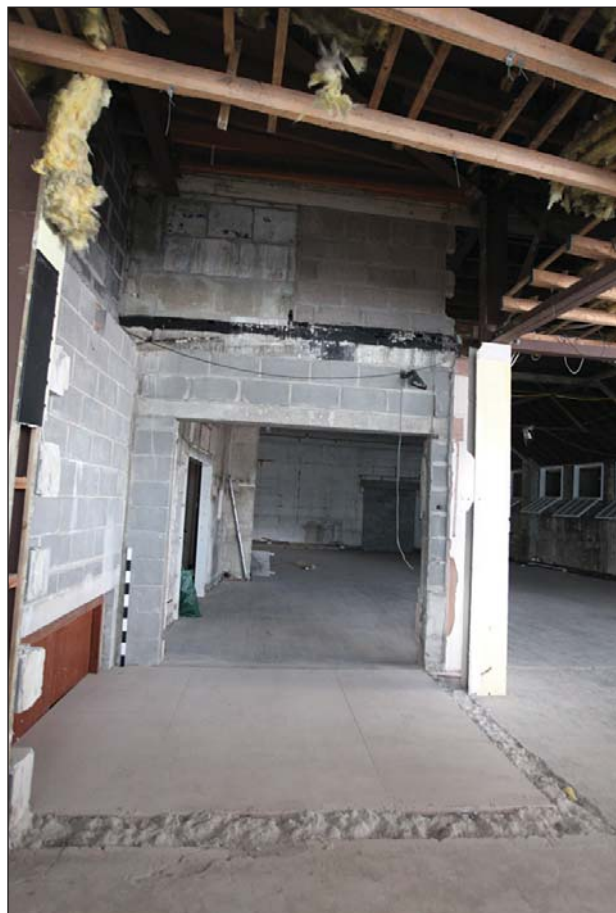
Plate 41: Ground floor east end of show rooms showing removed lift shaft
