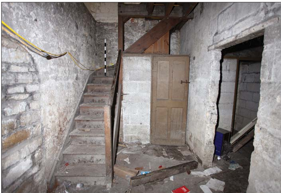
Plate 10: 9 Bridge Street stair access between sub-basement and basement
