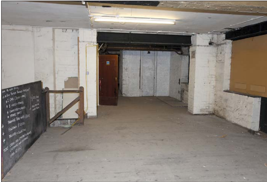
Plate 32: Basement 9-10 Bridge Street
