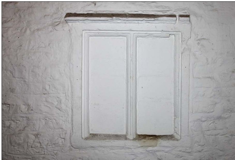
Plate 8: Detail of 17th century window frame north wall SLc
