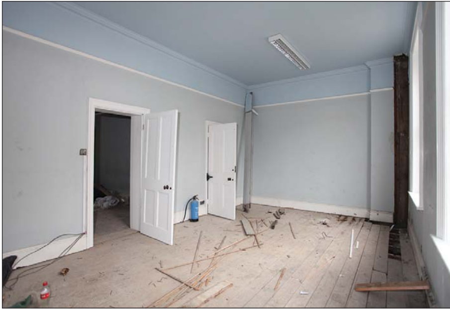
Plate 48: 1st floor 12 Northgate Street, west room
