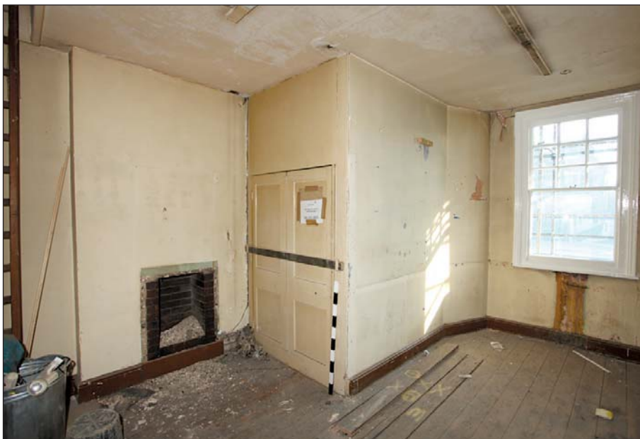
Plate 51: 1st floor 10 Bridge Street with former lift shaft
