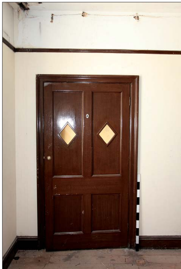
Plate 53: 2nd floor door to former lift shaft in 12 Northgate Street
