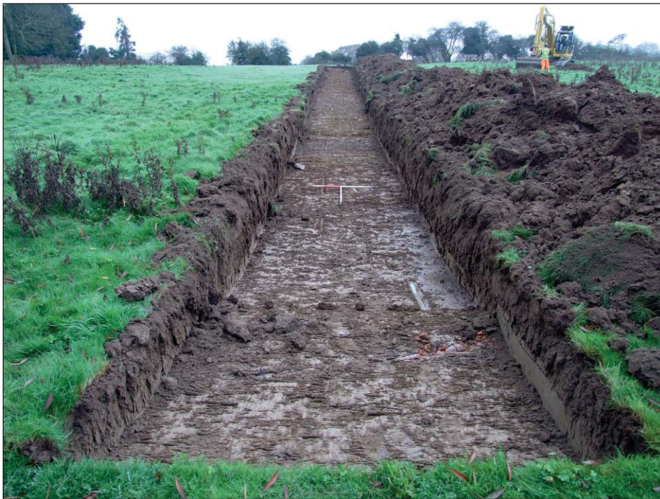
Plate 4: Trench 4, general shot, facing south
