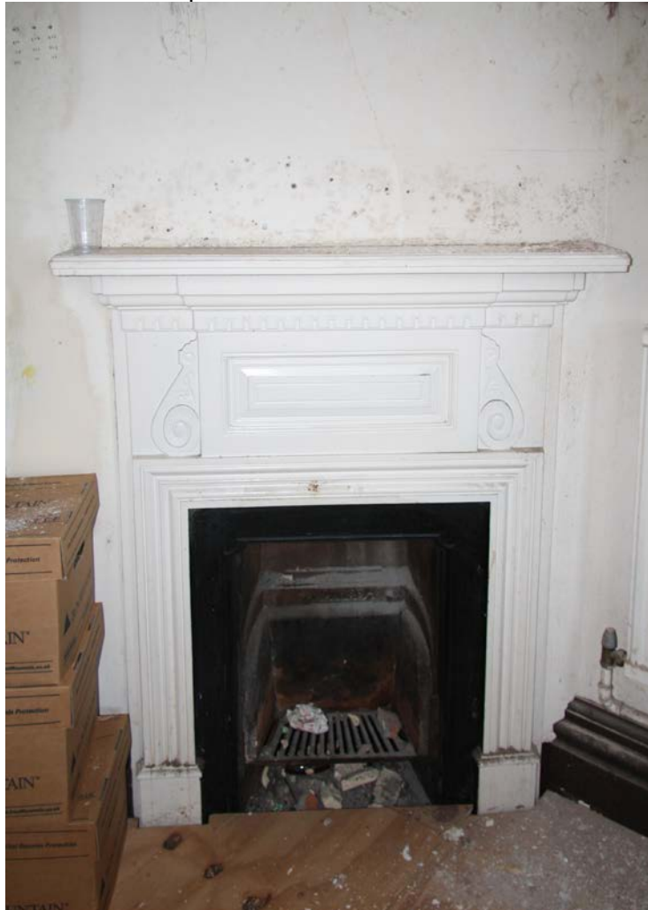
Plate 8: Fireplace at west end of the second floor
