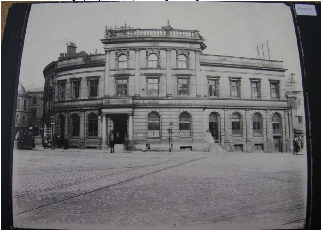
Plate 1: Undated photograph (pre-1935) showing the original Oldham Joint Stock Bank façade
