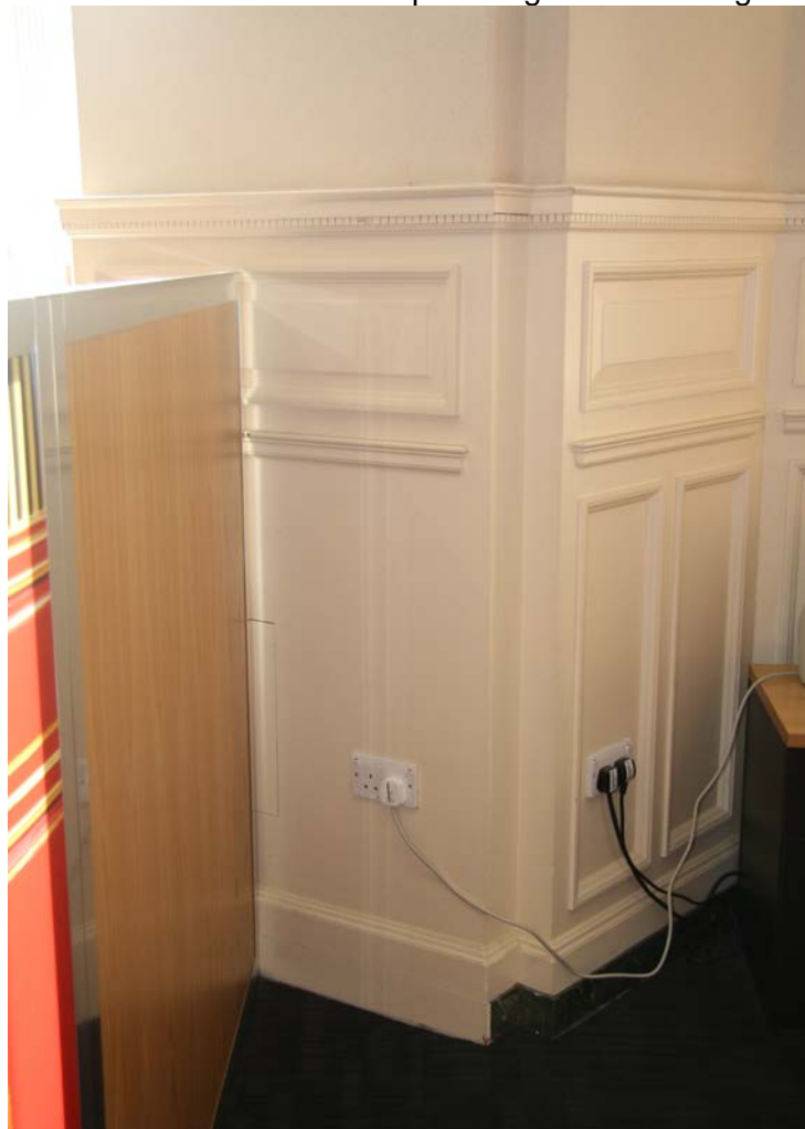
Plate 6: Ground floor dado panelling in the banking hall
