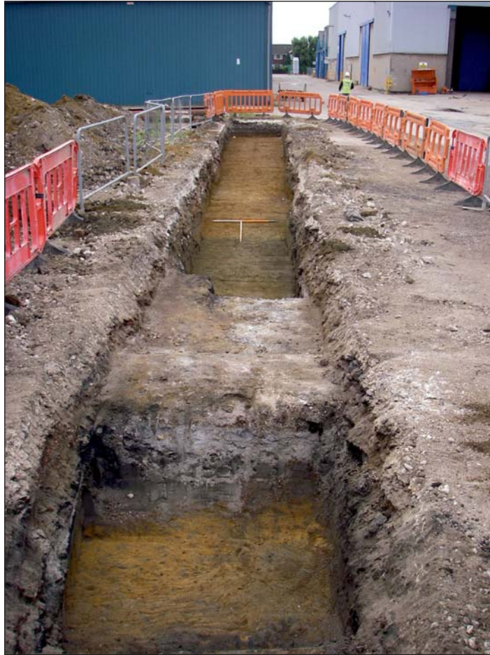
Plate 7: General view of Trench 3 looking southeast
