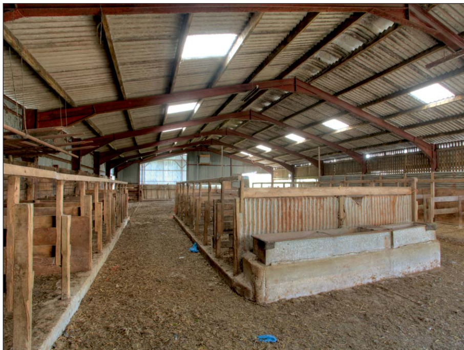
Plate 4: North-south orientated barn interior
