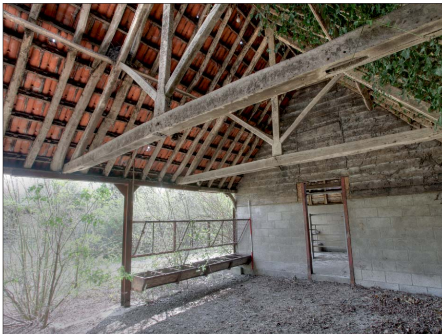
Plate 26: Eastern study building, west end: east room
