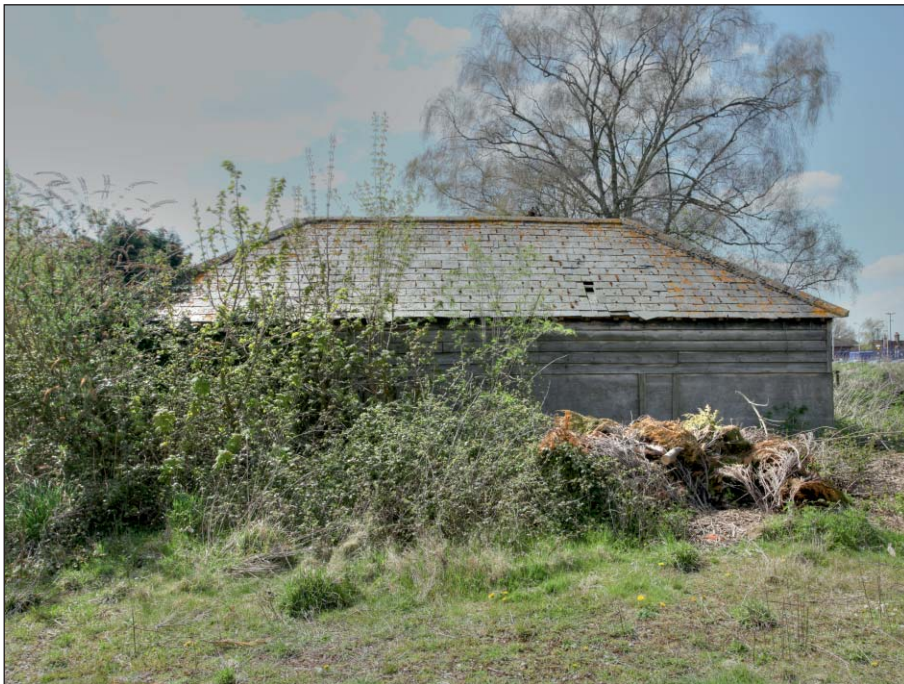
Plate 18: Eastern study building, east end: east elevation
