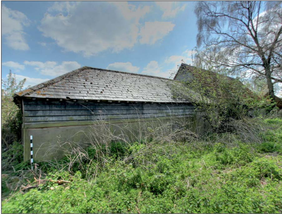
Plate 17: Eastern study building, east end: north elevation
