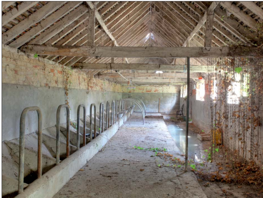
Plate 15: Western study building: interior
