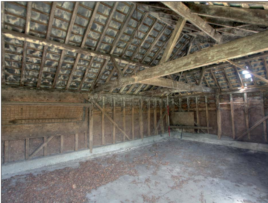
Plate 20: Eastern study building, east end: north-east corner
