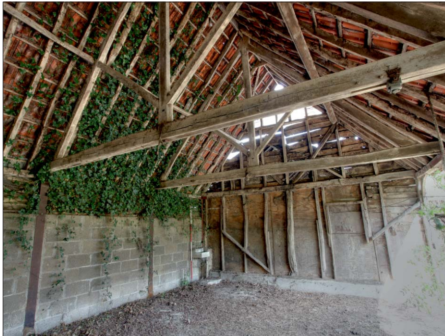
Plate 25: Eastern study building, west end: east room
