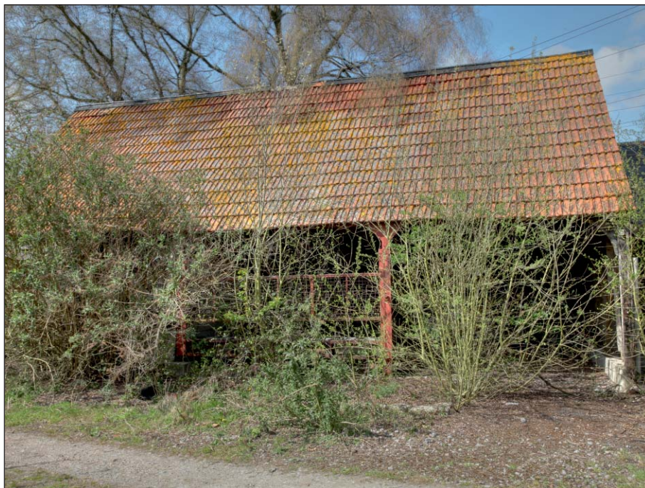
Plate 22: Eastern study building, west end: south elevation
