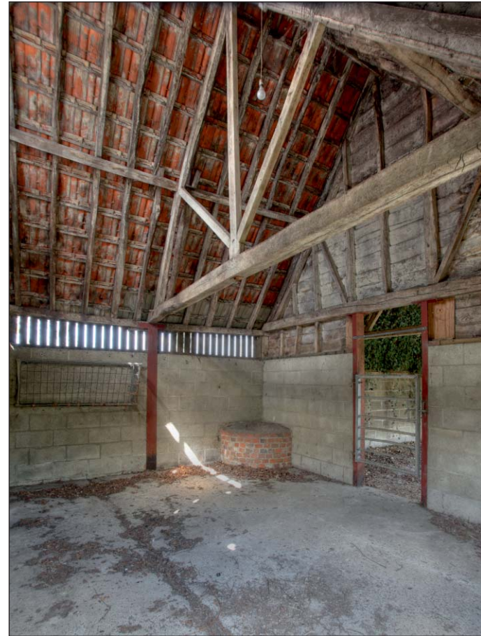
Plate 24: Eastern study building, west end: west room
