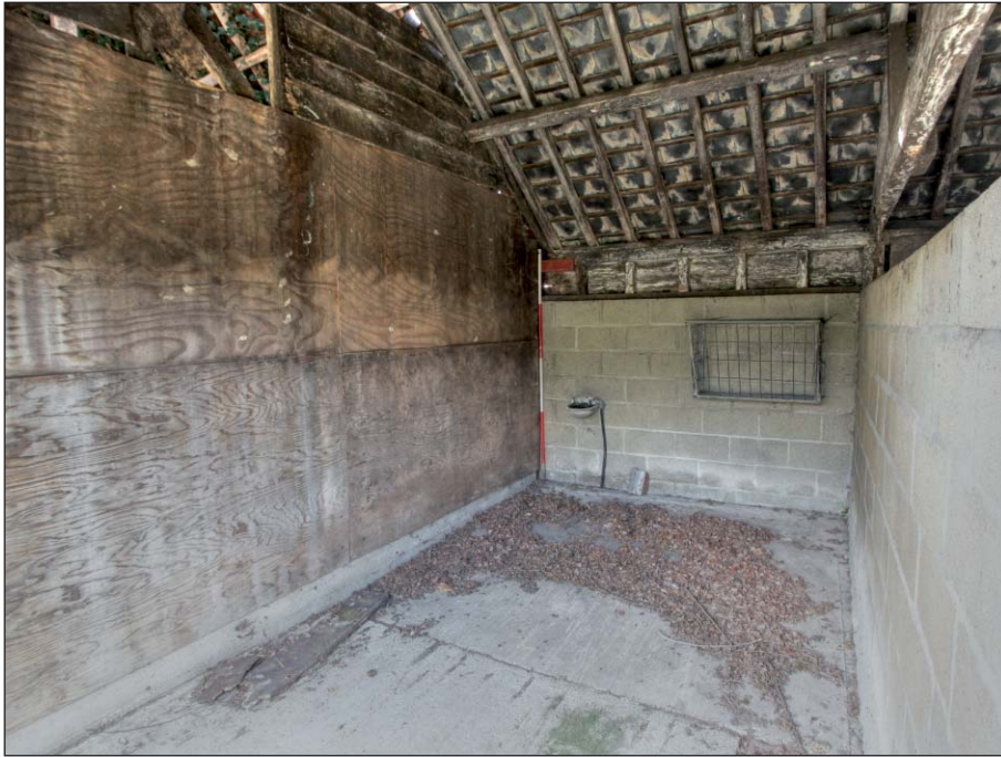
Plate 19: Eastern study building, east end: typical interior space
